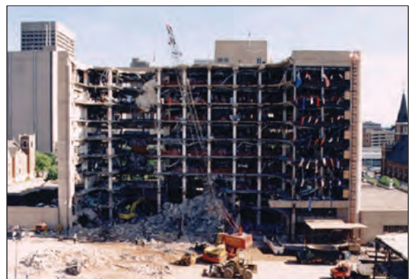
Figure 1-6: Aftermath of the Murrah Federal Building bombing
