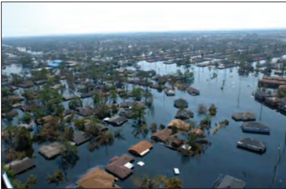
Figure 1-7: Flooding caused by Hurricane Katrina
