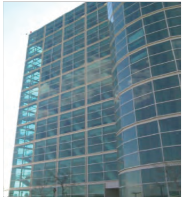
Figure 4-9. Building enclosure with a curtain glass wall
