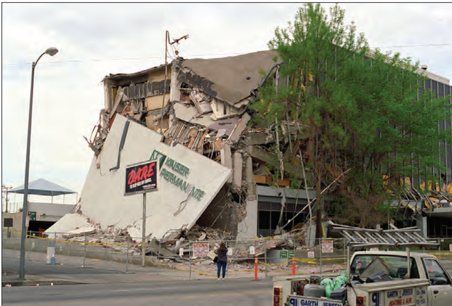
Figure 1-5: Building damaged by the Northridge Earthquake
