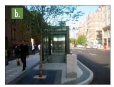
b. Barrier designed to protect the station entrance from an accidental vehicular impact, but an intentional strike is still possible
