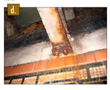
d. Severe corrosion of this steel beam and bearing in the station demonstrates a major flaw that could cause problems
