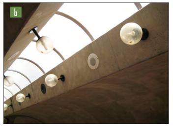
b. Example of fixture attachments that are not secure
