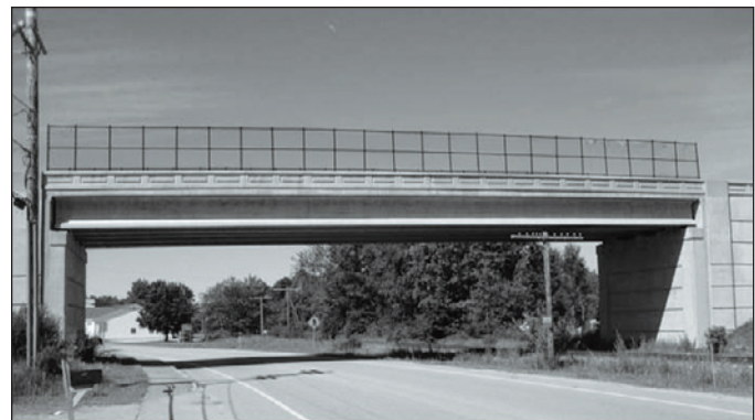
Figure 3-30: New Rollins Road Bridge, opened in 2000
