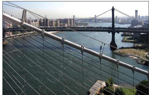
Figure 3-5. Brooklyn, Manhattan and Williamsburg bridges
