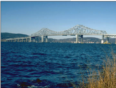
Tappan Zee Bridge
