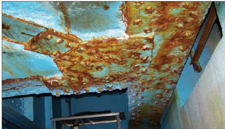
Figure 3-3: Corrosion of a steel member.
