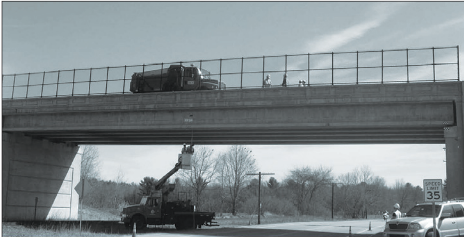
Figure 3-33: Photo of load test while survey crew takes displacement reading
