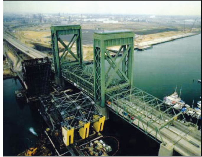
Figure 3-48. Schuyler Heim Lift Bridge Long Beach, CA
