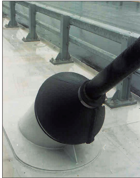
(b) Stay cable of the Tatara Bridge
