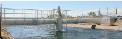
(c) Hydrokinetic canal application<sup>2</sup>
