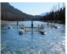
(b) Hydrokinetic free-flowing river application<sup>2</sup>
