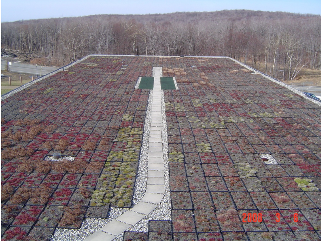
Figure 6. Green Roof on Industrial Building (Source: USACE, Baltimore District)
