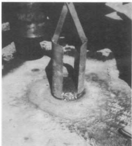
Figure 3. Removing a pavement core
