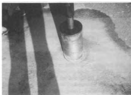
Figure 2. Close-up of pavement drill
