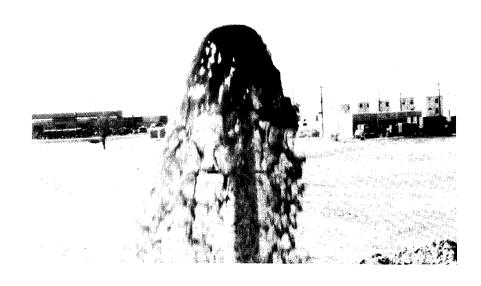
Figure 5. Discolored water as a result of pigging.
