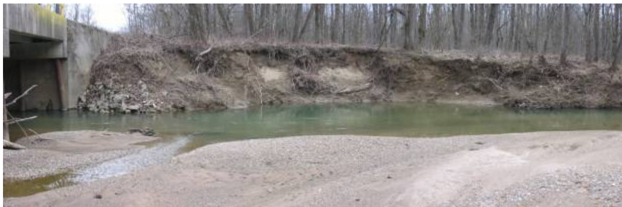
Figure C3. Demonstration site preconstruction, downstream side, northeast corner.
