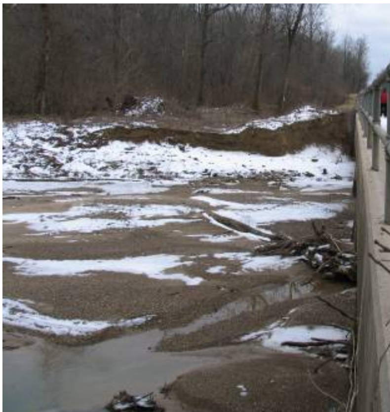
Figure C8. Demonstration site preconstruction, upstream side, northwest corner.
