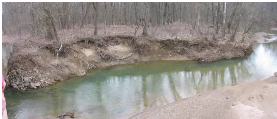
Figure C2. Demonstration site preconstruction, downstream side, northeast corner.
