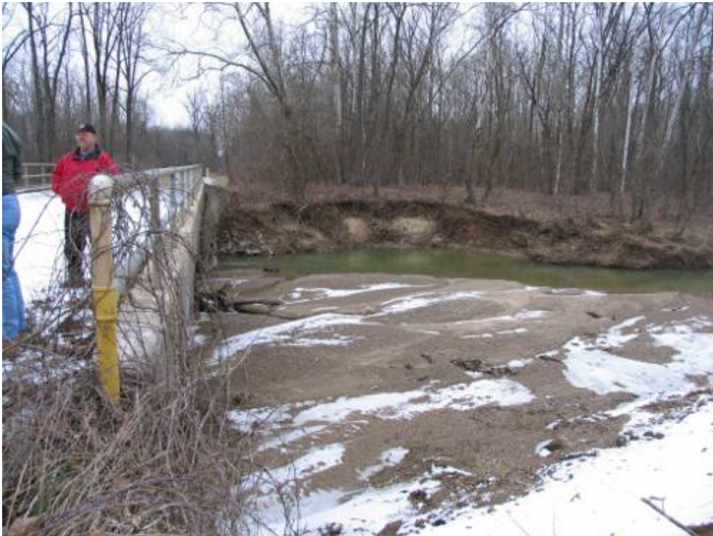
Figure C6. Demonstration site preconstruction, downstream side, northeast corner.
