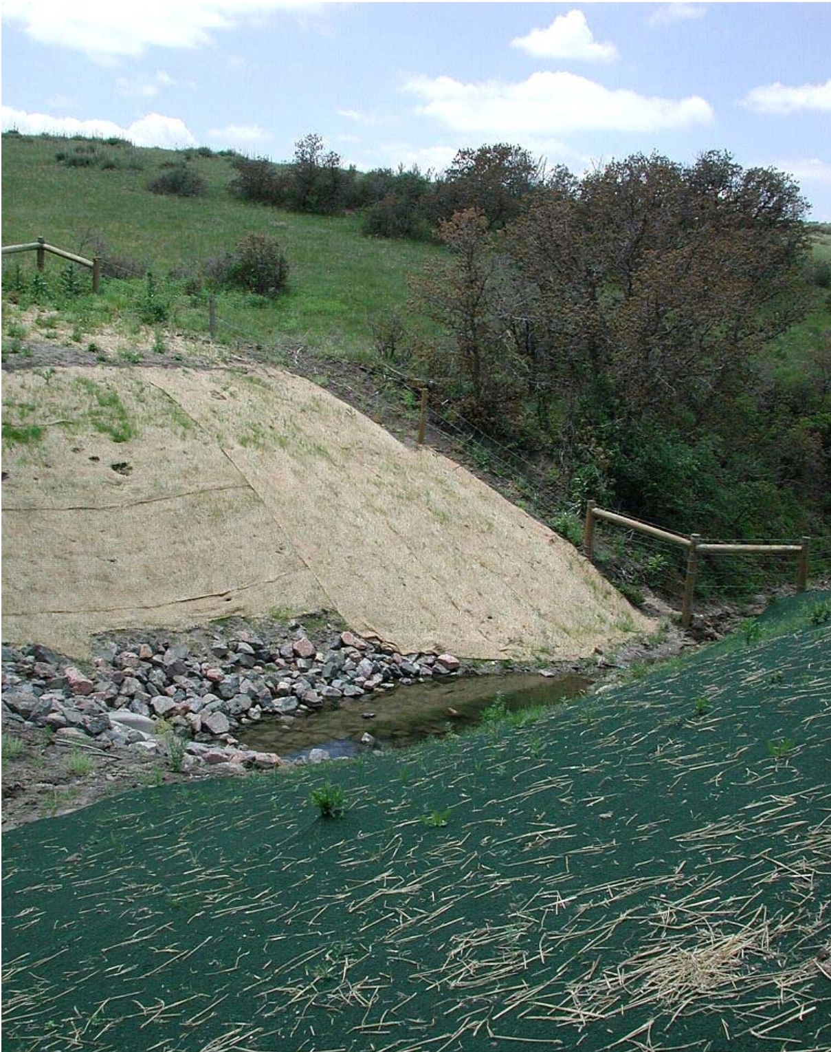
Figure B11. Demonstration of two different blankets, biodegradable jute and synthetic polymer.
