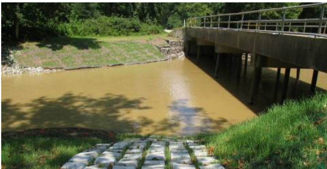
Figure C18. Demonstration site 1 month post-construction; looking at northwest corner.
