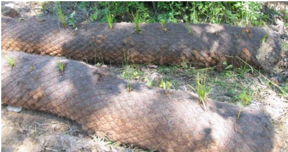
Figure B7. Vegetated biologs.
