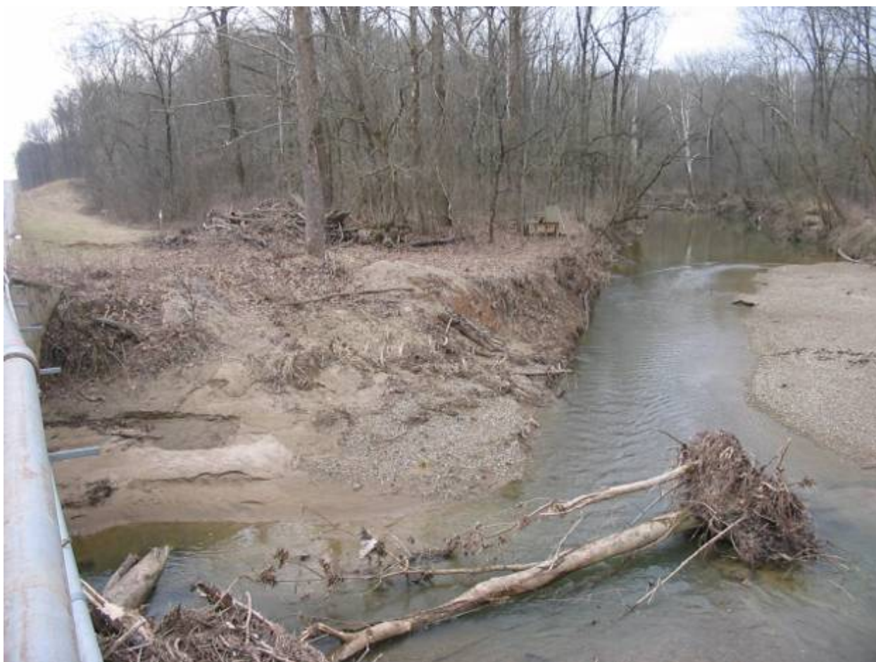
Figure C4. Demonstration site preconstruction, upstream side, southwest corner.
