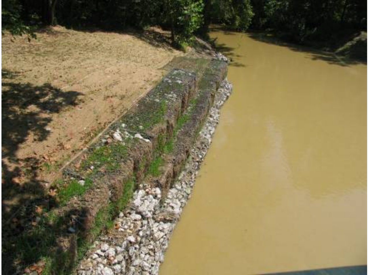
Figure C19. Demonstration site 1 month post-construction; view from bridge downstream at northeast corner.
