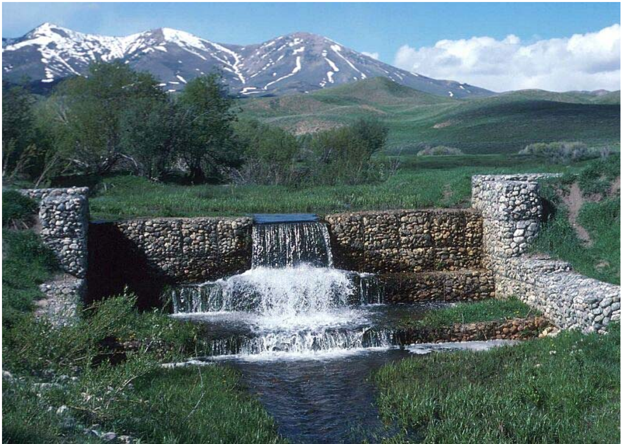
Figure B12. Gabions were used to develop this drop structure (source: USDA).
