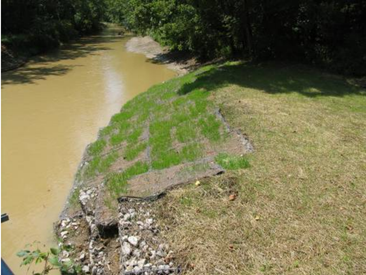
Figure C17. Demonstration site 1 month post-construction; upstream northwest corner.
