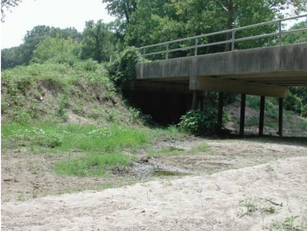
Figure C5. Demonstration site preconstruction, downstream side, southeast corner.
