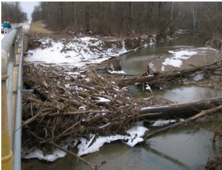
Figure C7. Demonstration site preconstruction, upstream side, southwest corner.
