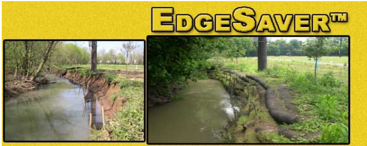
Figure B9. Compost filled sock system helps increase infiltration while providing channel stability (source: Filtrex).
