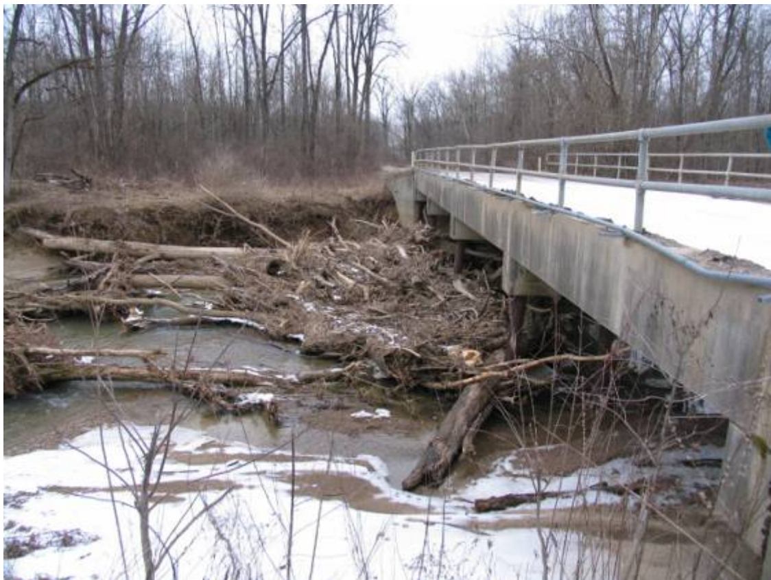
Figure C1. Demonstration site preconstruction, upstream side, northwest corner.
