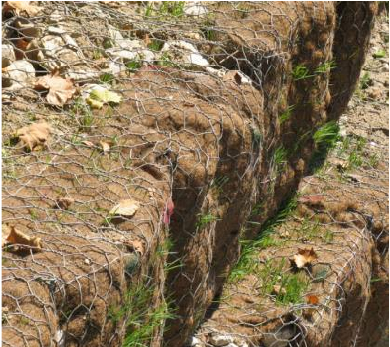
Figure B13. Gabions incorporating soil, erosion control blanket and seed.
