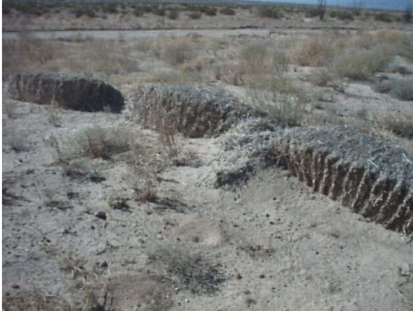
Figure C12. Close-up of bales shows that little degradation has occurred over the years, but sediment has accumulated at the base of the bales (Morrill, YPG).
