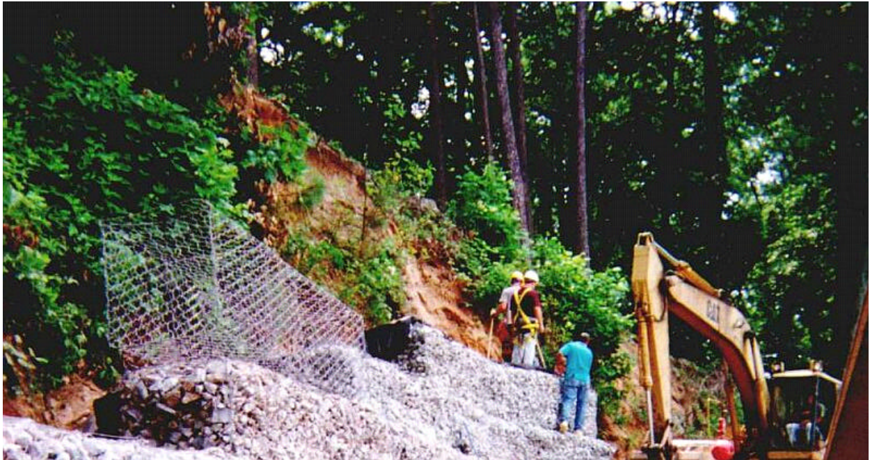
Figure B32. Installment of gabions to stabilize firing range backstop.
