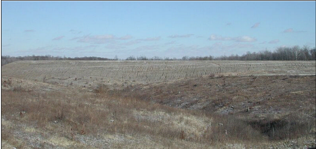
Figure C7. MPTR berm constructed entirely out of GeoWeb ® . Due to difficulties establishing vegetation, excessive rill and sheet erosion has occurred along the face of the berm.
