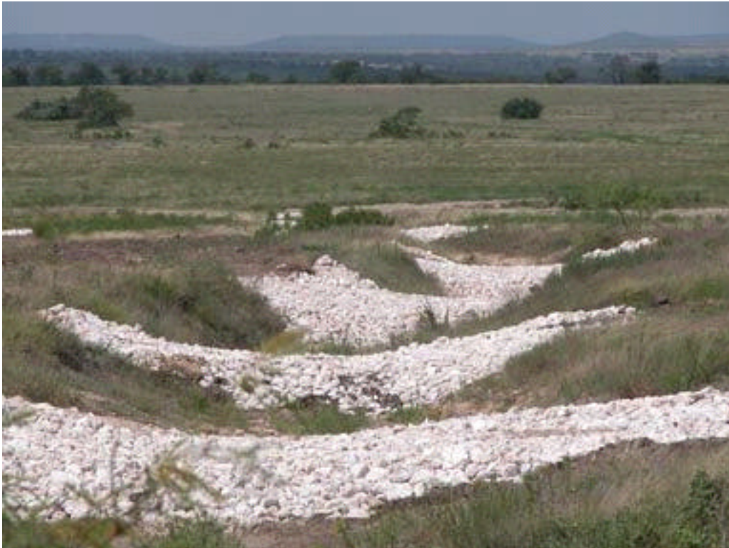
Figure C5. After-construction photograph of check dams in TA 52 that have helped reduce soil erosion while keeping the TA open (D. Jones, Fort Hood).
