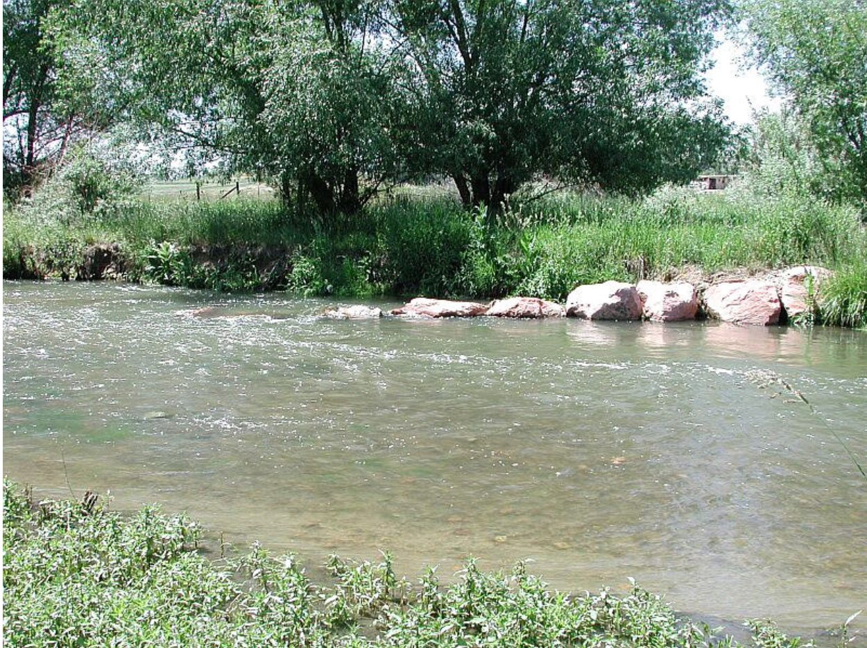
Figure B21. Rock weirs were used to help reduce velocity and cutting for stabilizing a stream in Colorado (source: USDA).
