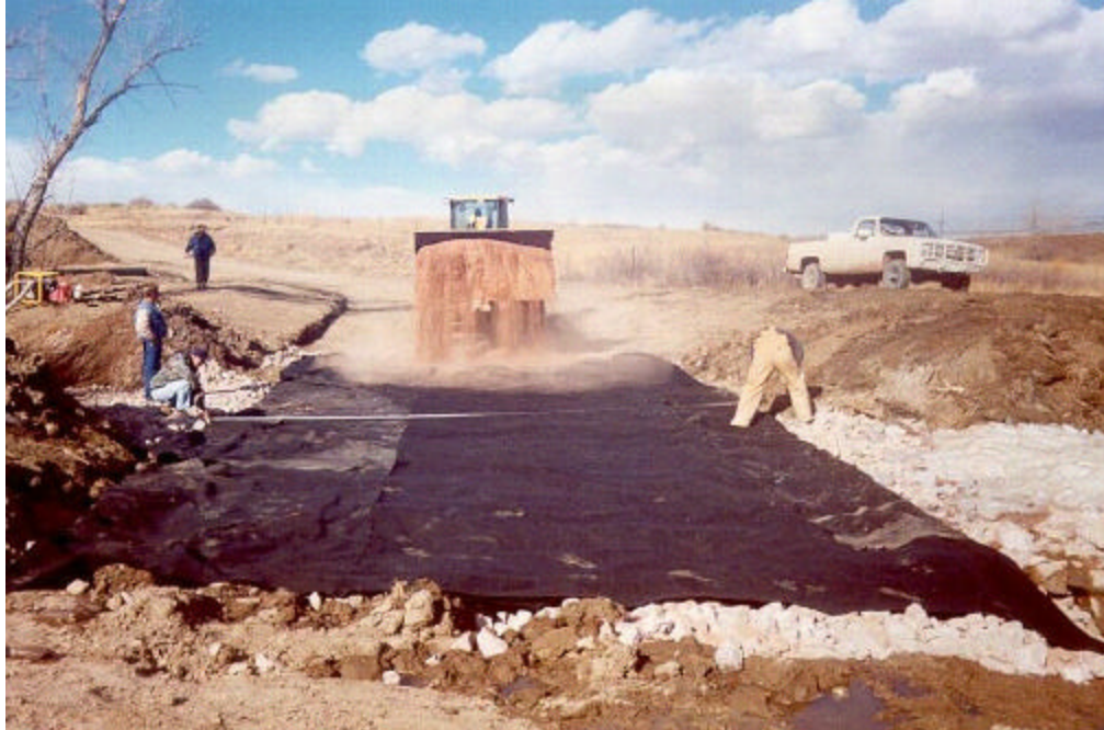
Figure B26. This nonwoven geotextile fabric was used in a low-water crossing at Fort Carson, CO, for both flow interception and structural reinforcement. Nonwoven geotextiles are used in areas that are generally saturated; consult a local vendor for help.
