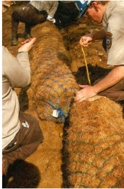
Figure B17. A close view of a coconut fiber log (BioDRAW®).
