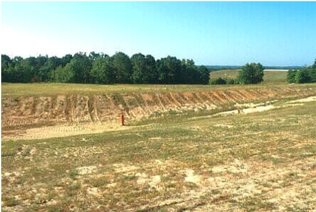
Figure B36. Terracing system on military drop zone.
