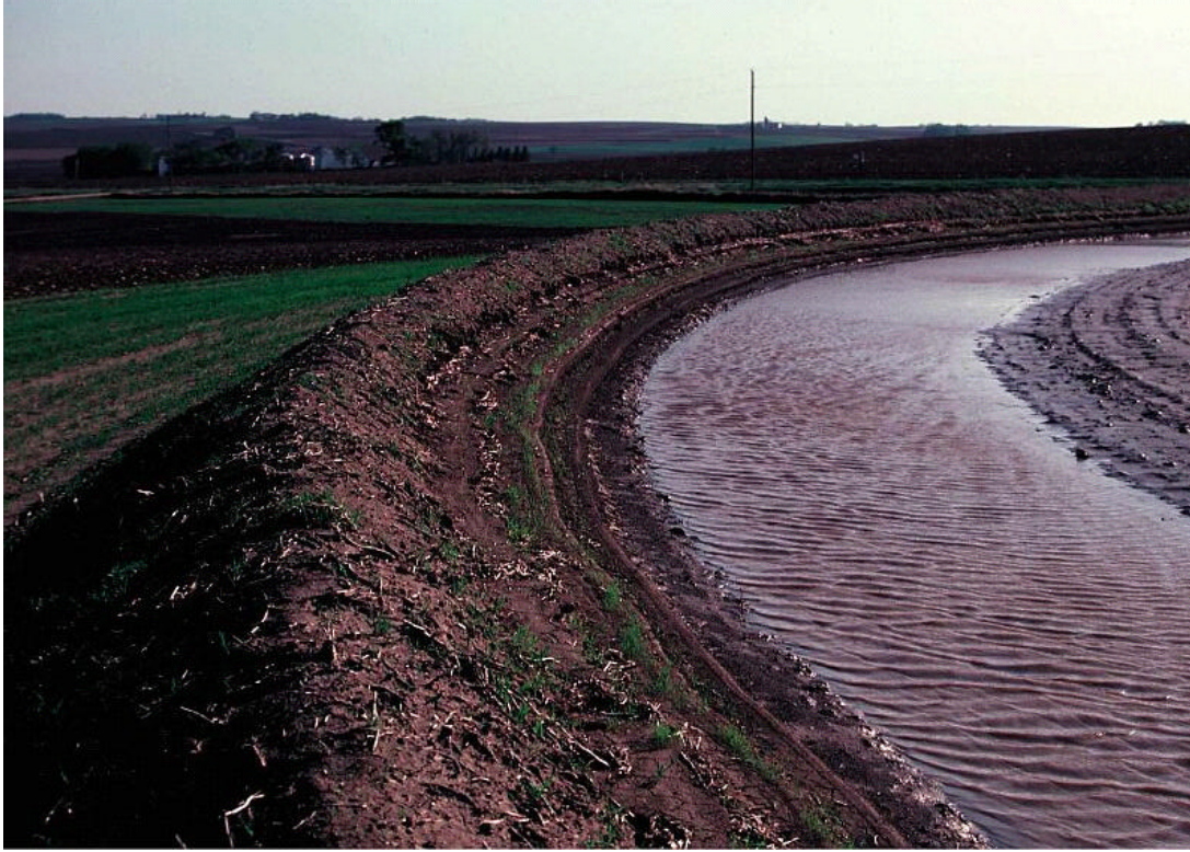
Figure B35. Newly constructed terrace on farmland (source: USDA).
