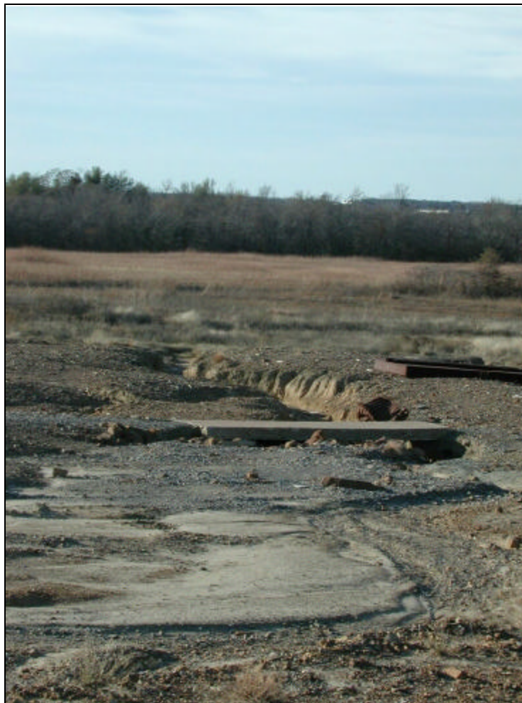
Figure A5. Combination of sheet, rill, and gully erosion on military facility.
