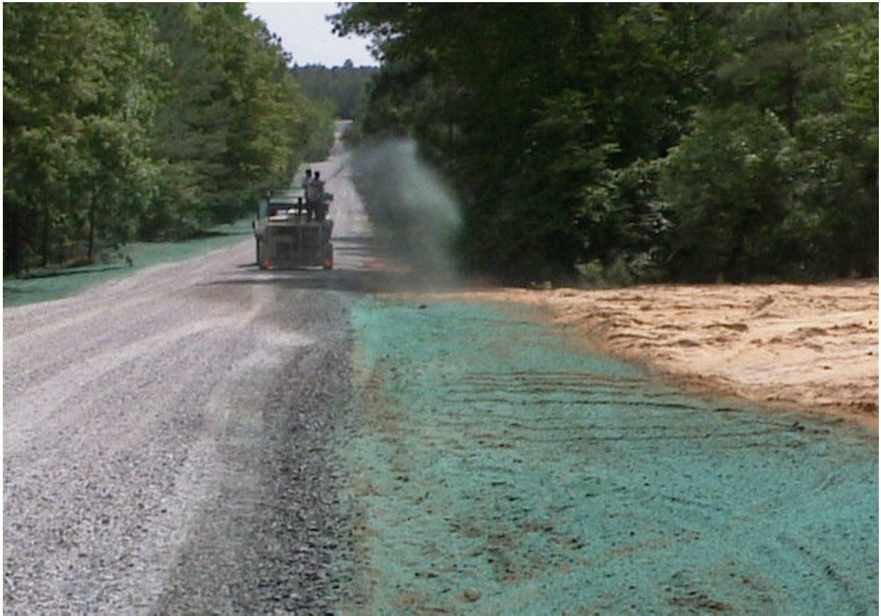
Figure B23. Application of hydraulic mulch and seed at Fort Bragg, NC.
