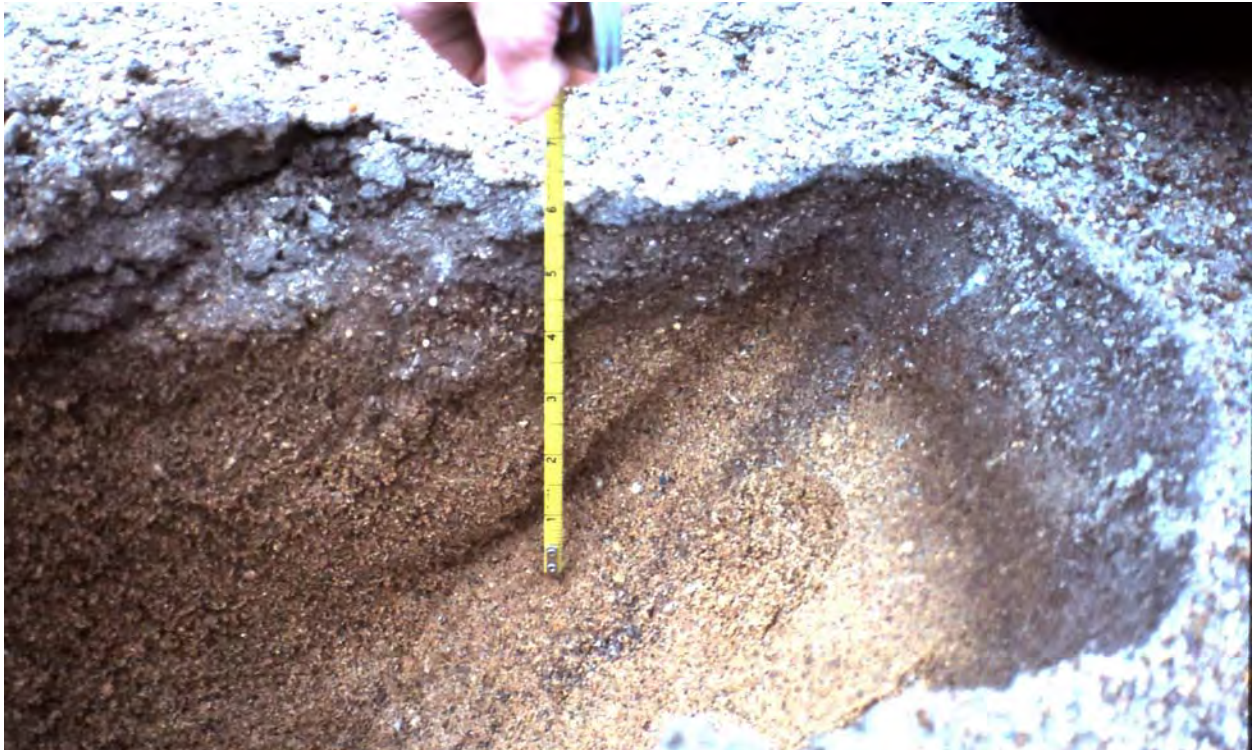
Figure A-38. Surface of a sand filter with 2-3 in. of hard crust (photo by ERDC-CERL).
