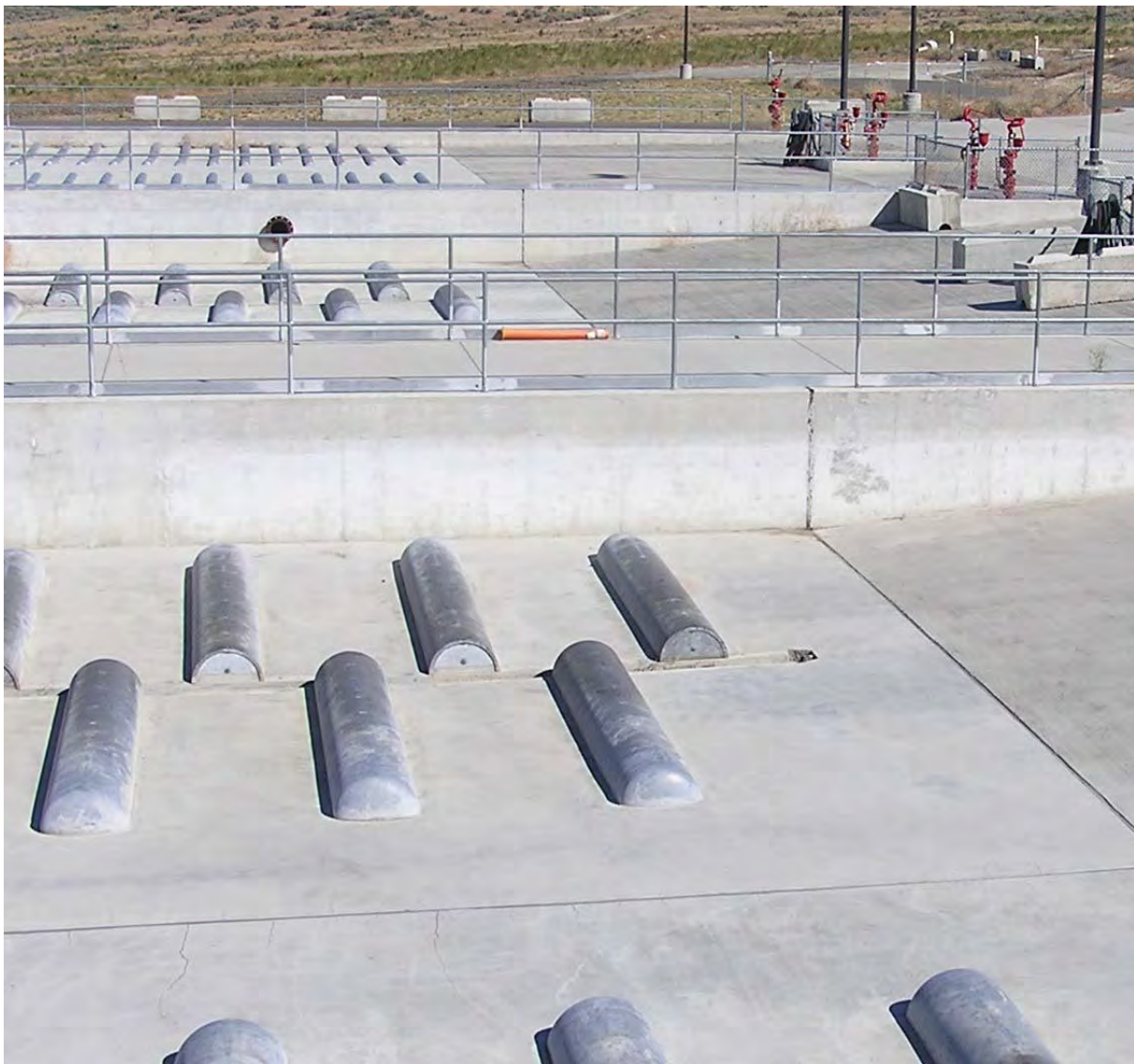
Figure A-8. Three two-lane baths at Yakima Training Center CVWF (photo by ERDC-CERL).
