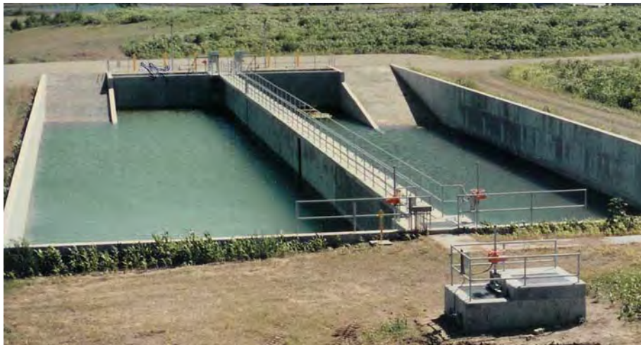
Figure A-18. Sedimentation basins with splitter box in foreground (photo by ERDC-CERL).
