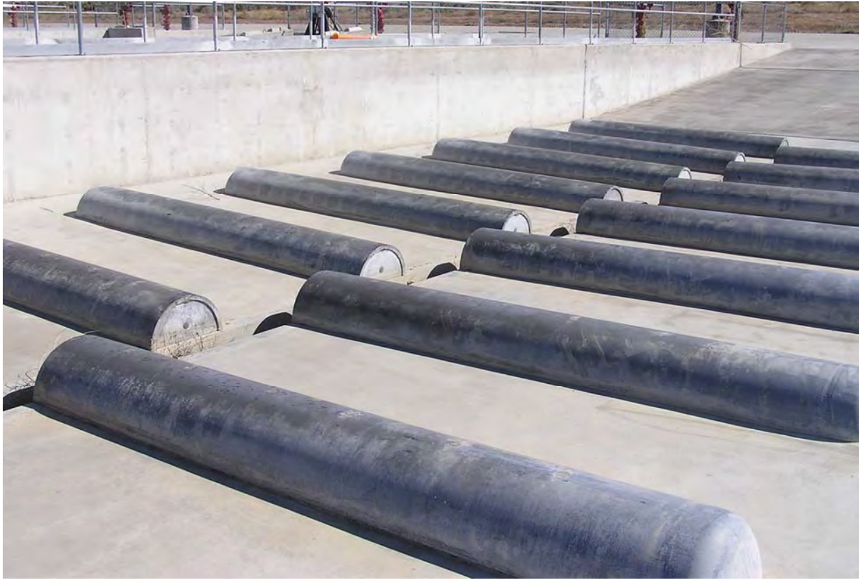
Figure A-9. Offset flexors in tracked-vehicle lane at Yakima Training Center CVWF (photo by ERDC-CERL).
