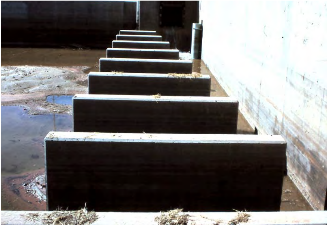
Figure A-19. Trough-like sedimentation basin inlet flow distribution structure (photo by ERDC-CERL).
