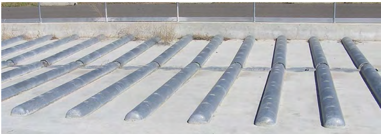
Figure A-10. Dual-purpose lane flexors at Yakima Training Center CVWF (photo by ERDC-CERL).
