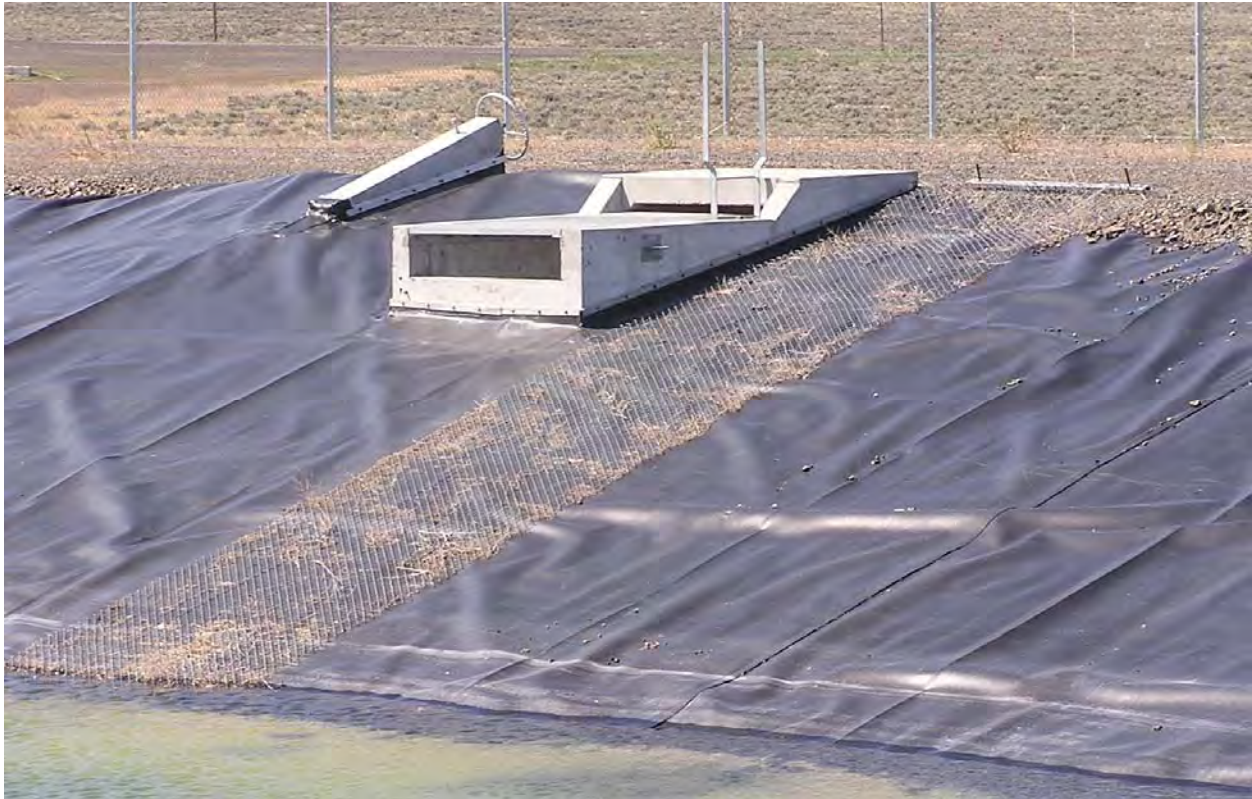
Figure A-28. Chain link can be used as a ladder for animals to escape basins (photo by ERDC-CERL).
