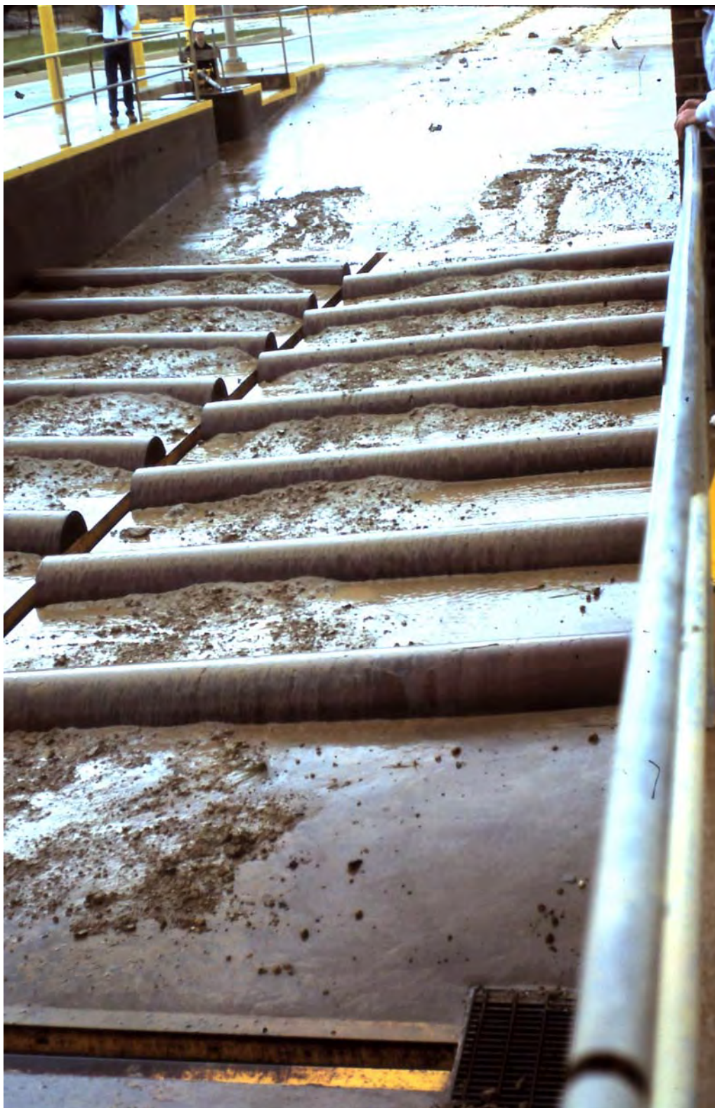
Figure A-14. Drained bath prior to a cleanout (photo by ERDC-CERL).
