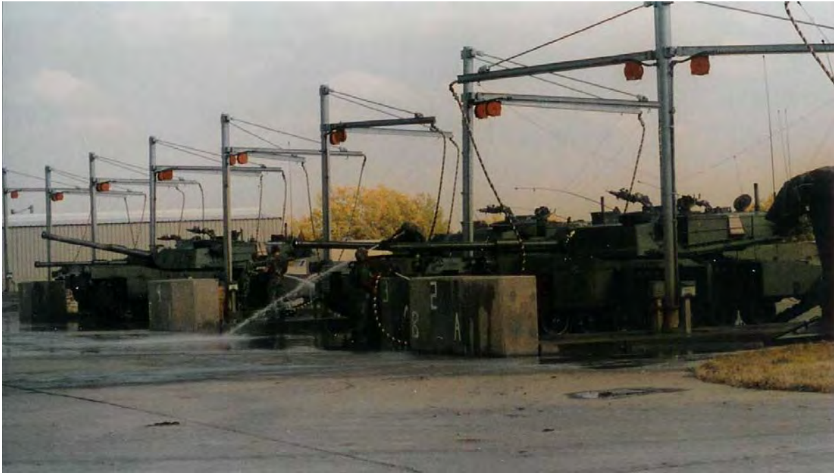
Figure A-17. M-1 tanks at wash stations (photo by ERDC-CERL).
