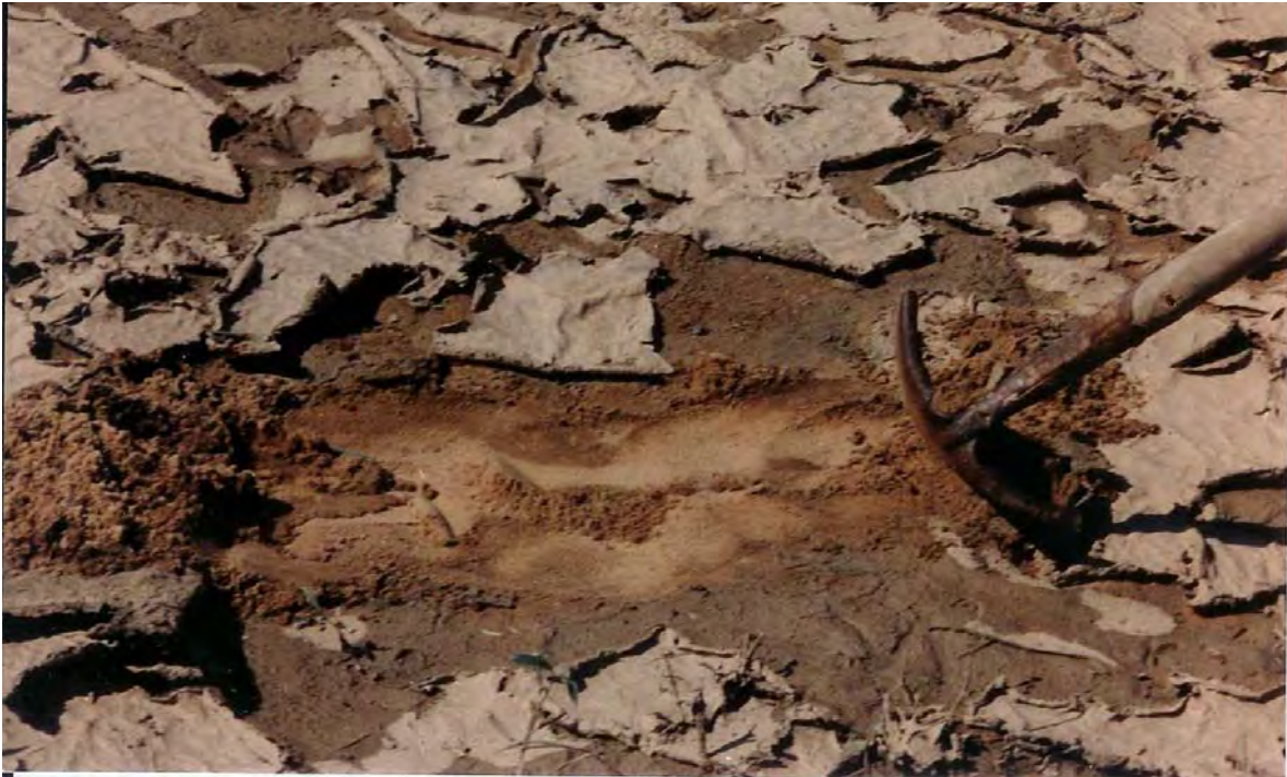
Figure A-37. Surface of sand filter that needs to be scraped (photo by ERDC-CERL).
