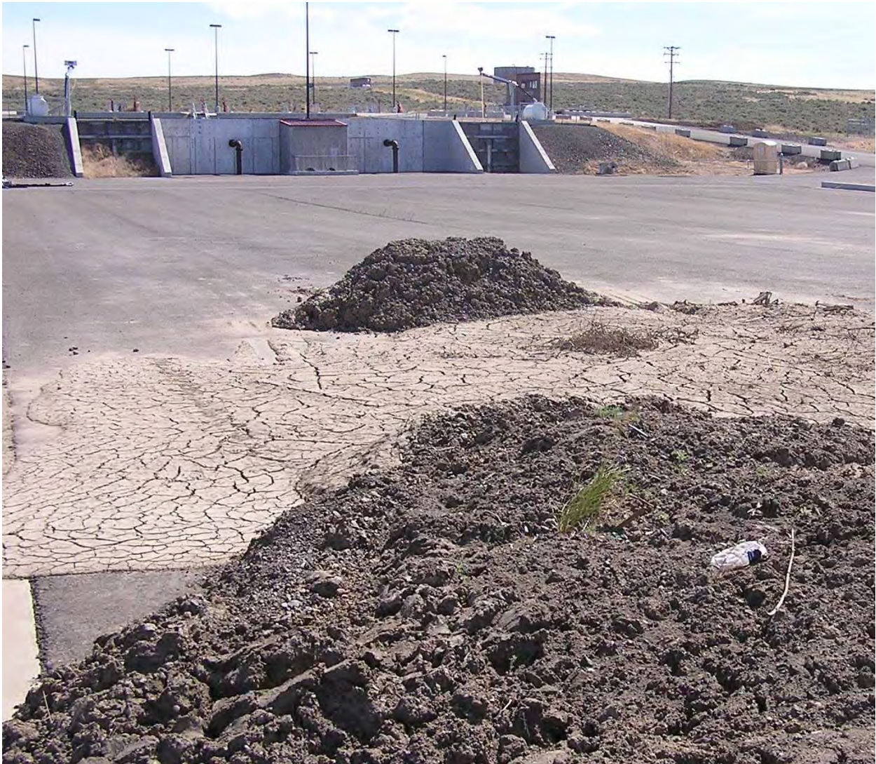
Figure A-32. Sediment drying area adjacent to sedimentation basins at the Yakima CVWF (photo by ERDC-CERL).
