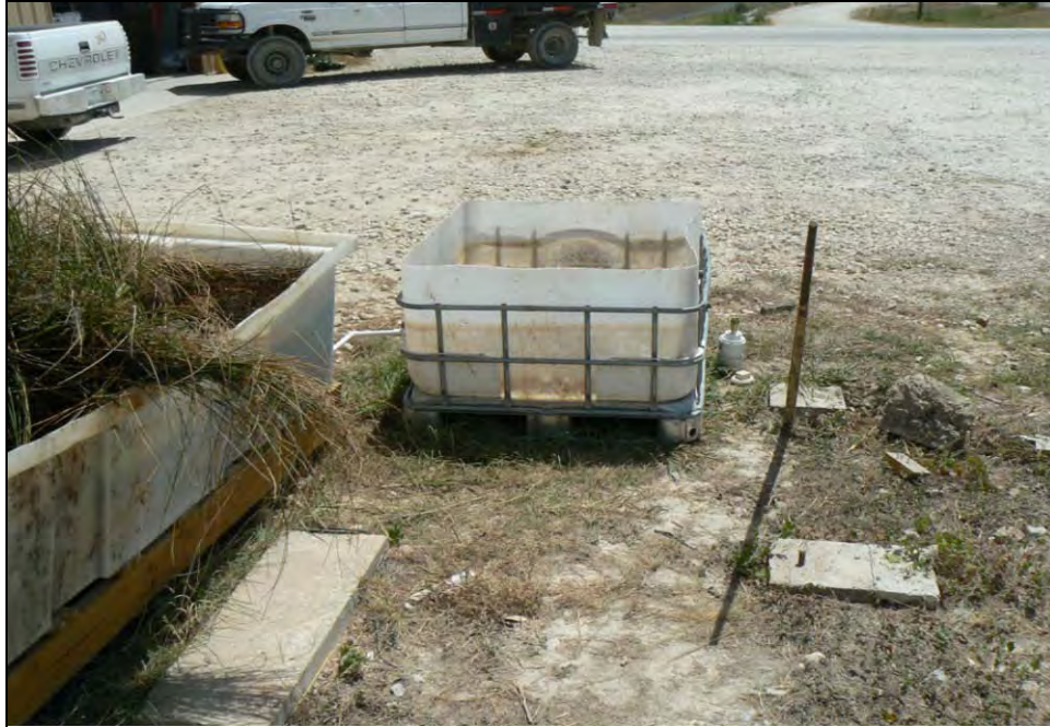
Figure A-13. Aeration container: step 6 (final) in polishing system.
