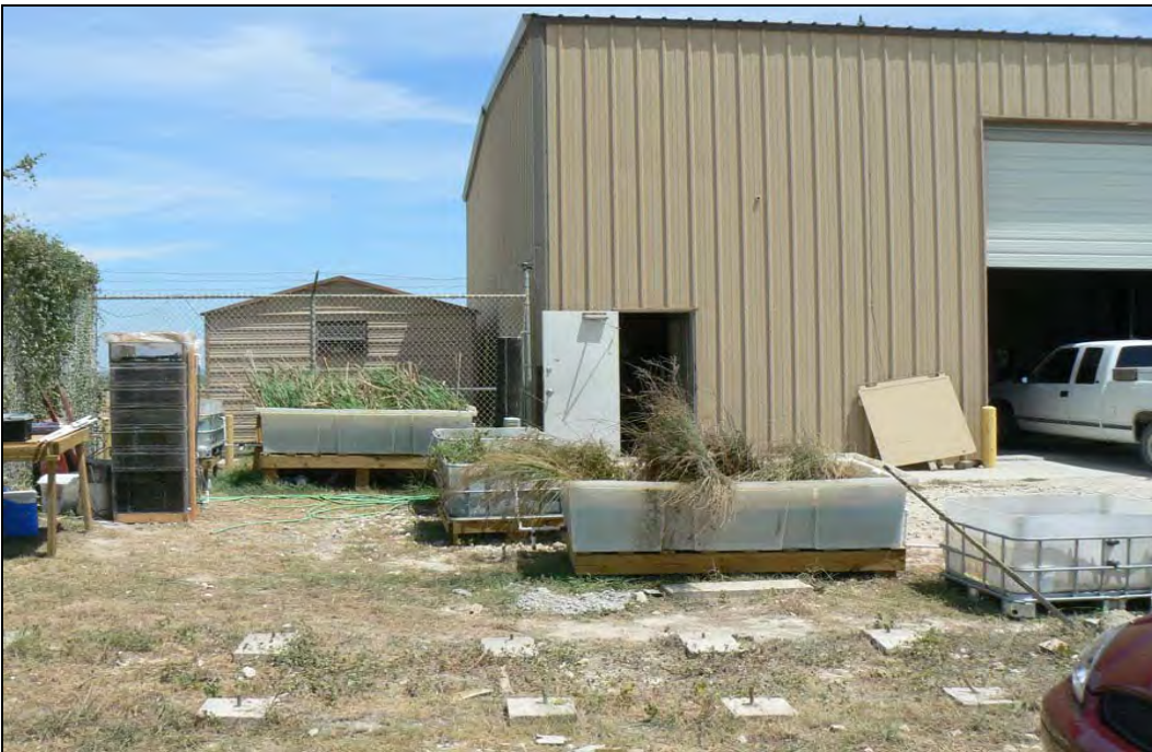
Figure A-15. Complete microbial mat and polishing treatment system (View 2).
