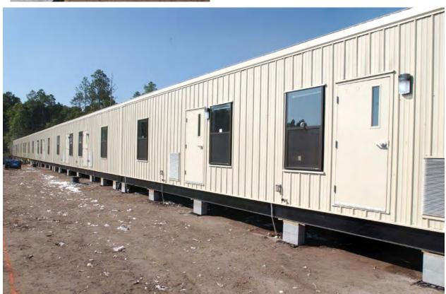
Figure A-4. Joined modular units awaiting exterior work.
