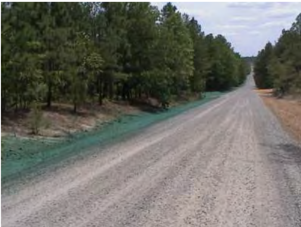
Figure F-6. Often hydroseeding may be the only Army CARES option for seeding steep slopes and narrow, long road shoulders.
