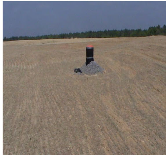
Figure C-7. Installed Higginbottom terrace inlet riser with gravel piled around it.
