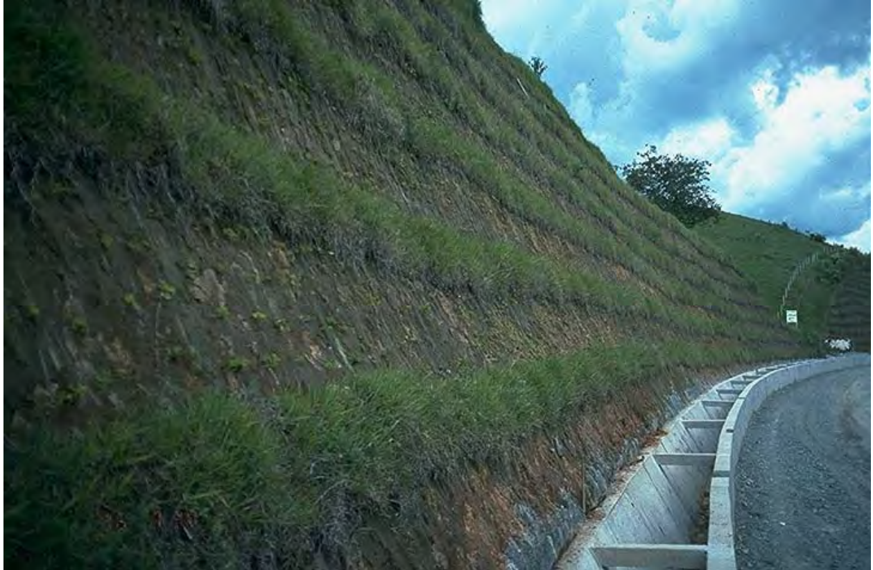
Figure B-2. Hedge grasses may be the only choice of vegetation on steep slopes.
