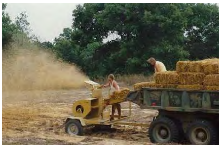
Figure C-11. Grain straw mulch applied at 4,000 lb/acre.
