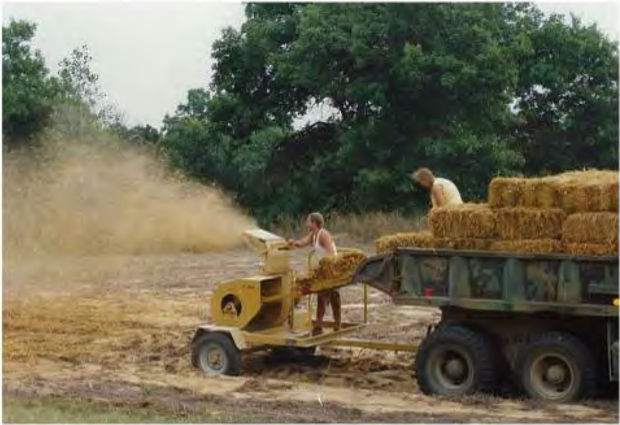
Figure B-3. Grain straw mulch applied at 4,000 lb/acre.
