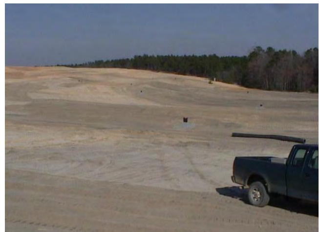
Figure C-10. Smooth, firm area to be seeded.
