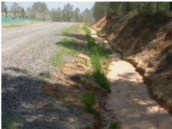
Figure F-9. Many revegetation failures can be traced to simple neglect, e.g., failure to construct check dams (left) or rill erosion (right).
