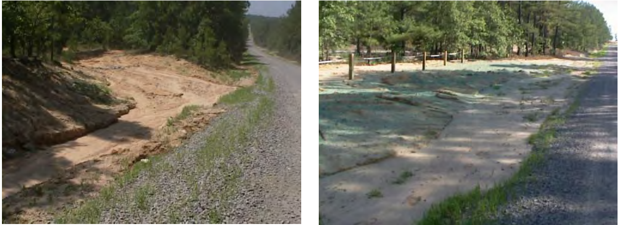
Figure F-7. In surface runoff and sediment problems, attack the source (origin, left) before implementing control measures (right) because it pays to "nip the evil in the bud."
