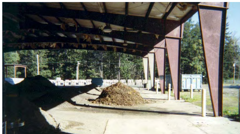
Figure A-12. Fort Lewis covered compost demonstration facility (side view).
