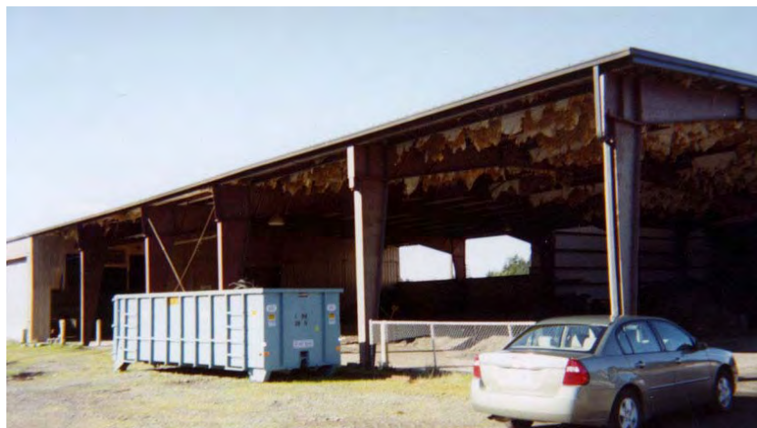
Figure A-11. Fort Lewis covered compost demonstration facility (front view).
