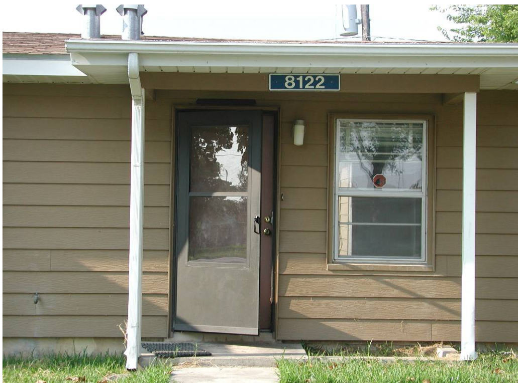
Figure B6. One story slab-on-grade housing unit (front door).
