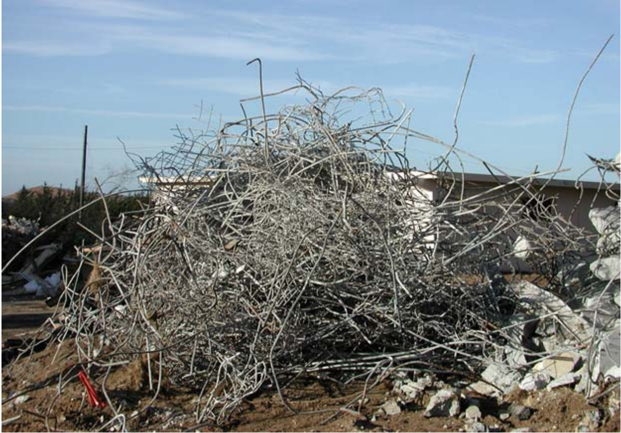
Figure C2. Scrap metal rebar separated for recycling.
