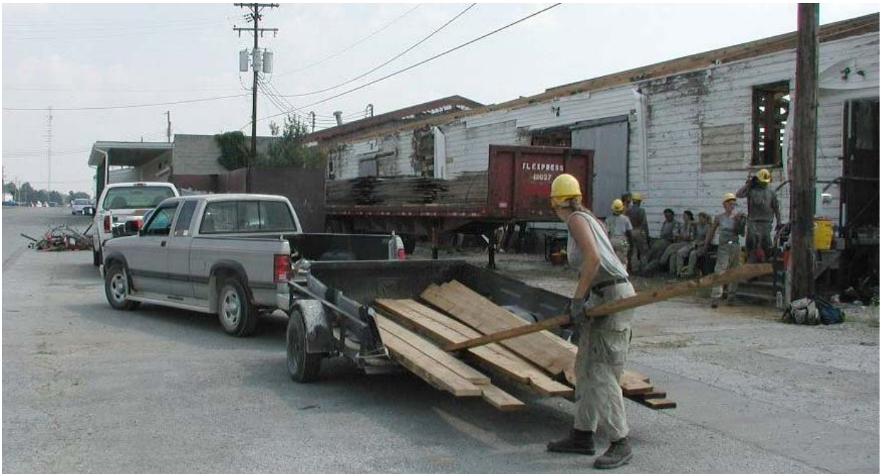
Figure C3. A worker loads salvaged lumber for recycling.
