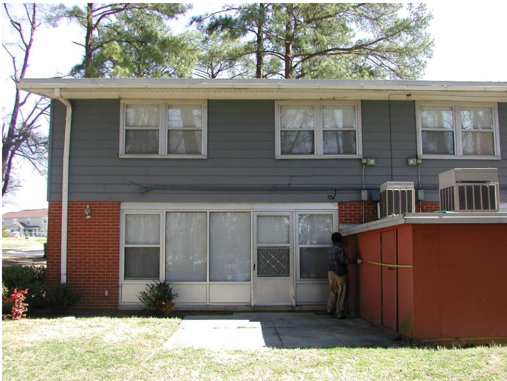
Figure B3. Exterior rear façade of one individual housing unit.
