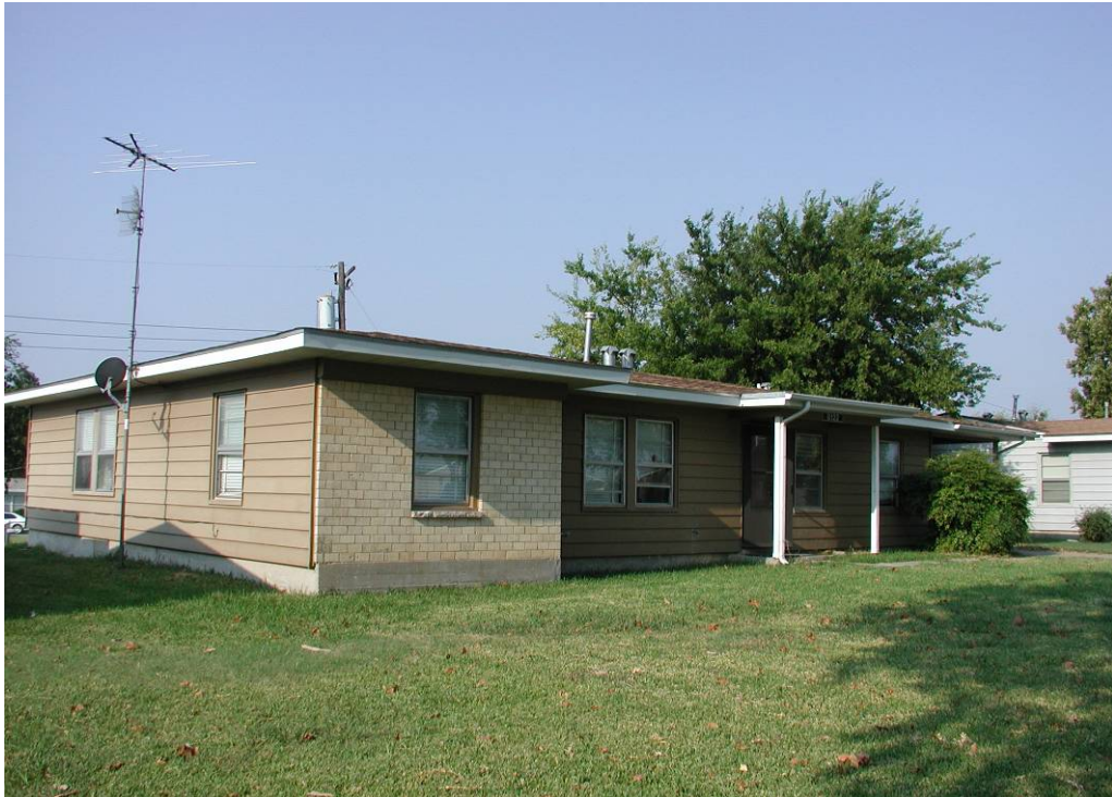
Figure B5. One story slab-on-grade housing unit.
