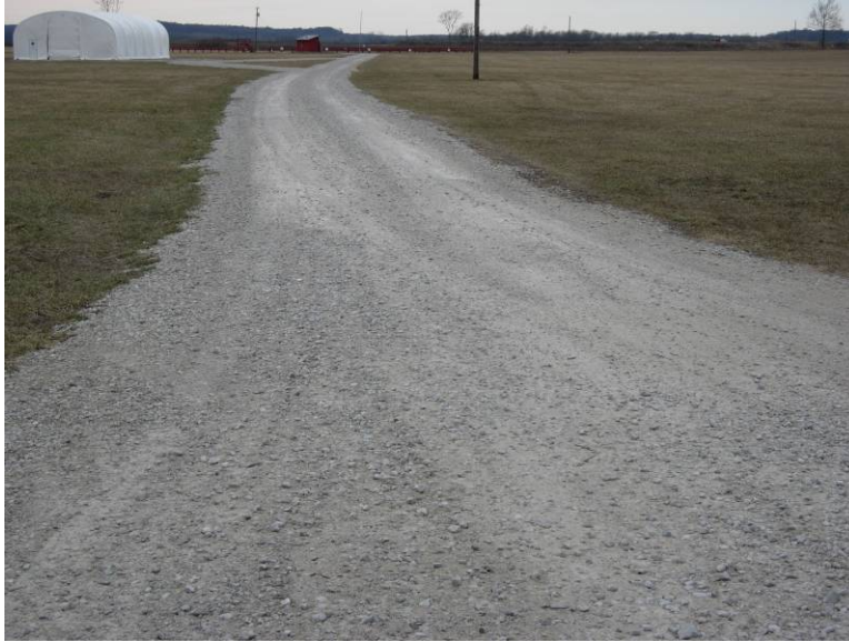
Figure B.3. Improved road with low erosion at Camp Atterbury
