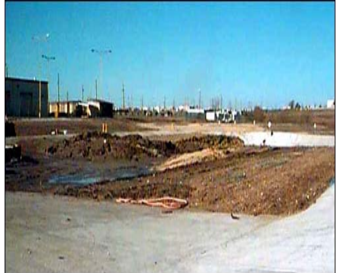
POL-Contaminated Soil Undergoing Biological Treatment
