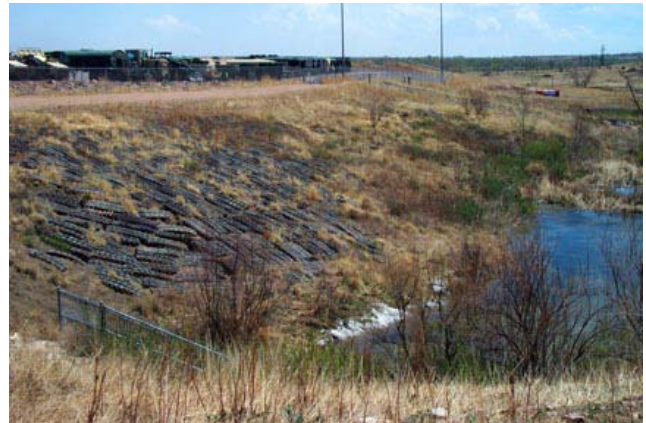
Tank Tracks Used for Erosion Control
