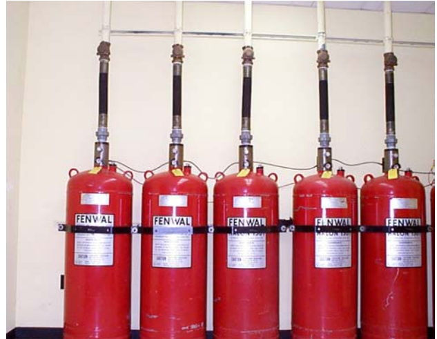
Flight Simulator Halon 1301 Suppression System
