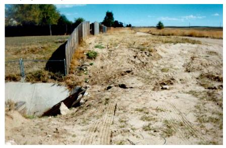
Figure 1. Unstable culvert inlet.
