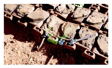
Figure 19. Using clamps to secure the cables.
