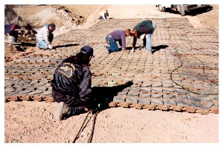
Figure 18. Using cables to string the tracks together.
