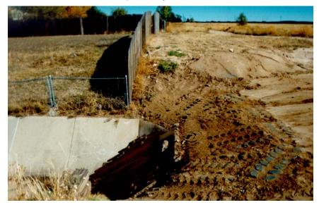
Figure 2. Stabilized culvert inlet.
