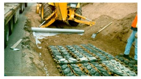
Figure 3. A drainage channel lined with geotextile and tank tracks.
