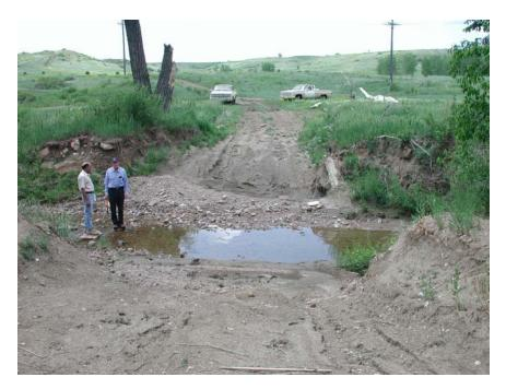
Figure 11. Heavily trafficked tank trail crossing before hardening.
