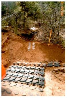
Figure 6. Tank tracks lining a natural inlet.
