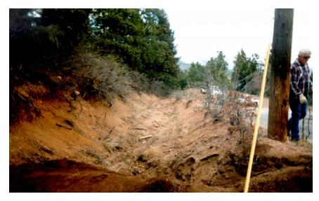
Figure 8. Erosion and scouring downstream from the project site.
