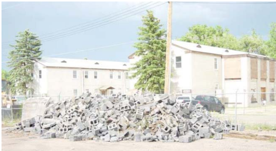
Figure B-16. Cinder block intended for recycling from Building 6286, but instead disposed as rubble due to unavailability of rock crusher (Innovar 2005).
