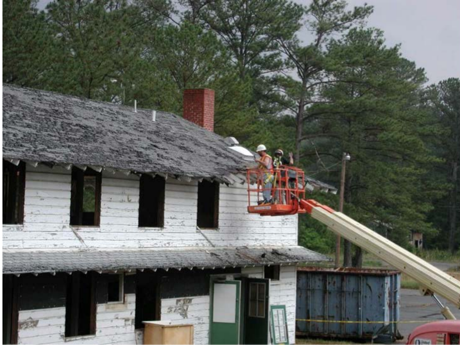
Figure A-3. Removing eaves at Fort McClellan in 2003 (Joyce Baird, ERDC-CERL).
