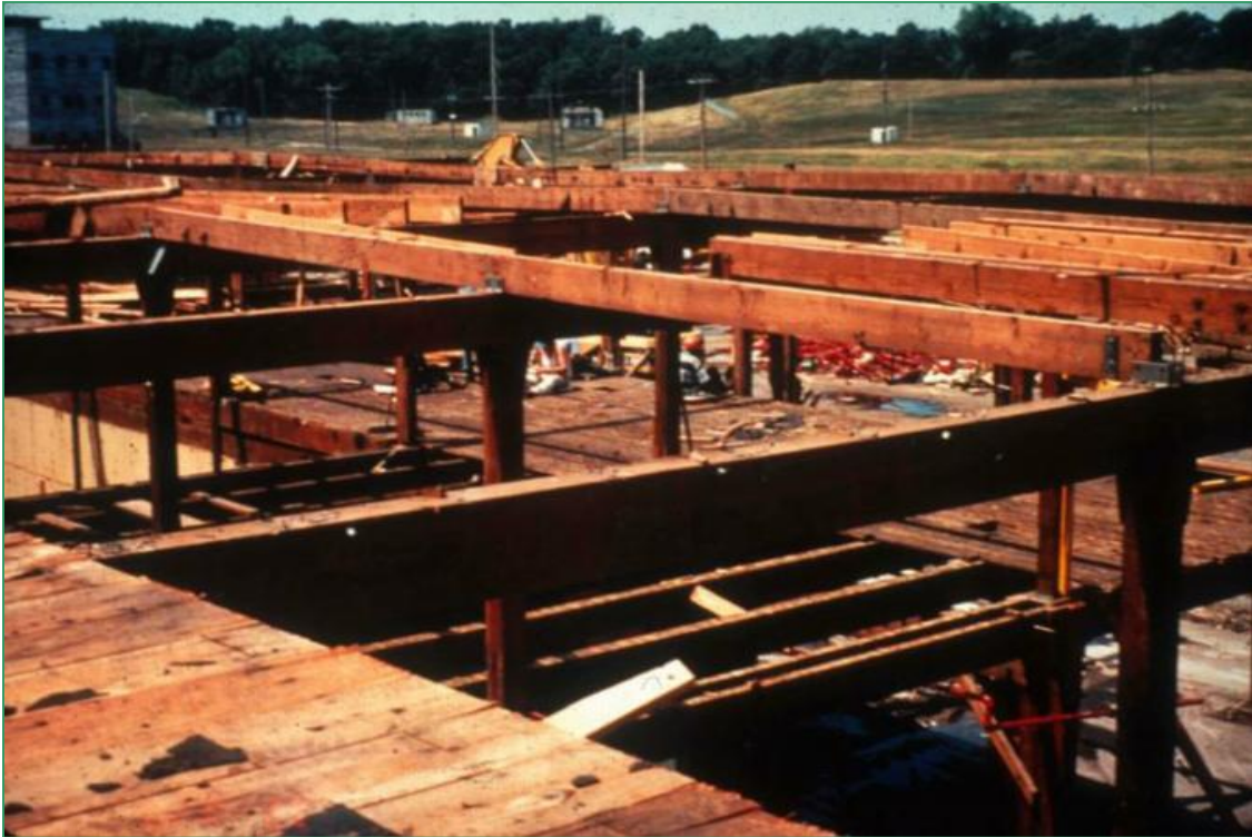
Figure B-17. Timber salvage at TCAAP in 1995 (TCAAP).
