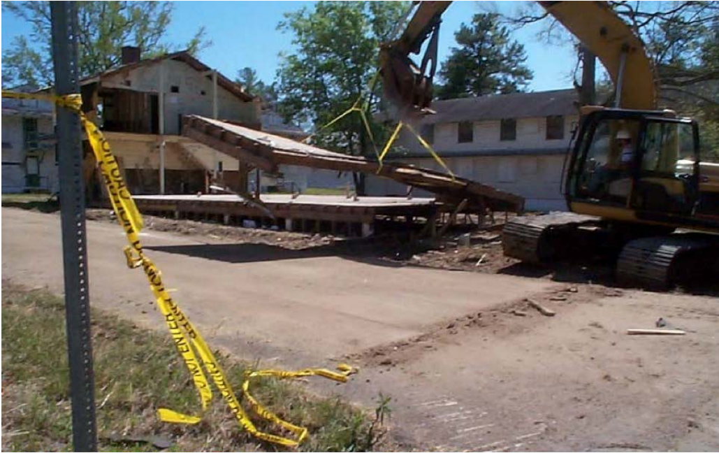
Figure A-5. Floor panelization at Fort McClellan in 2003 (Joyce Baird, ERDC-CERL).
