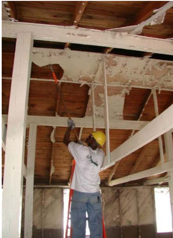
Figure A-2. Removing drywall in 2003 at Fort McClellan (Joyce Baird, ERDC-CERL).
