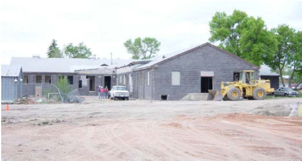
Figure B-8. Building 6286 at Fort Carson, showing CMU exterior shortly before deconstruction (Innovar 2005).
