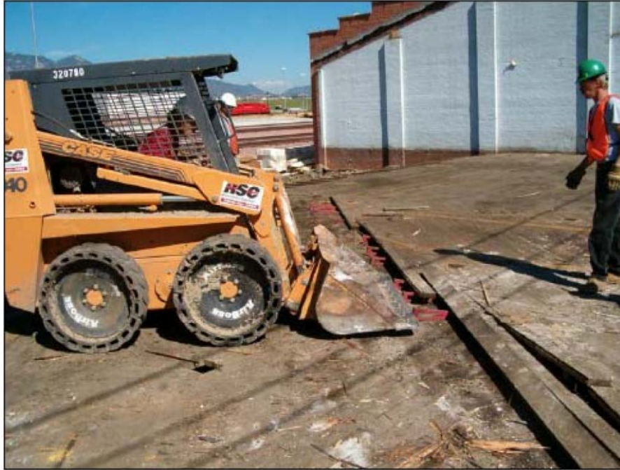
Figure B-14. Removing flooring with skid-steer loader at Building 227 (Innovar 2005).
