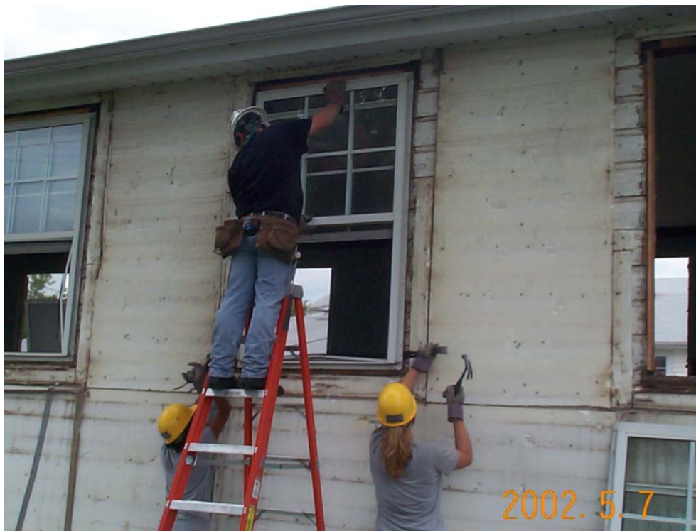
Figure A-4. Removing windows at Fort Campbell in 2002 (Joyce Baird, ERDC-CERL).
