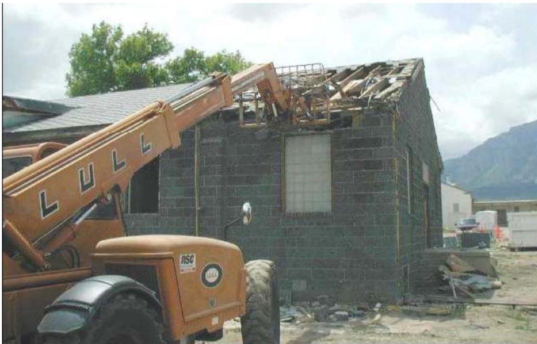
Figure B-10. Reach forklift removing a roof section of Building 6286 (Innovar 2005).
