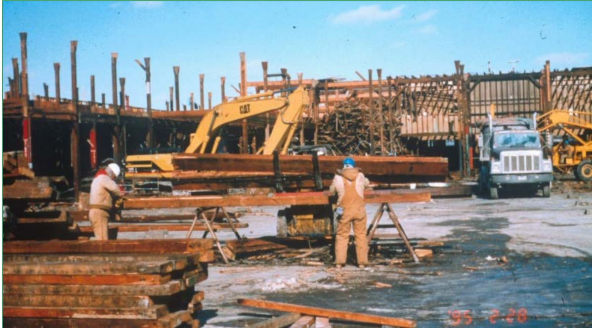
Figure B-18. Timber salvage at TCAAP in 1995 (TCAAP).
