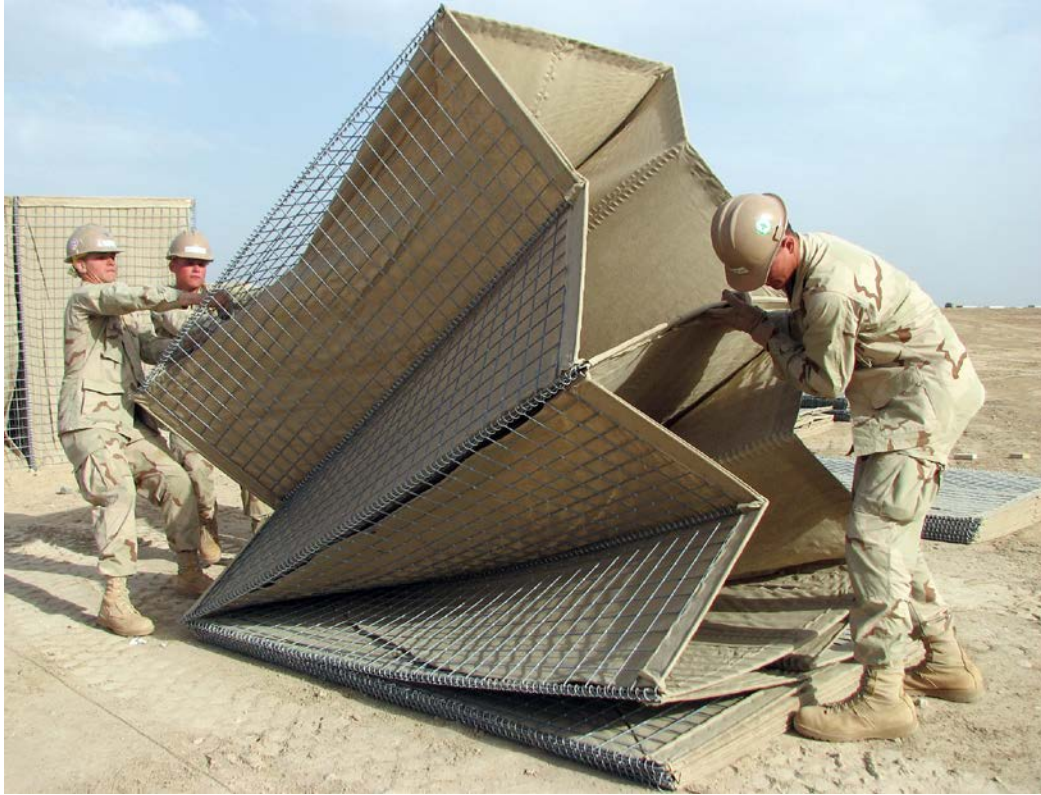
Figure D-10. U.S. Navy personnel assembling HESCO bastions (Wikipedia http://en.wikipedia.org/wiki/Hesco_bastion ).
