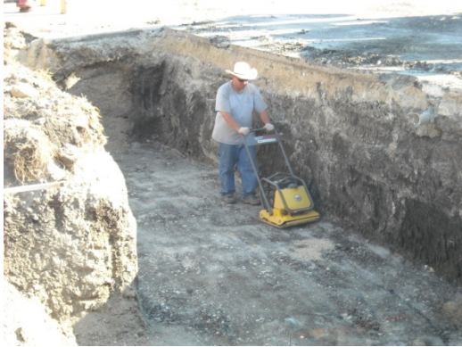
Figure B-7. Trench compaction.
