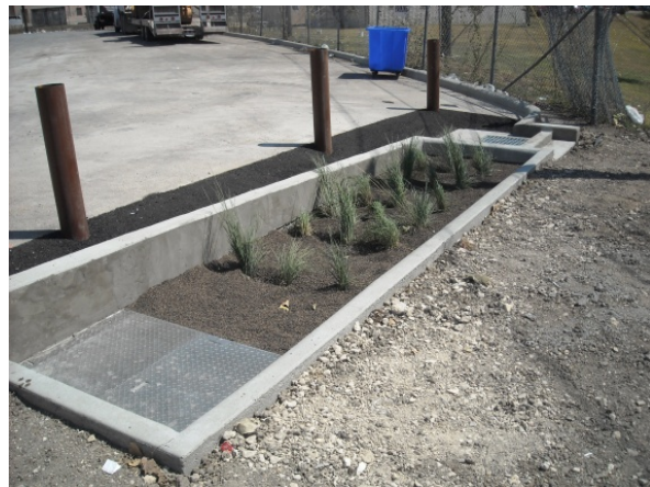
Figure B-9. Guard posts installed to protect against vehicle damage.
