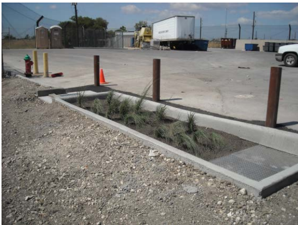
Figure B-9. Guard posts installed to protect against vehicle damage.
