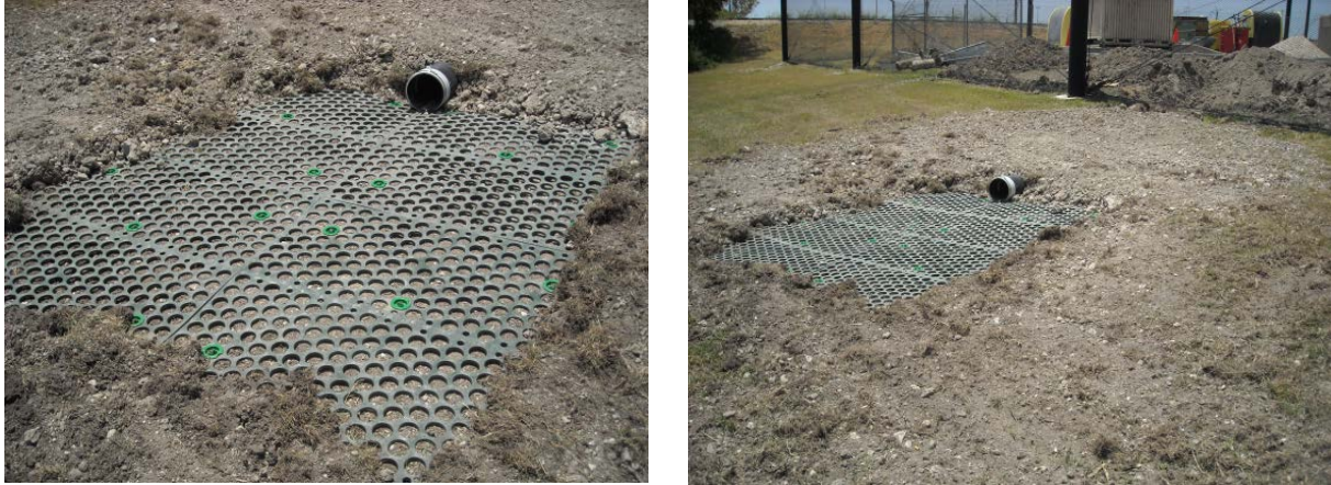
Figure B-10. Scour pads and riprap at overflow areas
