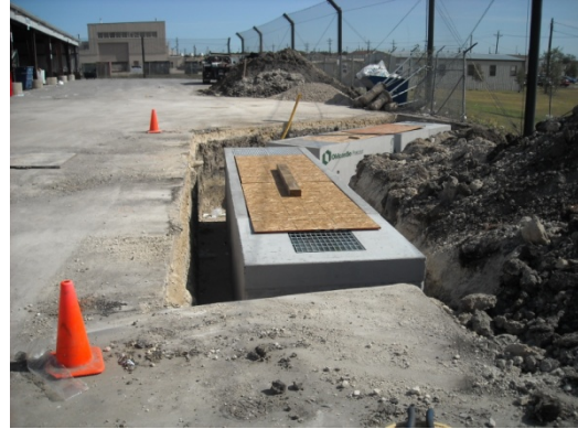
Figure B-8. MWS in place.
