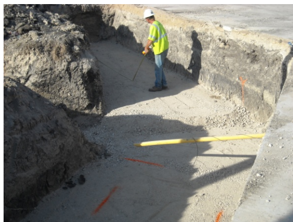
Figure B-6. Trench excavation.
