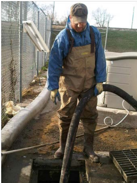
Figure B-21. Settling area being vacuumed.
