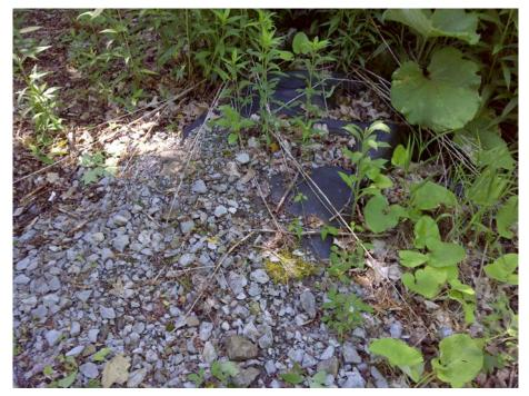
Figure B-3. Geotexttile and gravel system used to cover a hardened historic village site at Fort Drum (ERDC-CERL, 2013).
