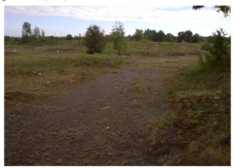
Figure B-1. Plastic geogrid netting is providing soil stabilization in an archaeologically sensitive training area at Fort Drum (ERDC-CERL, 2013).
