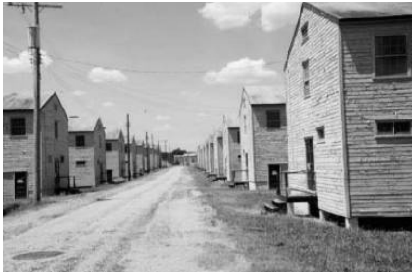
Figure D-3. Two-story, World War II-era, wood-sided Army barracks.
