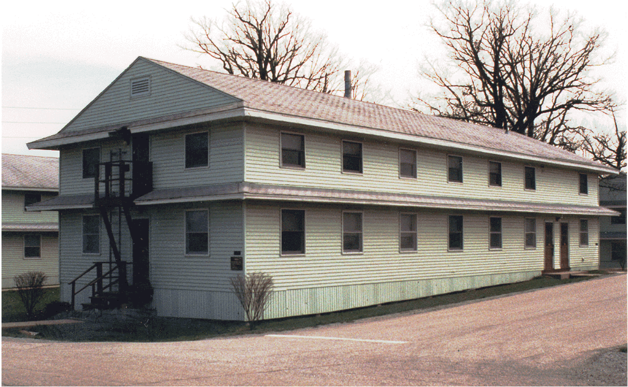
Figure D-2. Vinyl-sided, two-story Army barracks.
