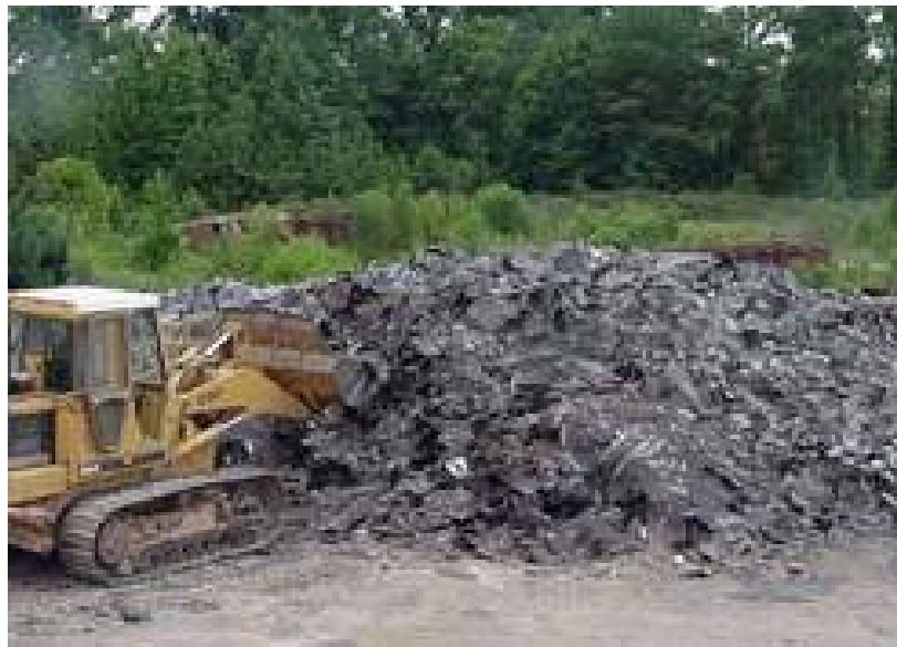
Figure C-2. Tear-off shingle waste.
