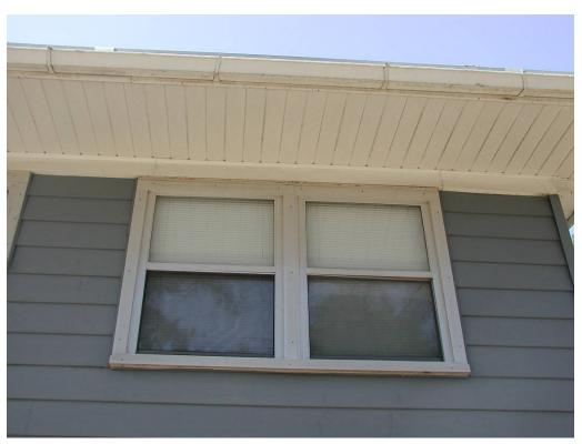
Figure B-4. Typical aluminum window of an eight-unit family housing building.
