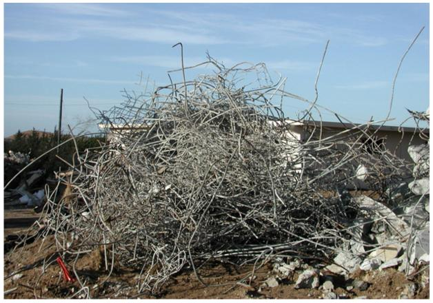
Figure C-2. Scrap metal rebar separated for recycling.
