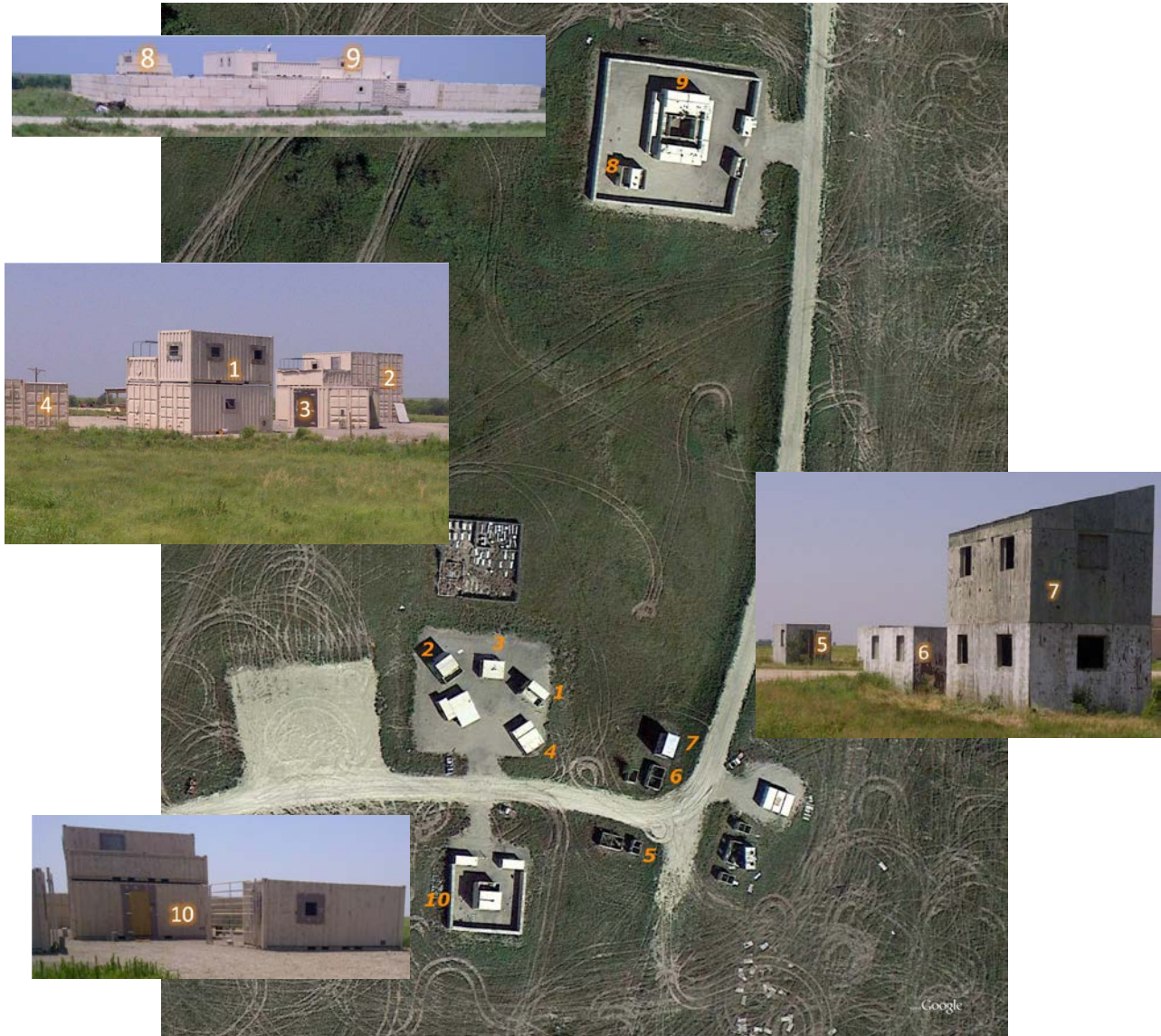
Figure A-1. Aerial view of temporary UTA site example, with the site's buildings shown in photo insets (source: Google Maps for aerial view; ERDC-CERL for photos, 2013).
