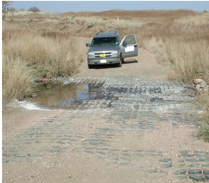
Figure C-15. Low-water crossings installed with used tank tracks as solution to erosion from vehicles crossing shallow ditches (top photo). The tank track design proved more durable than other commercial solutions, remaining in place during heavy precipitation events or high water flows (bottom photo) (ERDC-CERL).
