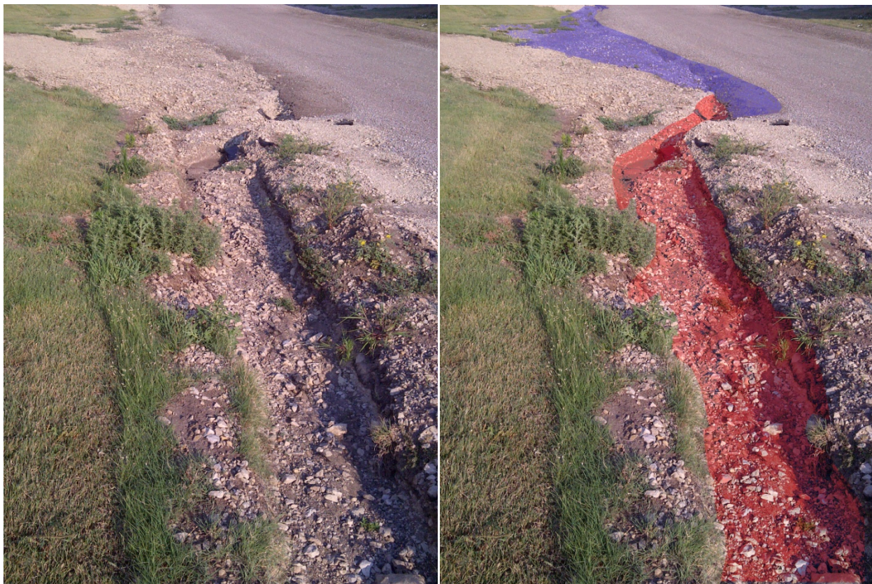
12 13 Figure C-17. Erosion caused from high-volume water flow from driveway 14 entering a roadway. Altered photo on right shows resulting erosion of gravel 15 fines (blue area) and formation of a gully (red area) (ERDC-CERL).
