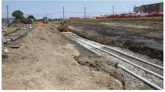
Figure B-4. Subsurface drainage system of perforated pipe installed.
