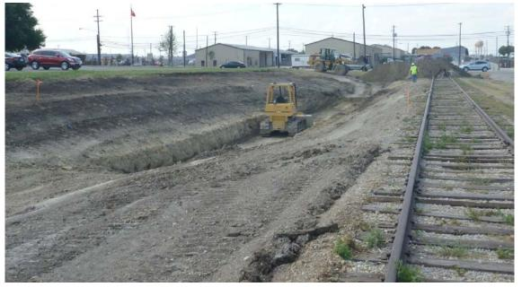
Figure B-3. Bioswale trench excavation.
