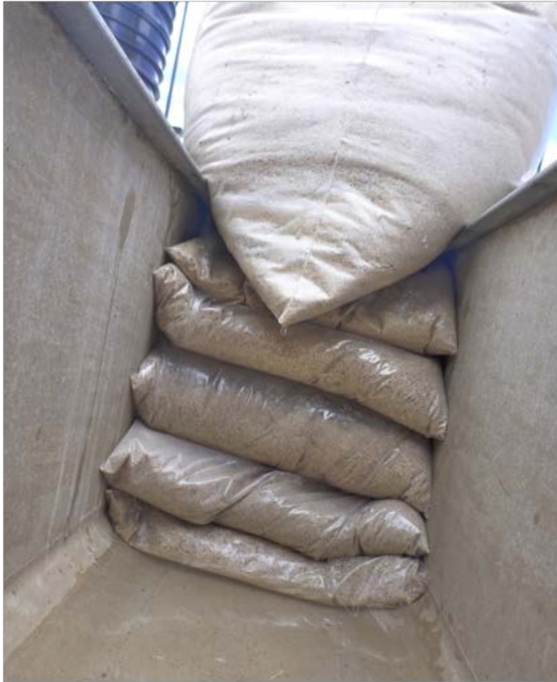
Figure B-6. Sand bag dam set up.
