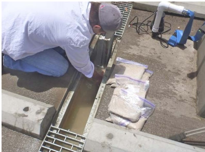
Figure B-7. Setup of the dam and sump pump in trough.
