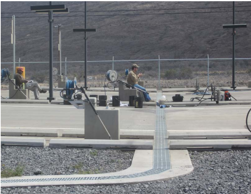
Figure B-4. CVWF concrete wash basin with trough in middle.
