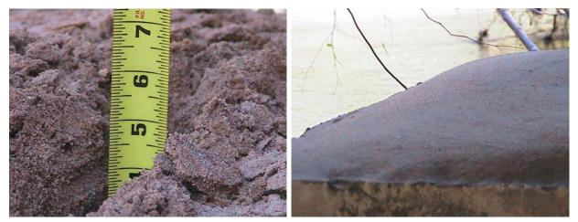
Figure E-1. At Randall Creek, 2nd Armored Division Road, one storm dumped 7 in. of sediment on a pier almost 4 ft above streambed.
