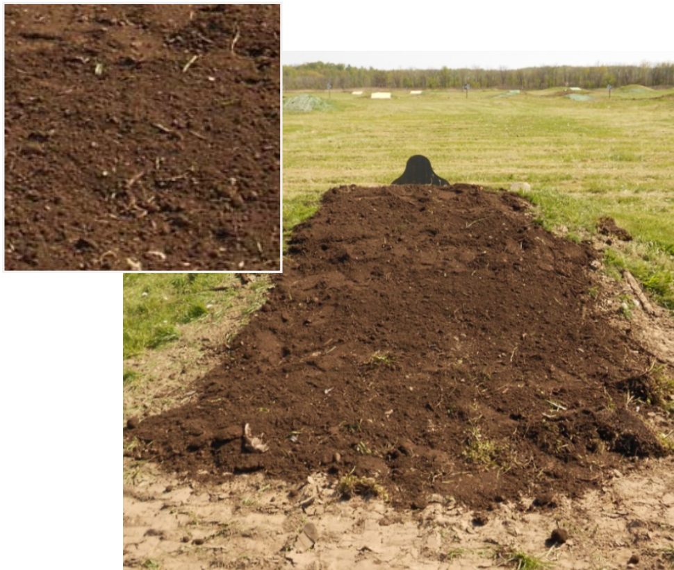
Figure B-11. Treatment #7: Compost installation (ERDC-CERL 2012).
