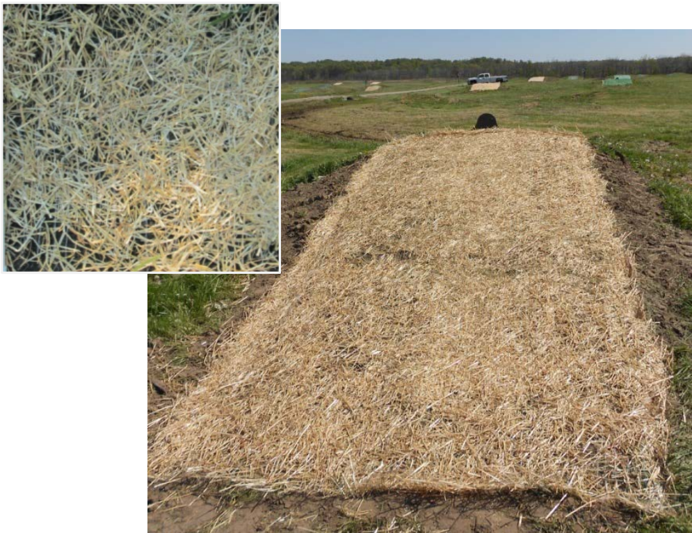
Figure B-9. Treatment #5: Double-net straw ECB treatment installation (ERDC-CERL 2012).
