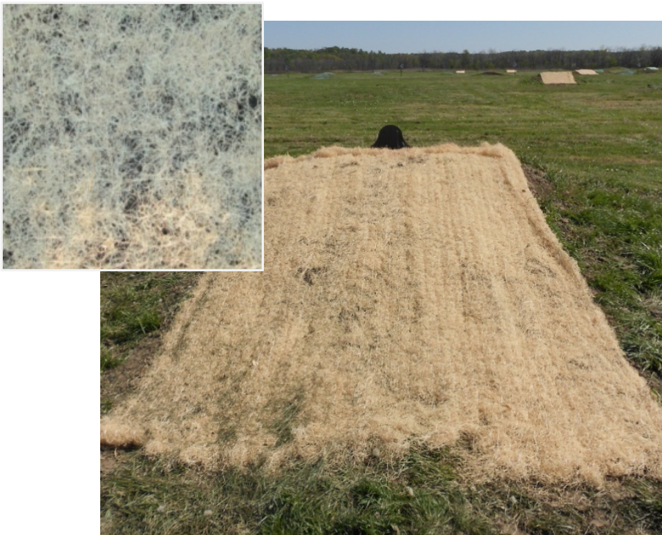
Figure B-7. Treatment #3: Net-free excelsior ECB treatment installation (ERDC-CERL 2012).
