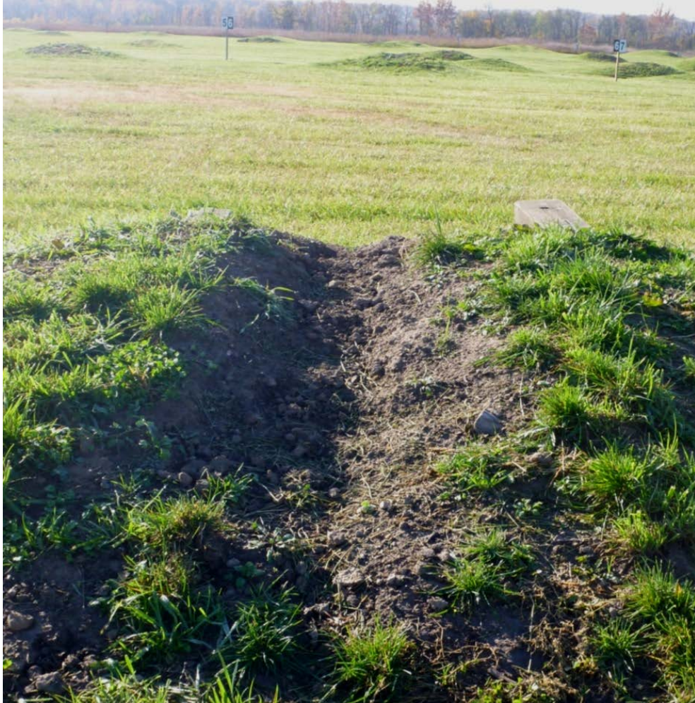
Figure B-3. Typical pattern erosion and soil loss on SIT emplacement berm at Camp Atterbury demonstration site (ERDC-CERL 2012). Note: photo is taken looking toward target.
