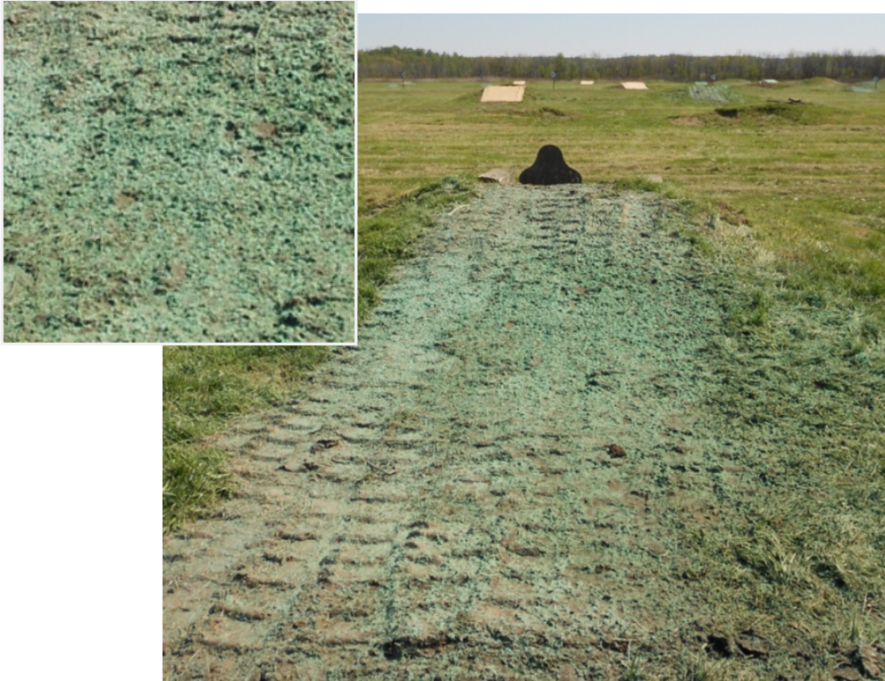
Figure B-10. Treatment #6: Hydro-mulch (Camp Atterbury current treatment) installation (ERDC-CERL 2012).
