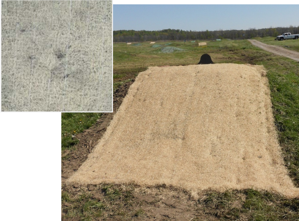
Figure B-8. Treatment #4: Double-net excelsior ECB treatment installation (ERDC-CERL 2012).
