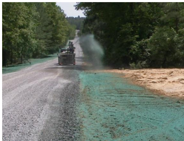
Figure C-3. Use hydroseeding for difficult shoulder areas (Phillips and Jordan).
