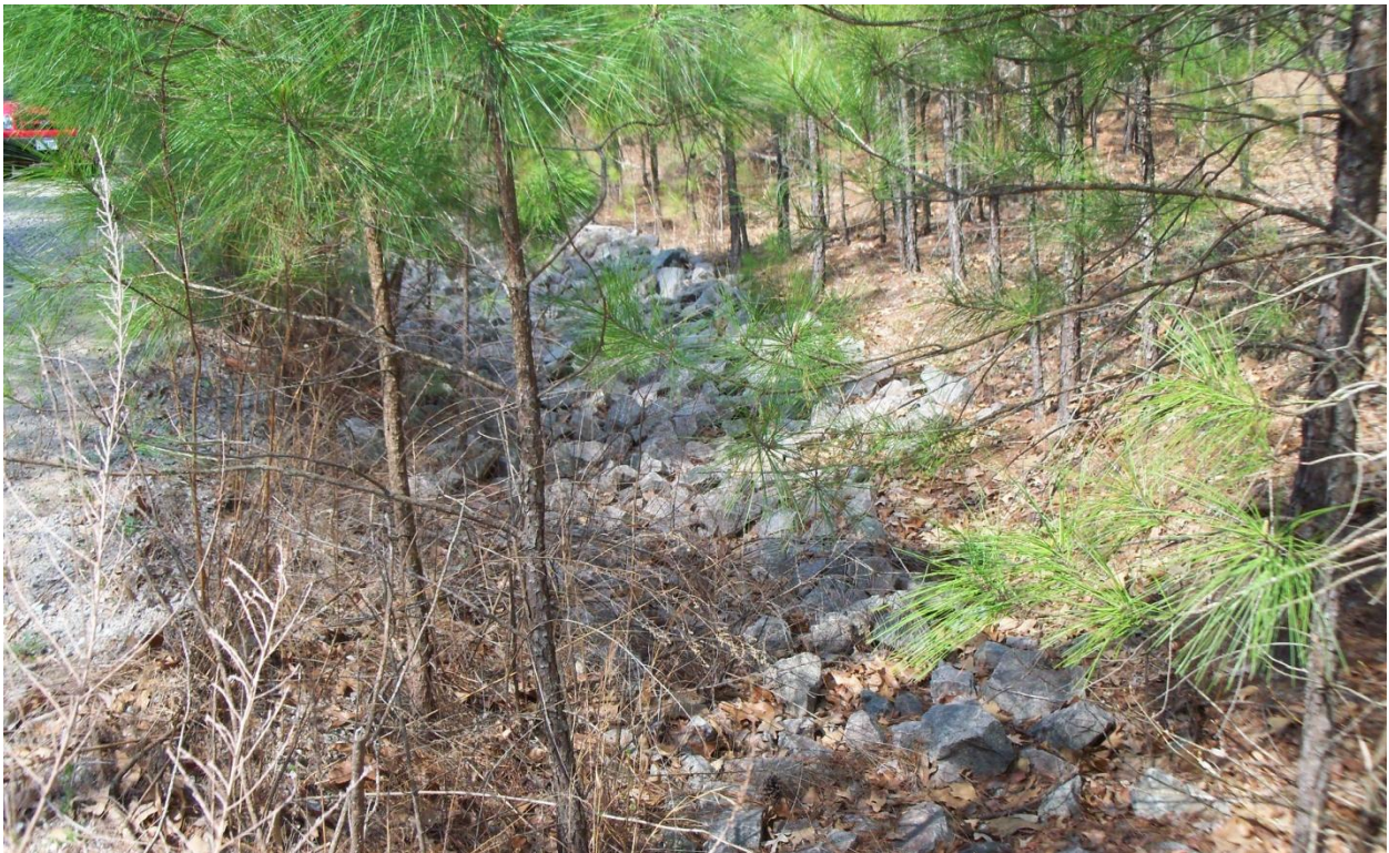
Figure B-12. Riprap in ditch along road is being used for erosion control (Phillips and Jordan, Inc.).
