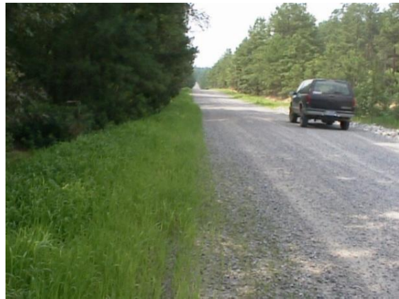
Figure C-2. Stabilize road shoulder with vegetation (ERDC-CERL).
