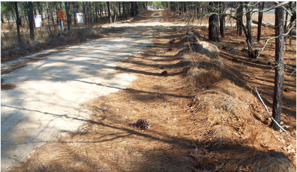
Figure B-4. Another place where ridges of soil along the side of the road prevent water from running into forest; however, the road's flatness means little damage is done (Phillips and Jordan, Inc.).
