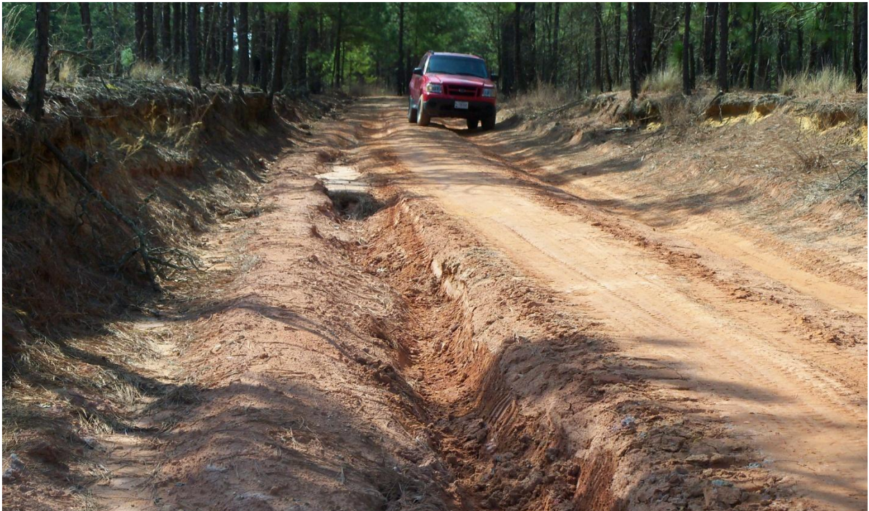
Figure B-8. Close-up of gully from previous picture. Note that headcut in gully is moving up the hill (Phillips and Jordan, Inc.).
