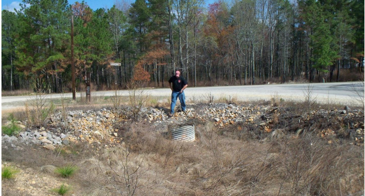
Figure B-13. Sediment basin along roadside to carry runoff away from roadway (Phillips and Jordan, Inc.).
