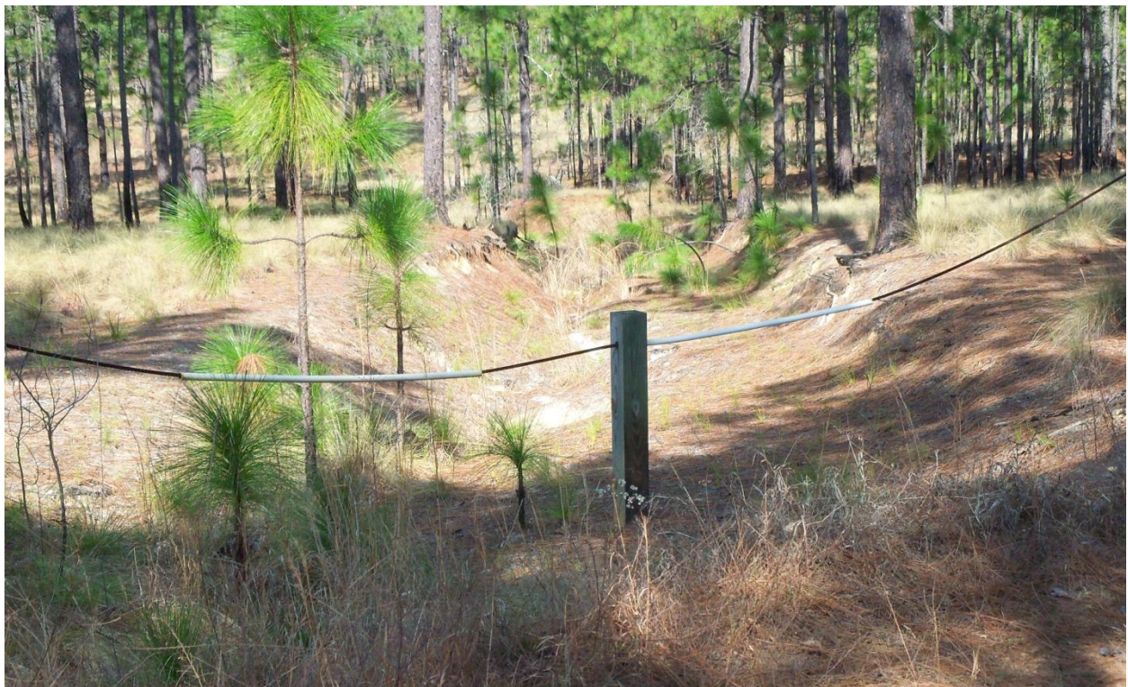
Figure B-14. Stabilized channel to convey water away from road (Phillips and Jordan, Inc.).
