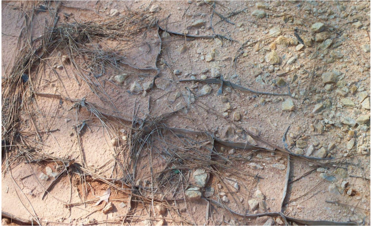
Figure B-17. Close-up of erosion control mat (Geoweb) in road surface (Phillips and Jordan, Inc.).
