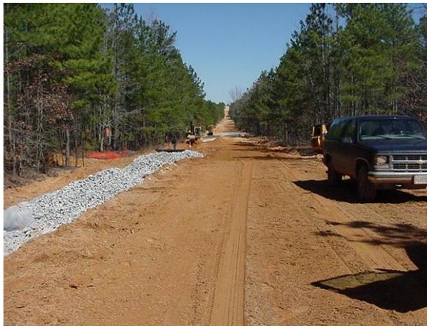
Figure B-19. Treatment #1 - layer of sandy borrow material only (ERDC-CERL).
