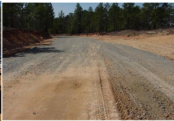
Figure B-20. Treatment #4 - fabric, 2-ft riprap cover, and 12-in. crusher run cover (ERDC-CERL).
