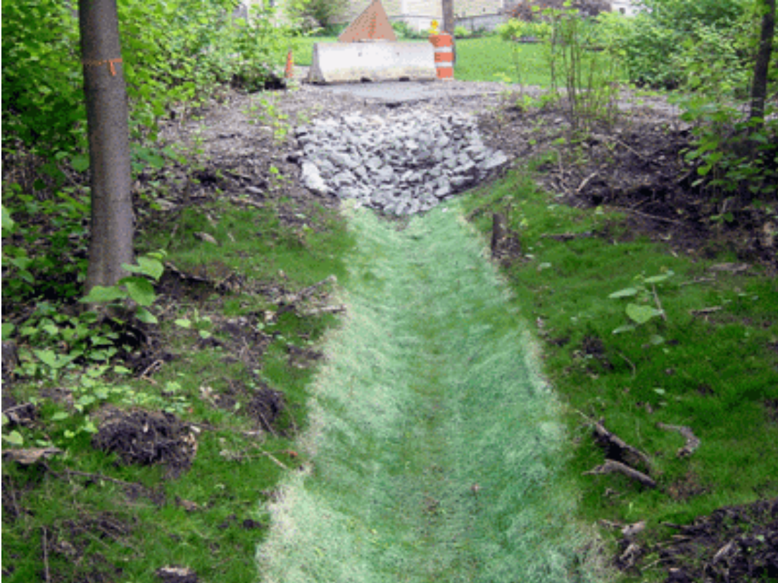
Figure C-18. Vegetated swale with potential for natural debris (RiverSides 2006).
