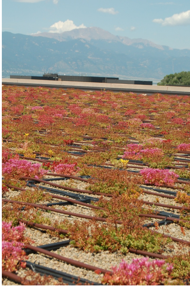
Figure C-25. Green roof atop 21st Space Wing Headquarters Building at Peterson Air Force Base, CO (photo by Thea Skinner).
