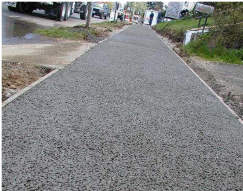
Figure C-45. Pervious concrete walkway (NRMCA).
