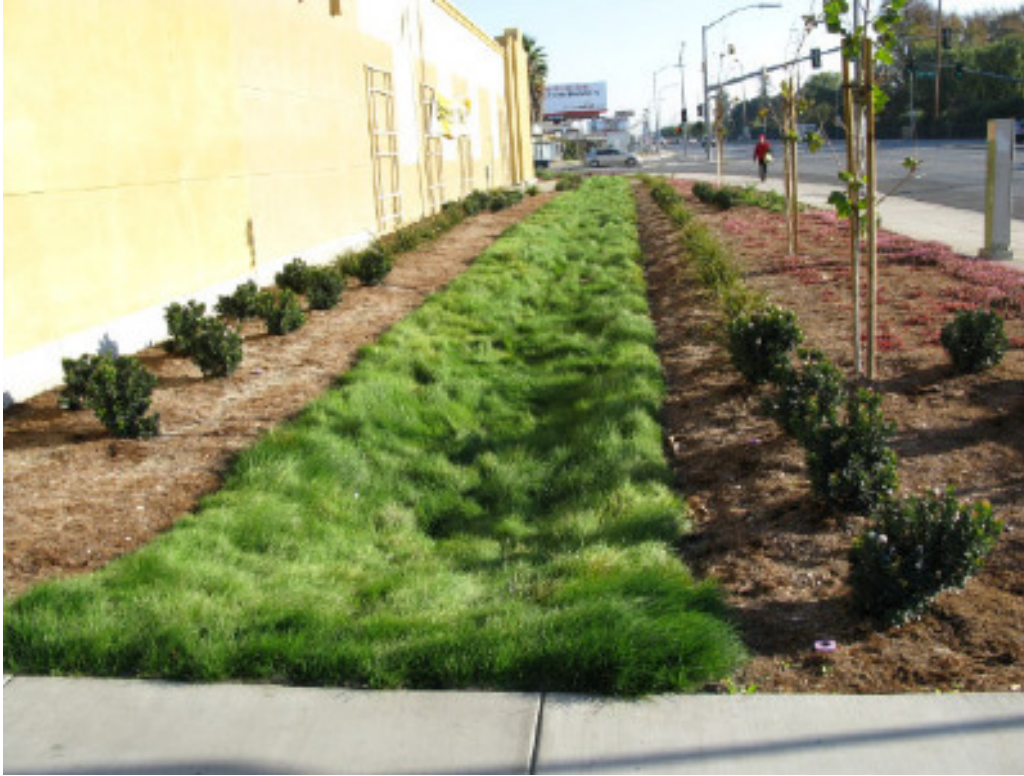
Figure C-12. Vegetated swale (courtesy of Mission Engineers, Inc. of Santa Clara, CA).
