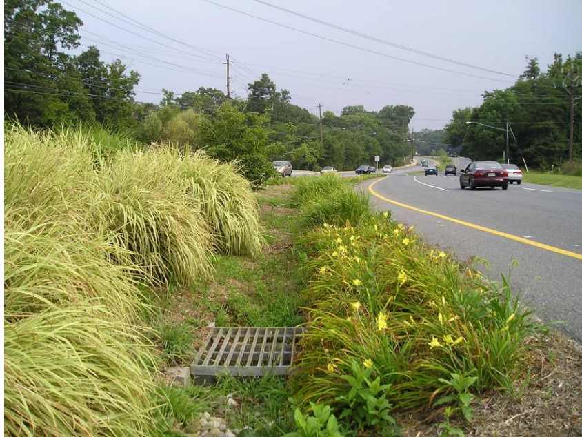
Figure C-10. Bioretention cell in Adelphi Road median, Adelphi, MD (Low Impact Development Center, Inc.).
