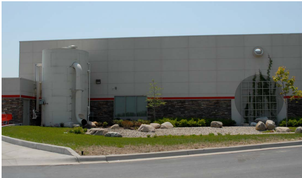
Figure C-55. Cistern at a shopping center in Allen Park, MI (courtesy of SEMCOG Regional Planning Partnership).
