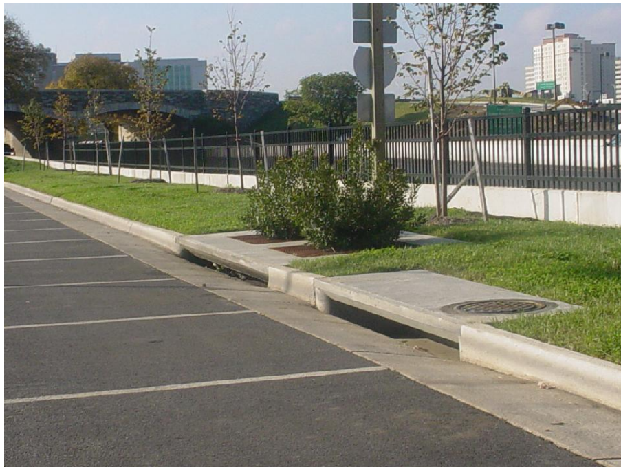
Figure C-6. Tree boxes at the Pentagon (courtesy of Low Impact Development Center, Inc.).
