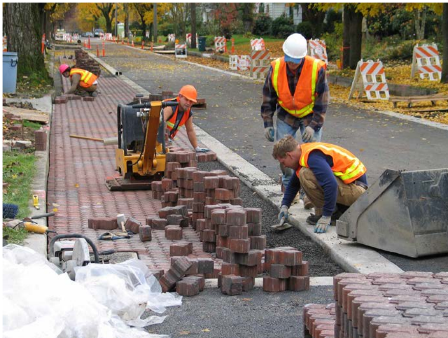
Figure C-41. Manual PICP installation (Portland Bureau of Environmental Sciences).
