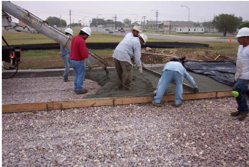
Figure C-46. Construction of permeable asphalt, Fort Hood, TX (photo by Fort Hood Environmental Support Team).
