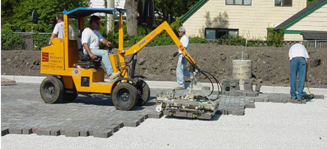
Figure C-42. Mechanical PICP installation (LPS Pavement).
