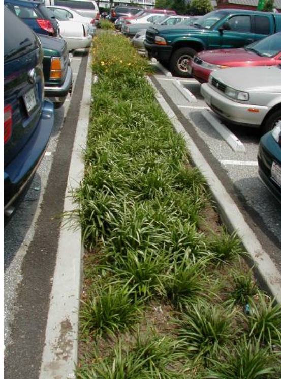
Figure C-5. Bioretention cell, Washington Navy Yard, DC (courtesy of Low Impact Development Center, Inc.).
