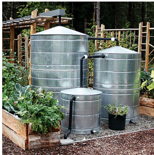
Figure C-53. Linked cisterns (photo courtesy of Sunset Publishing Corporation).
