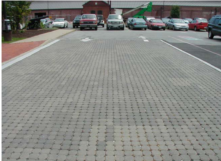
Figure C-43. Navy Yard parking lot PICP retrofit (Low Impact Development Center, Inc.).
