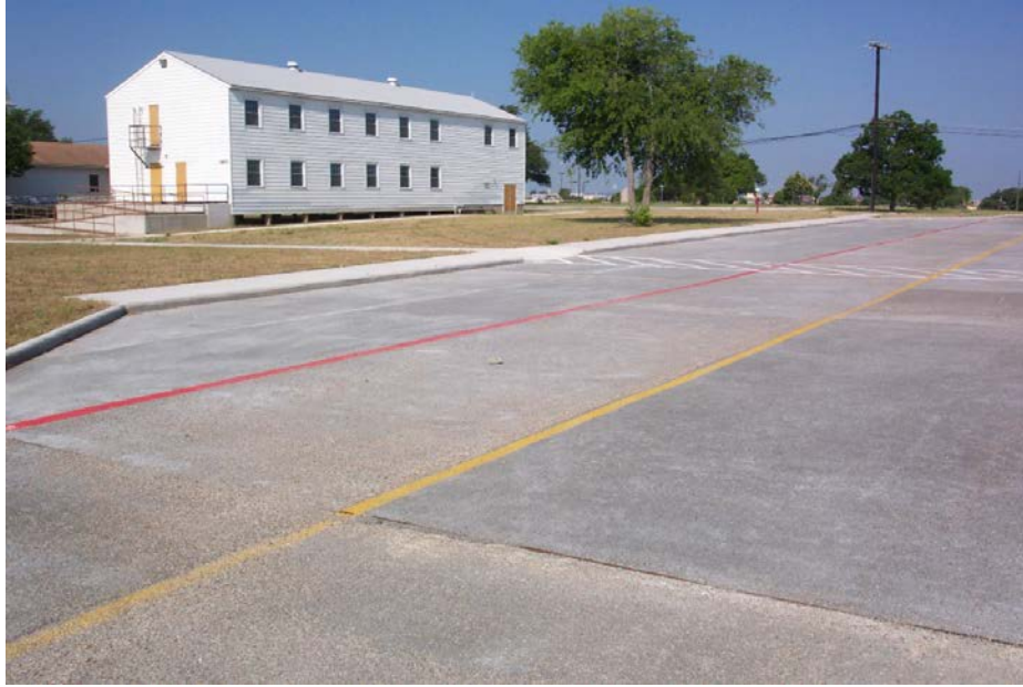
Figure C-48. Permeable asphalt at Fort Hood, Texas (photo by Fort Hood Environmental Support Team).
