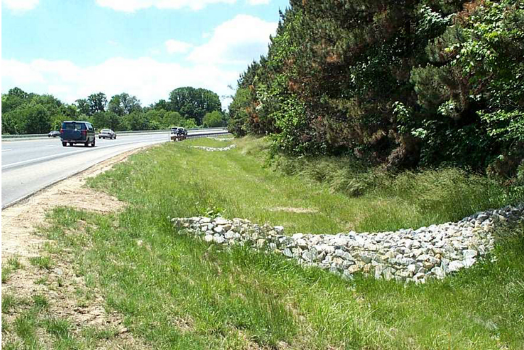
Figure C-11. Grassed swale with a check dam (photo by Delaware Department of Transportation).
