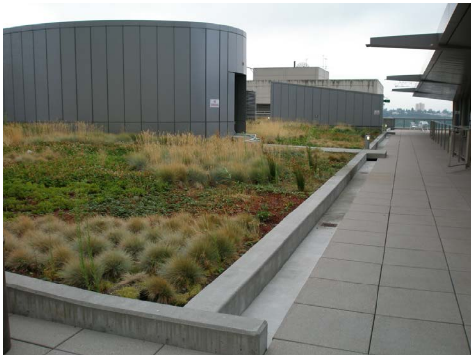
Figure C-27. Green roof on Seattle City Hall (courtesy of SvR Design Company, Seattle, WA).
