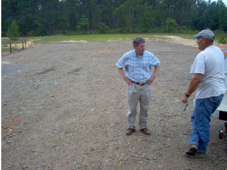
Figure A-14. Concrete from lead-based painted building was recycled as pavement base at Fort Jackson.
