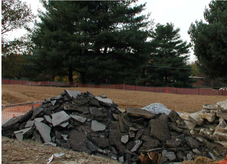
Figure A-19. Asphalt paving segregated for recycling at Andrews AFB.
