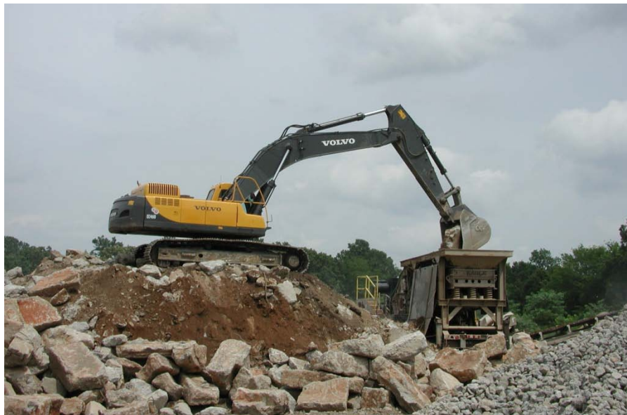
Figure A-20. Fort Campbell's concrete recycling operation.
