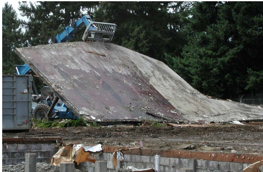
Figure A-32. Inverting a barracks floor deck for "upside-down" disassembly at Fort Lewis.
