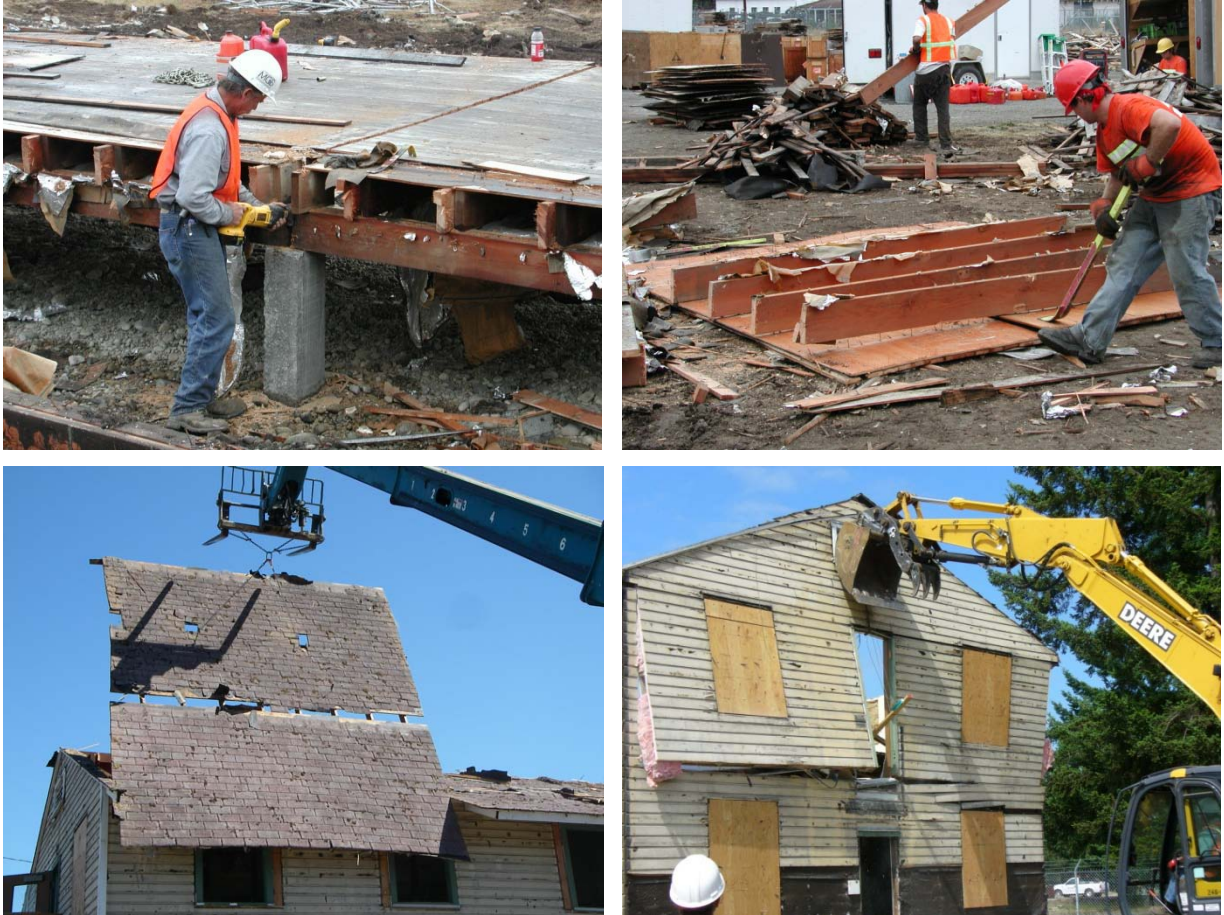
Figure A-31. Panelized deconstruction at Fort Lewis.
