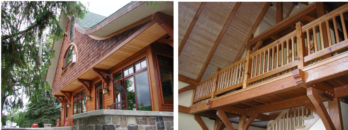
Figure A-29. Timber-frame home built with salvaged lumber near Badger Army Ammunition Plant.
