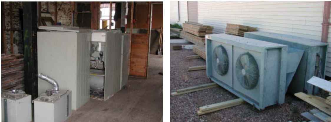
Figure A-5. Mechanical equipment recovered for reuse from buildings at Fort Campbell and Fort Carson.
