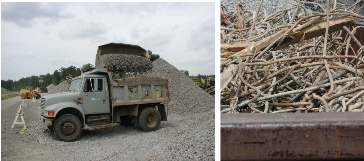
Figure A-23. Recycled concrete aggregate ready for use (left) and recyclable steel reinforcing (right) at Fort Campbell.
