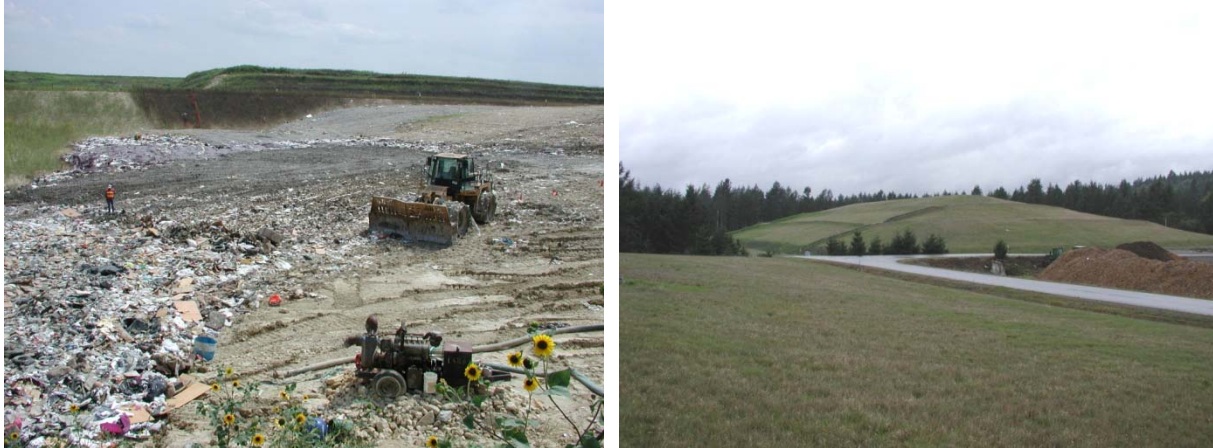
Figure A-1. Active construction and demolition landfill cell at Fort Hood (left) and closed landfill cells at Fort Lewis (right).
