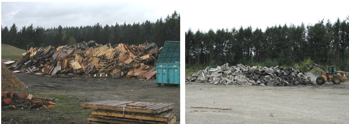
Figure A-39. Wood, concrete, and asphalt at Fort Lewis Earthworks awaiting recycling.
