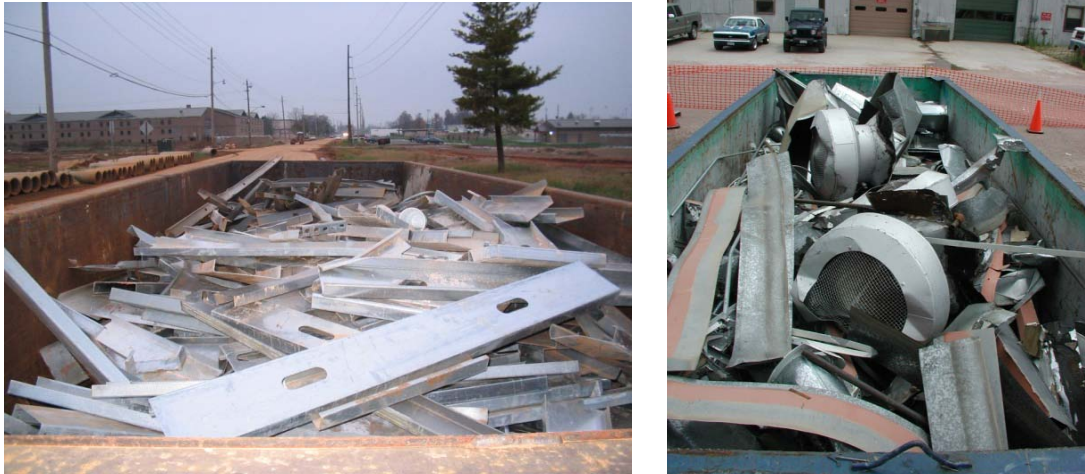
Figure A-24. Metal scrap segregated for recycling from new construction at Fort Campbell (left) and deconstruction at Fort Carson) (right). (Photo on the left by Wilmot Associates.)
