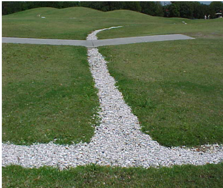
Figure H-25. French drain on a golf course (Golfmak Inc. n.d.).
