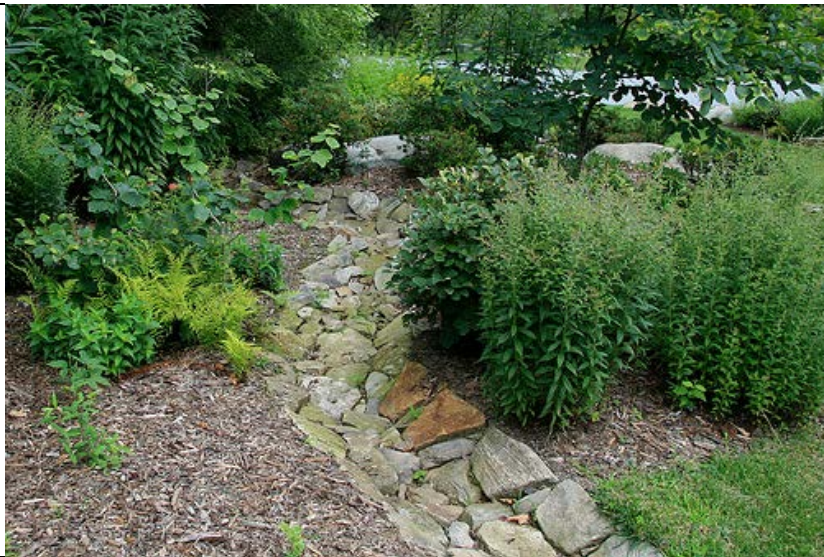
Figure H-62. Stone swale within the landscape (Roberts 2009).
