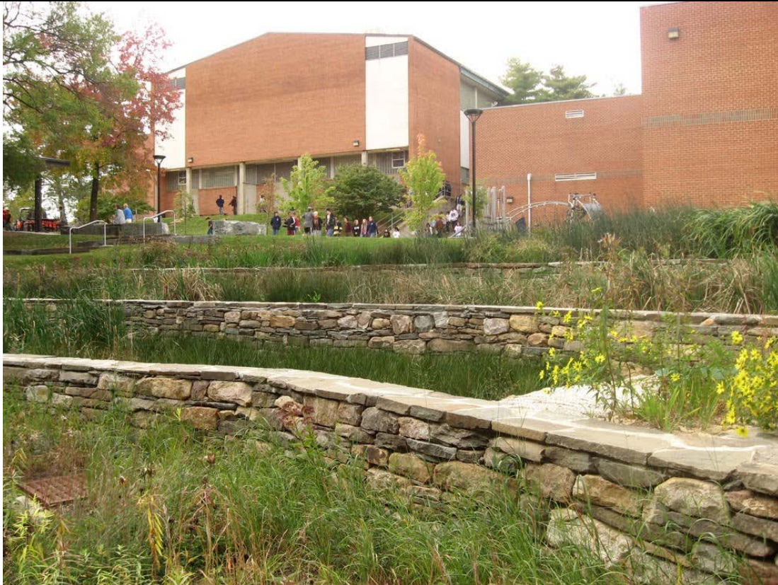
Figure H-59. Terraced blackwater treatment system at Sidwell Friends School, Washington DC (EPA 2008h).
