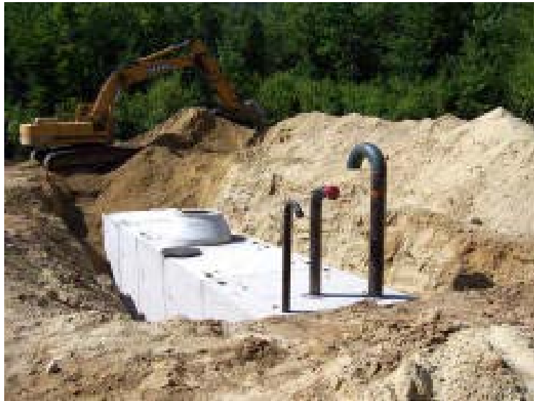
Figure H-22. Precast concrete cistern during installation (American Concrete Industries n.d).
