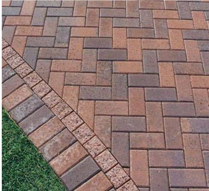
Figure H-23. Walkway made with brick pavers (Décor Guide 2011).
