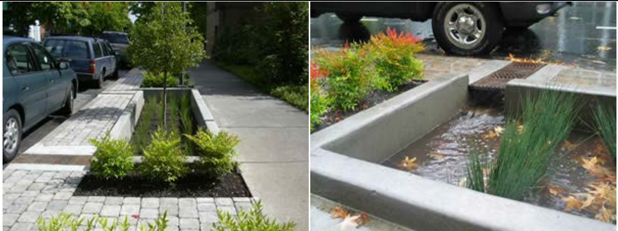
Figure H-57. Stormwater planters between the street and sidewalk. Image on right shows active collection of runoff during storm events, Portland, OR. (Portland Bureau of Environmental Services 2011).
