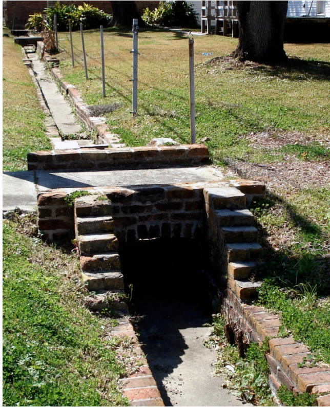
Figure I-4. Linear masonry trough at Jackson Barracks, LA (Low 2008).
