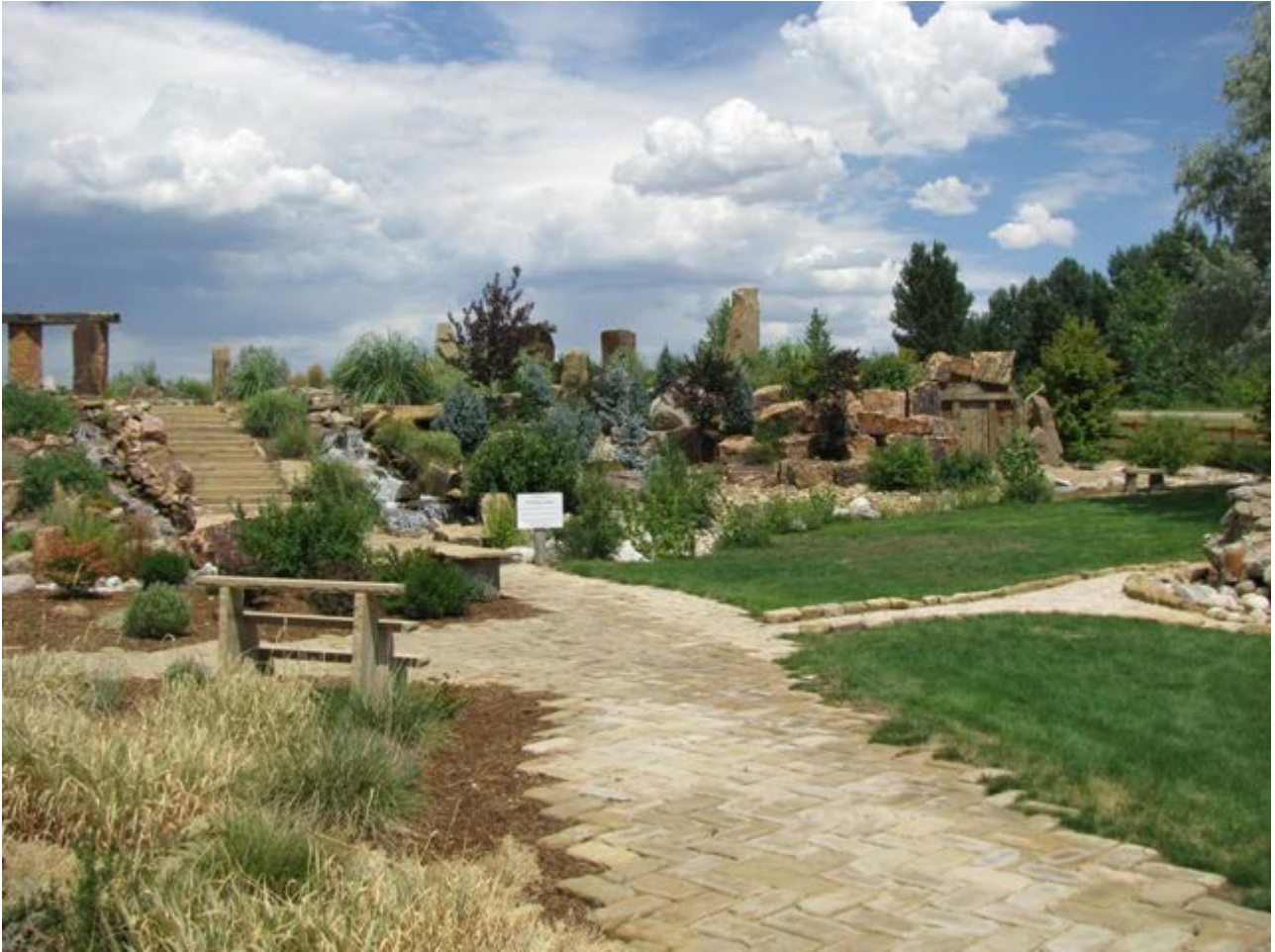
Figure H-34. Sandstone pavers used for the walkways (GroundTradesXchange 2008).
