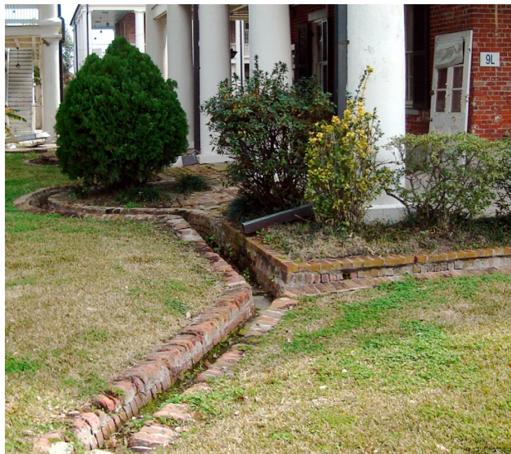
Figure I-5. Linear masonry trough at Jackson Barracks, LA (Low 2008).
