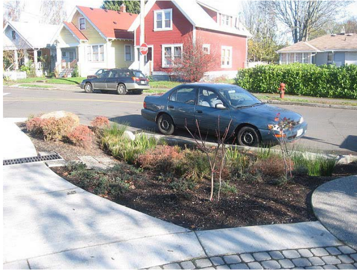
H-51. Examples of how impervious surfaces can be separated from each other with sections of pervious pavement, vegetated areas, and a drain between the sidewalk and the street (EPA 2008i).
