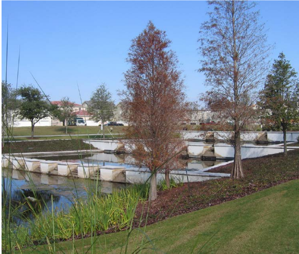
Figure H-87. An example of a slope avenue at Baldin Park, FL (Low 2008).
