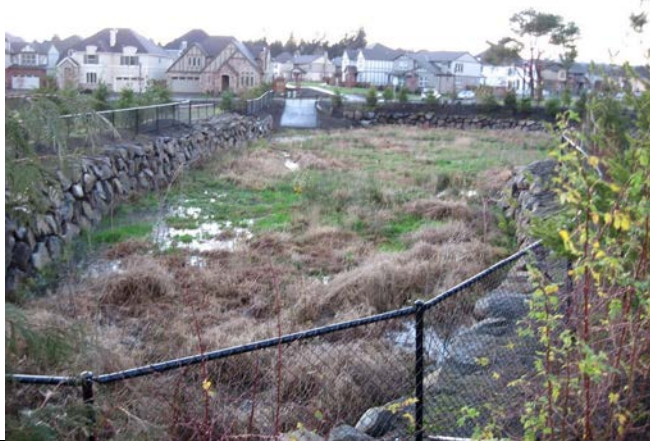
Figure H-84. Large retention basin, with vertical stone walls and protective fence to allow steeper pond edges and therefore, maximize retention volume capacity (EPA 2007).
