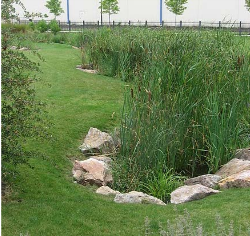
Figure H-64. Bioretention swale in Chicago (EPA 2008b).
