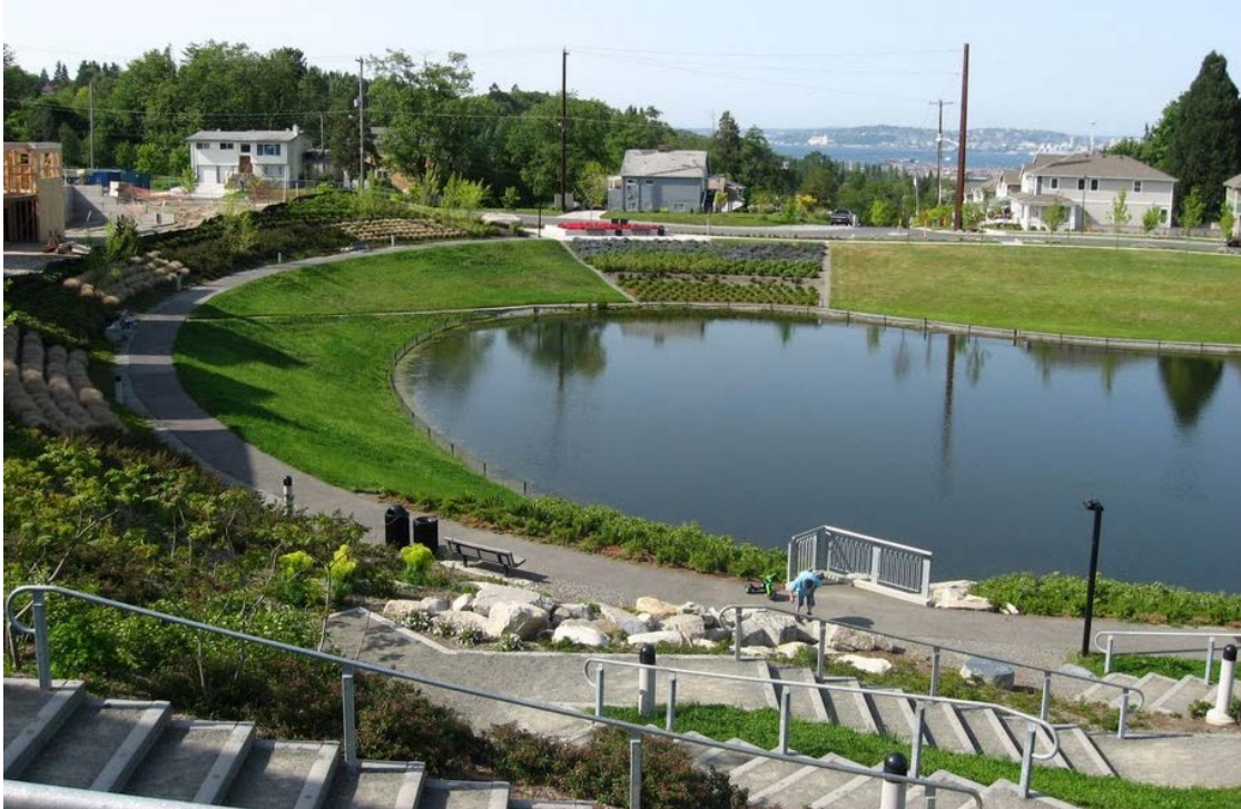
Figure H-83. An urban retention pond in Seattle, WA, includes a walking trail and overlook decks that let it double as a community amenity in addition to its role for stormwater management (EPA 2007).
