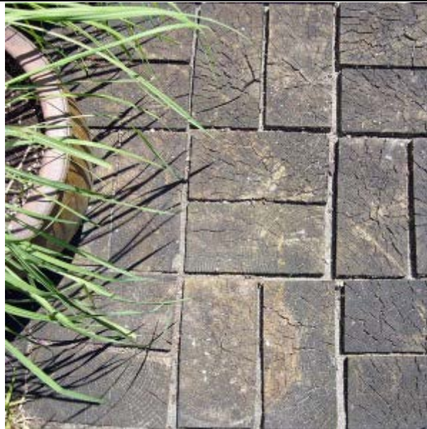
Figure H-76. Wood paving blocks (Vancouver Modern Residential Blog 2010).
