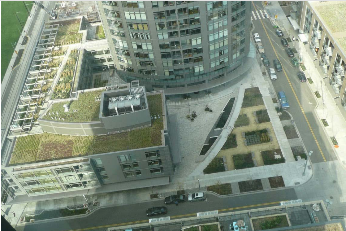
Figure H-69. Green roof in Portland, OR, with street planters below (EPA 2008c).
