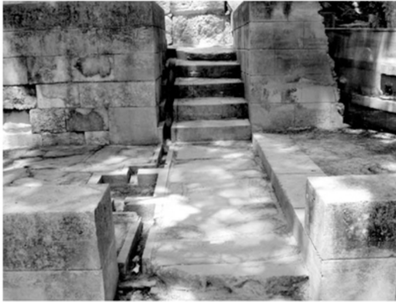
Figure I-1. Part of restored stairway with parabolic runnels in Knossos Palace, Crete (Angelakis et al. 2005).
