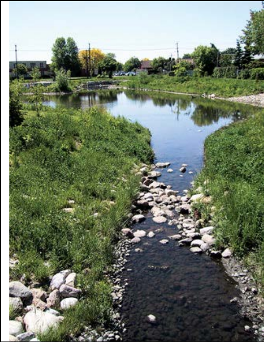
Figure H-85. Terraview Park and Willowfield Gardens Park in Toronto, Ontario, utilize the flow of Massey Creek within created and linked pools of water to collect and filter area stormwater (Anderson 2010).
