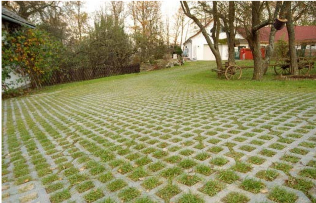
Figure H-35. Turf block used in an entryway drive and parking lot (Alpine Limited n.d.).
