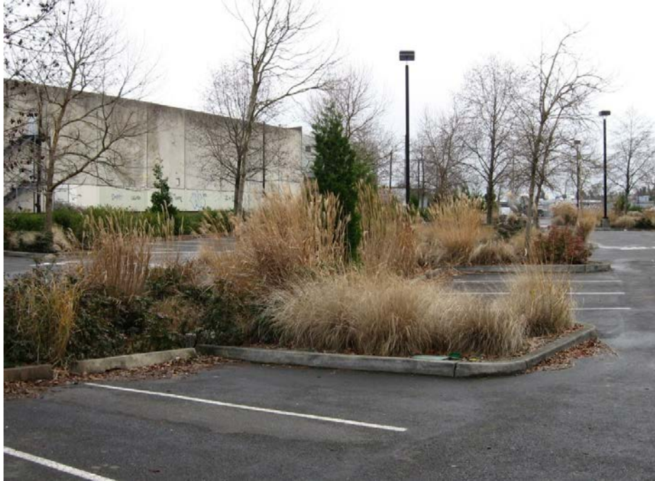
Figure H-73. Vegetative swale utilized in a parking lot in Portland, OR (EPA 2007b).
