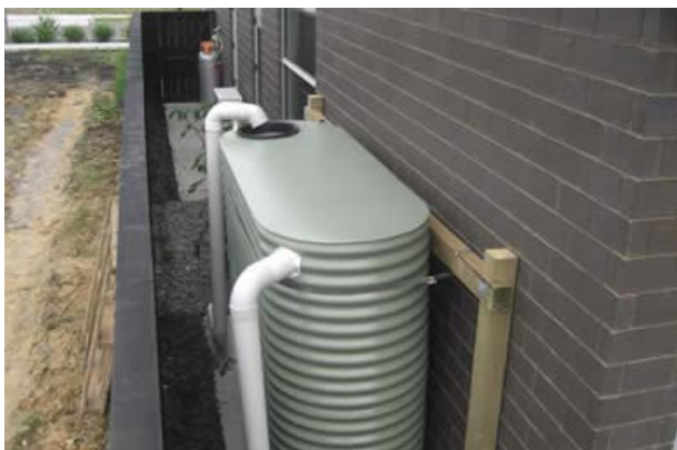
Figure H-17. Metal cisterns can also be installed above ground, either round (not shown) or in slimline dimensions in order to be less invasive (Tanks Alot n.d.)
