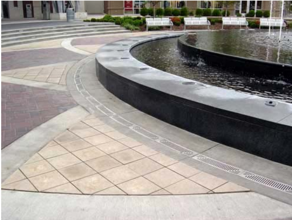
Figure H-36. Trench drain along this fountain captures stormwater and fountain overflow to be reused in the civic water feature (Novak 2008).
