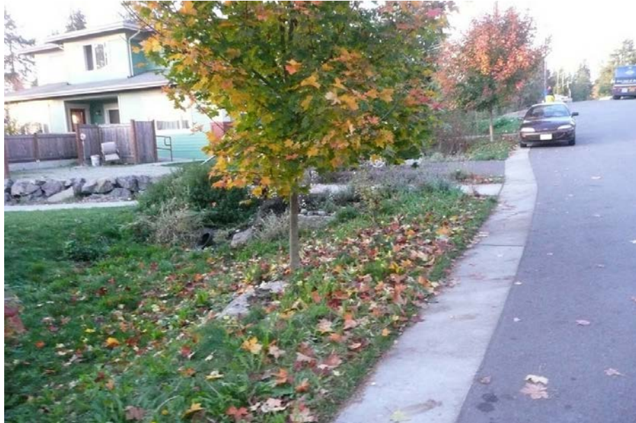
Figure H-37. Vegetated swale runs the length of the street (EPA, 2008k).
