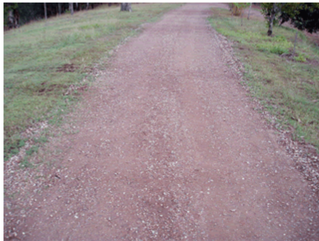
Figure H-71. Stabilized road surface made from compacted earth (Total Earthworks and Environmental Services n.d.).
