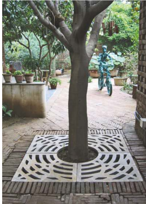
Figure H-39. Grated tree well in an urban area (KK Manhole & Gratings Co. Pvt. Ltd n.d.).
