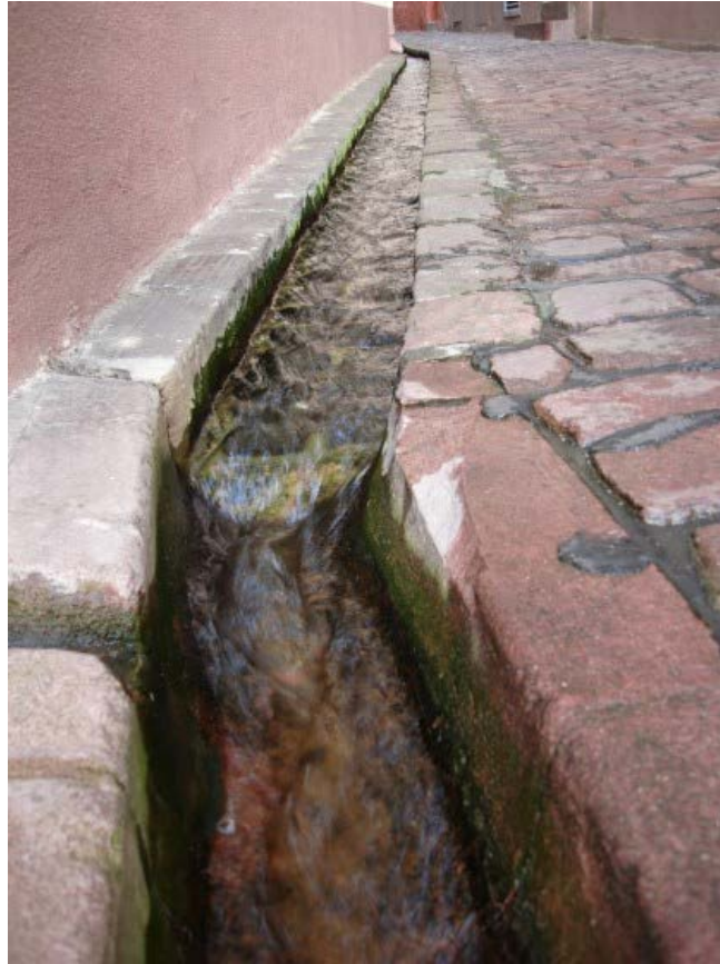
Figure H-32. Masonry trough, Freiburg, Germany; a thirteenth-century stormwater channel system forms part of the Dreisam river (Lisa Town 2009).
