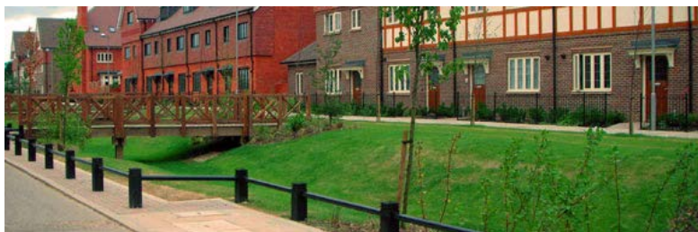
Figure H-63. This swale system in Upton, Northampton, England, implements SUDS to provide flood protection and additional recreation area (Sustainable cities™ n.d.).
