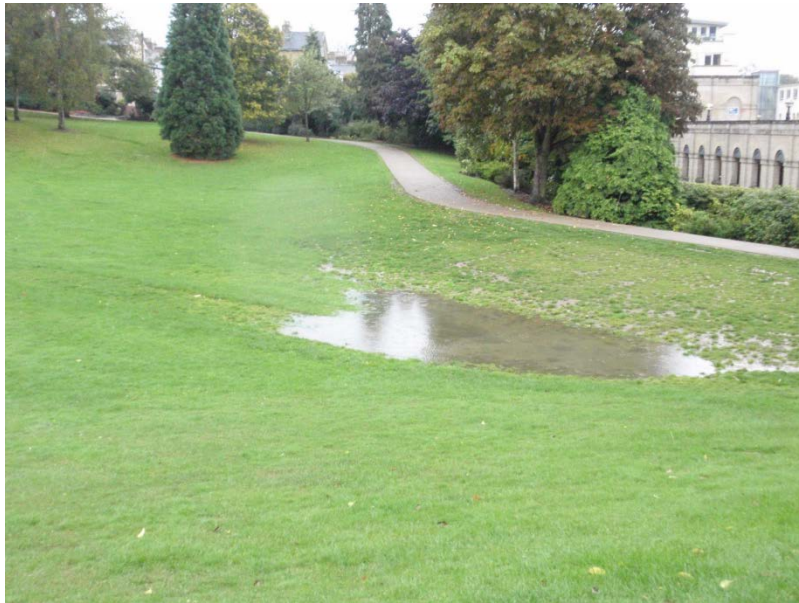
Figure H-56. Depression in grassy area holding stormwater (Isabel 2010).
