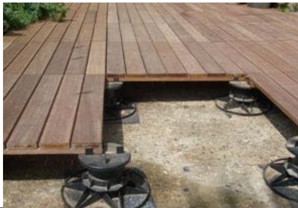
Figure H-79. Another option for a walkway that uses timber paving tiles (Wallbarn 2011).
