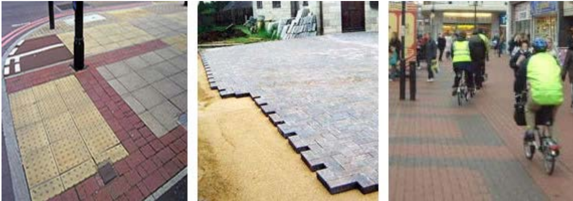
Figure H-41. Various examples of asphalt block used as pavers (Top Asphalt Limited n.d.).
