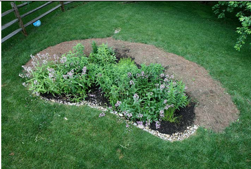
Figure H-55. A rain garden with an underdrain (see outlet in gravel just above garden berm left of center; Wilson 2009).
