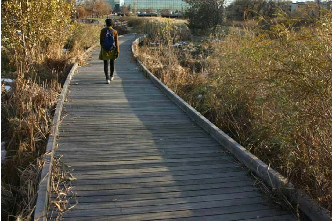
Figure H-77. Planked walkway traversing a wetland, Denver, CO (American Trails 2009).
