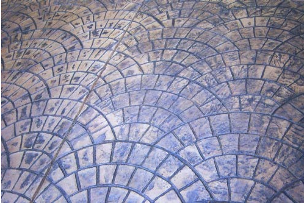
Figure H-42. Cast-in-place concrete, stamped with the block pattern, then colored and finished to achieve desired look (Professional Concrete 2010).
