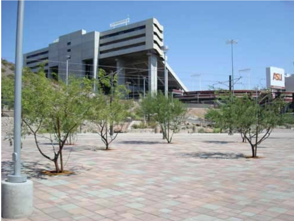
Figure H-31. Tree grove integrated into paved area creates a pervious surface parking lot without curbs (Novak 2008).
