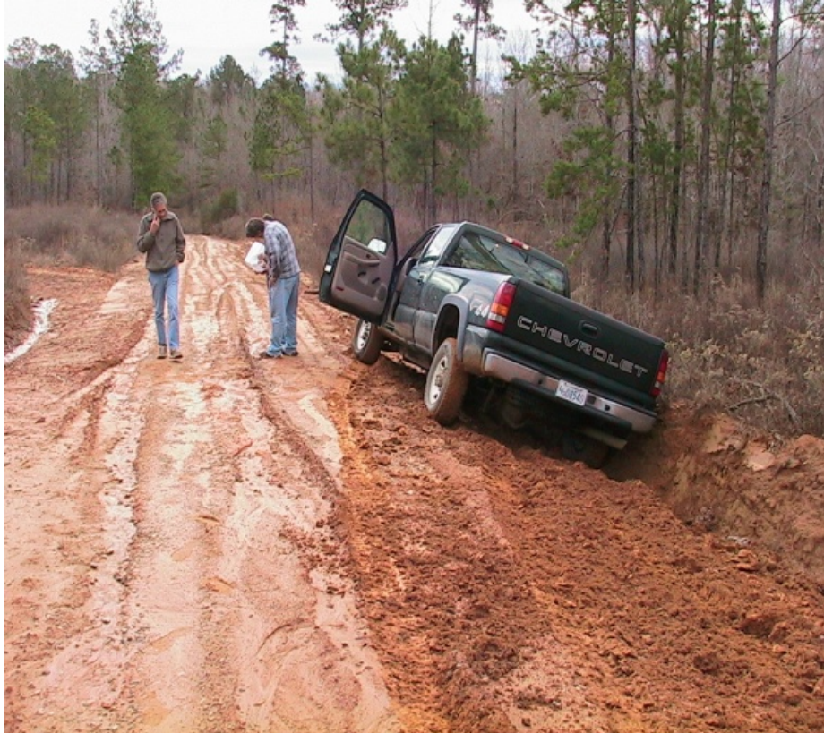
Figure A-7. An example of issues with water on unsurfaced roadways as a road inspection crew slipped off the roadway under wet clay conditions.
