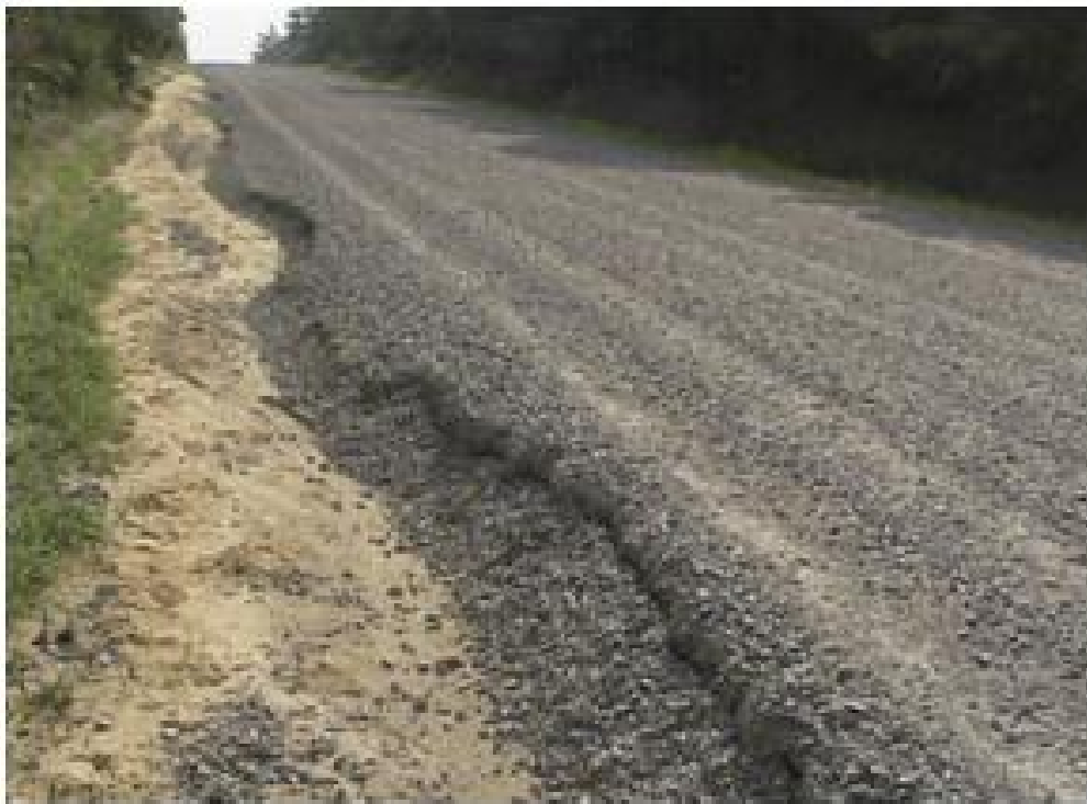
Figure A-4. Lack of timely repair to an eroded shoulder can result in expensive maintenance.
