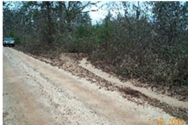
Figure A-15. Turnout to divert water away from the road.
