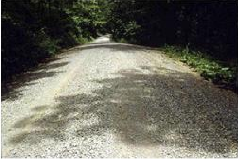
Figure A-9. A proper road crown is the first line of defense against water.
