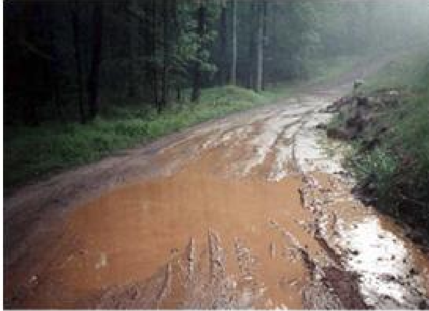
Figure A-6. A low-lying area in a road with poor drainage ditches results in a flooded road.
