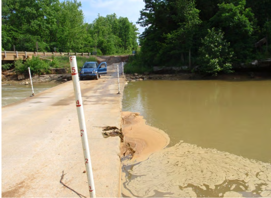
Figure B-2. Markers along edge of LWC with depth marks (photo by Scot Serafin, Fort Knox, KY).
