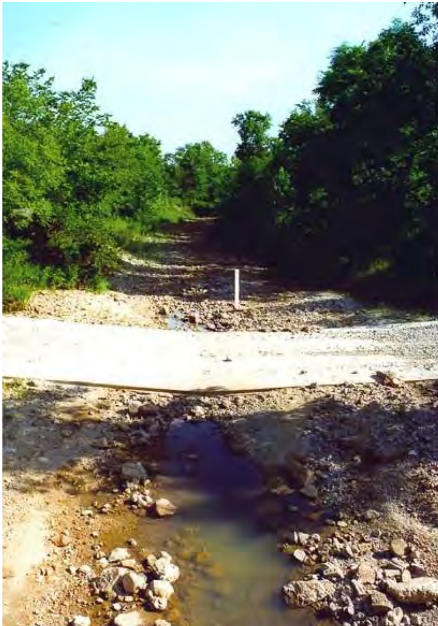
Figure C-6. Cement slab LWC (photo by Joe Proffitt, Fort Leonard Wood, MO) .
