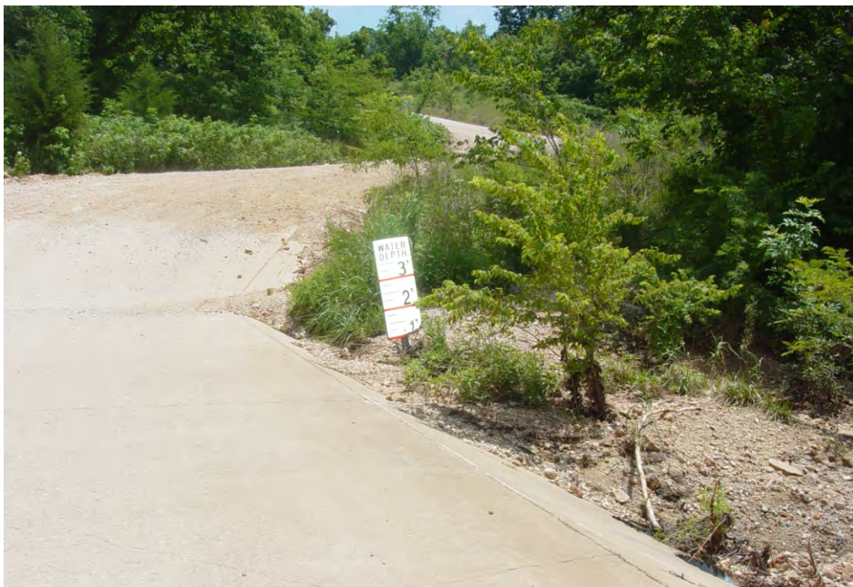
Figure B-3. High-water depth gauge (photo by Joe Proffitt, Fort Leonard Wood, MO).
