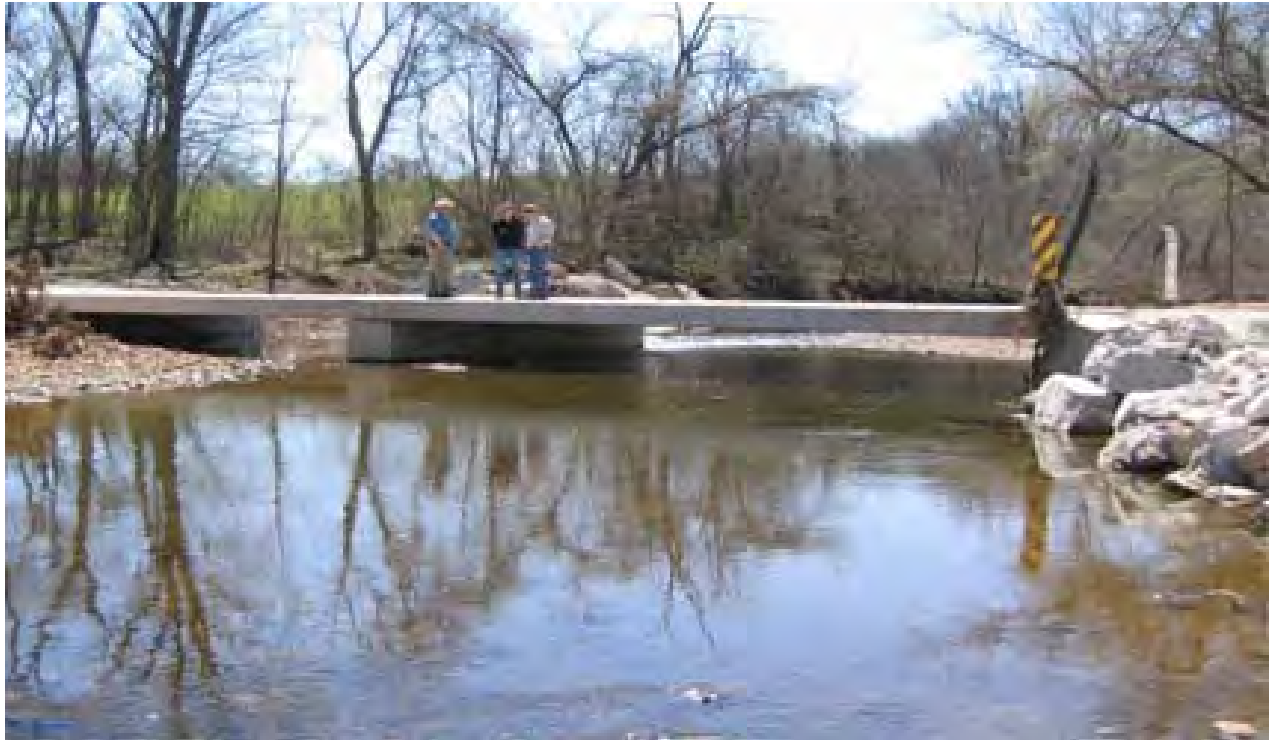
Figure A-3. Low-water bridge (photo courtesy of U.S. Fish and Wildlife Service, MO).
