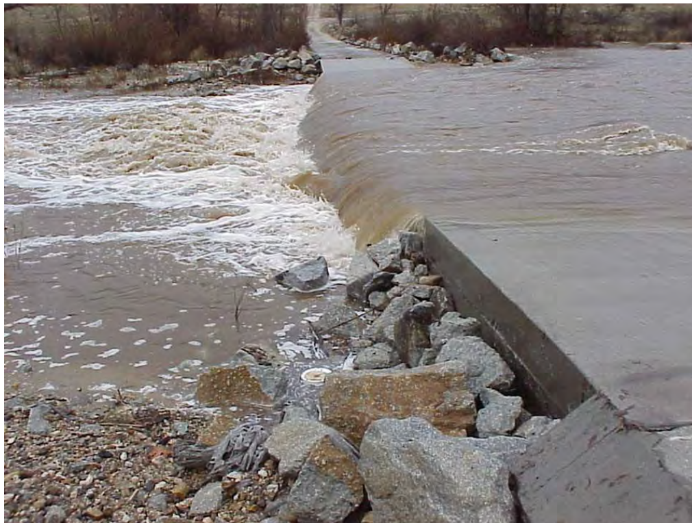
Figure C-2. Narrowed stream where scouring is occurring (photo by Art Hazebrook, Fort Hunter Liggett, CA).
