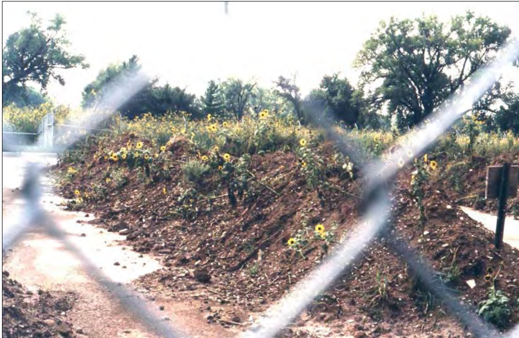
Figure B-11. Bioremediation pad at Fort Riley.
