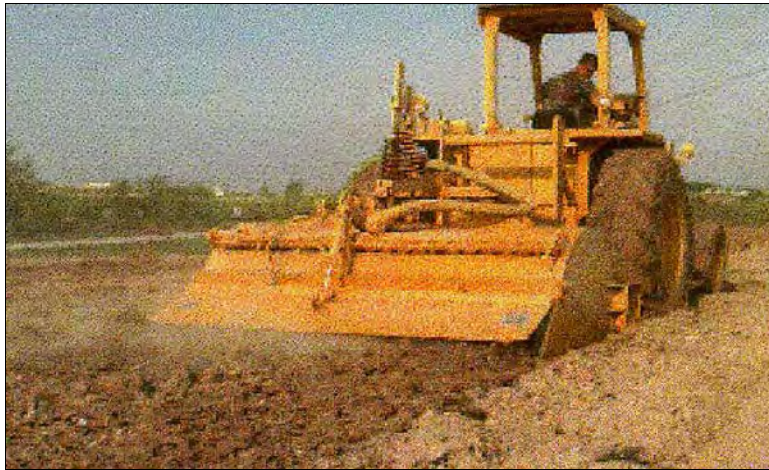
Figure B-7. Tilling operation.
