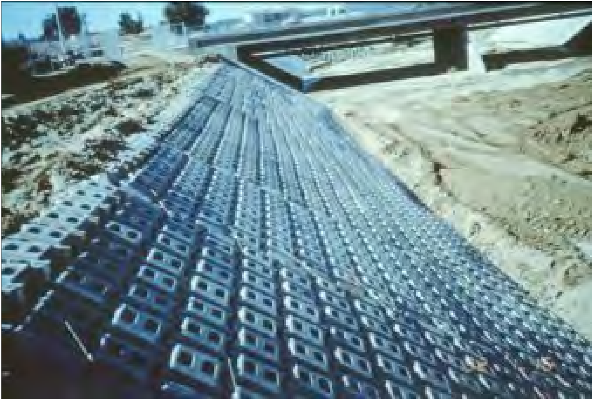
Figure A-6. ACB installed on open channel embankment.
