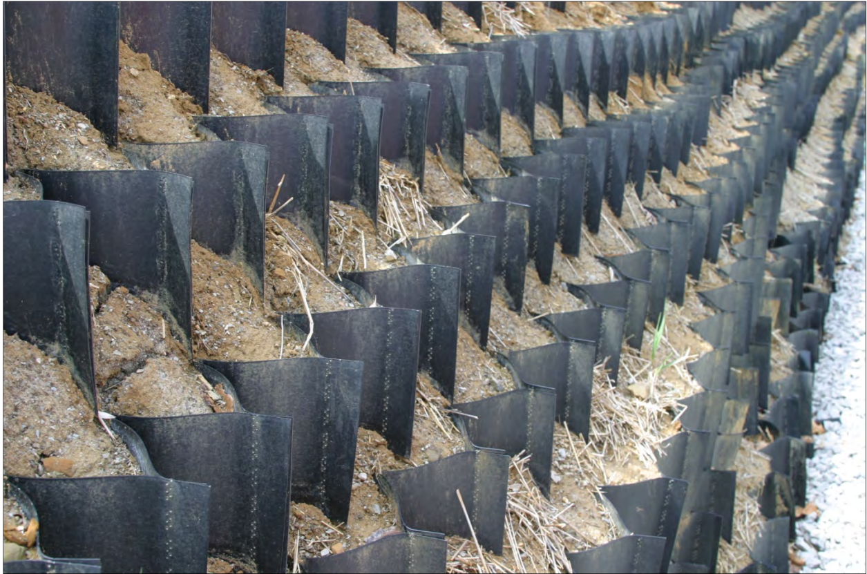
Figure A-3. Geocells installed as a retaining wall.
