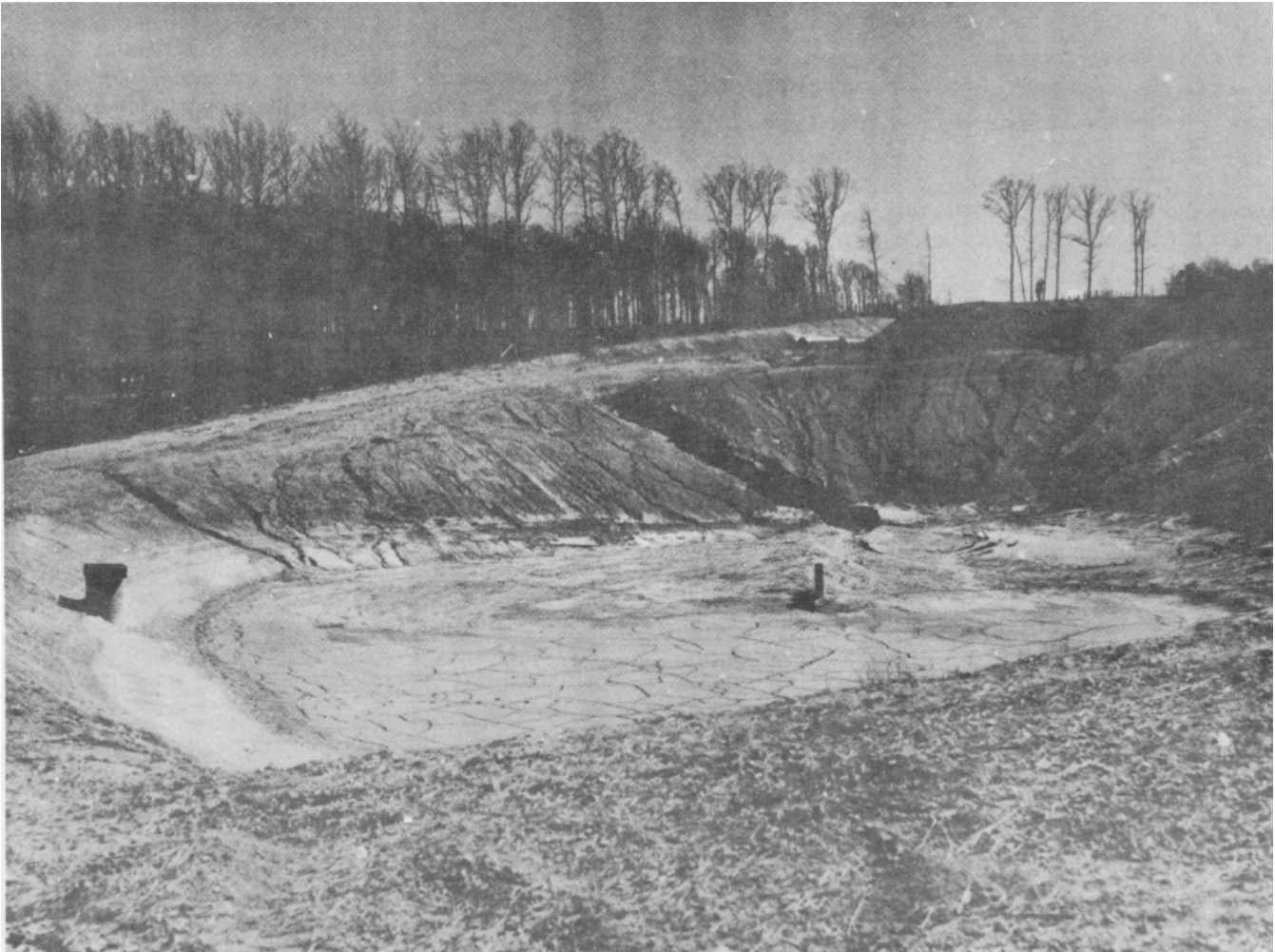
Figure 7-1. Sediment basin on a construction site.
