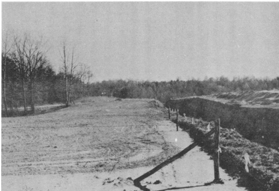
Figure 15-6. Sanitary landfill with topsoil replaced and revegetated as fill is completed.
