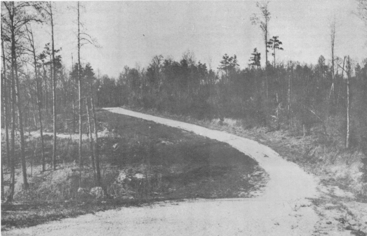
Figure 10-12. Vegetated firebreak with rock-surfaced patrol road
