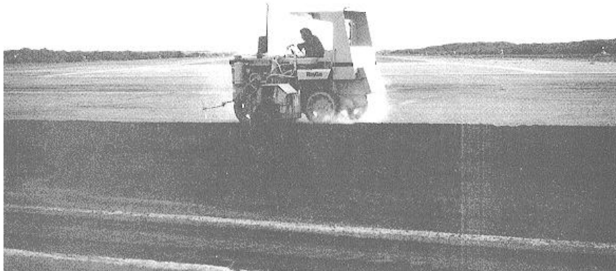
Figure 3-34. Self-propelled pavement milling machine.
