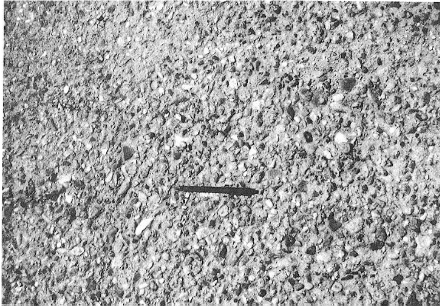
Figure 4-15. Polished aggregate.
