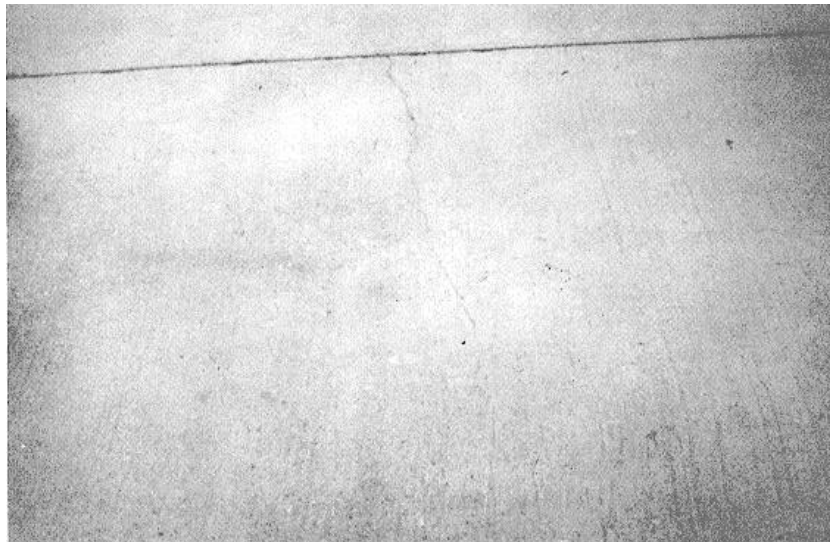
Figure 4-22. Shrinkage crack.
