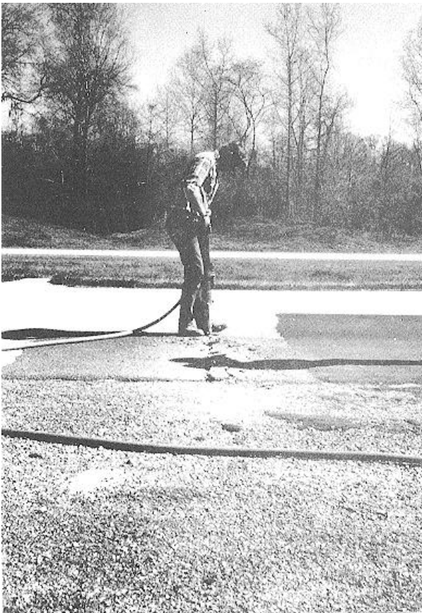
Figure 3-28. Removing damaged pavement with a jackhammer.
