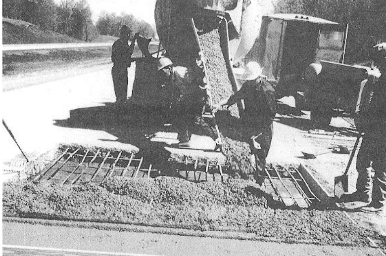
Figure 4-40. Placing concrete in patch area.
