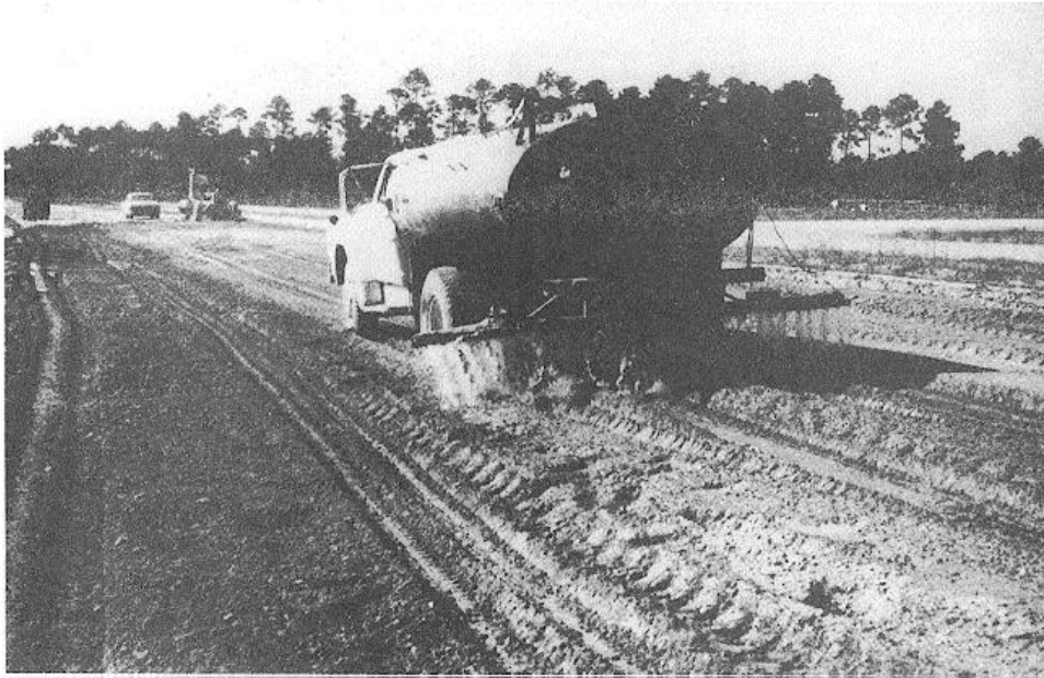
Figure 5-14. Adding water to the soil.
