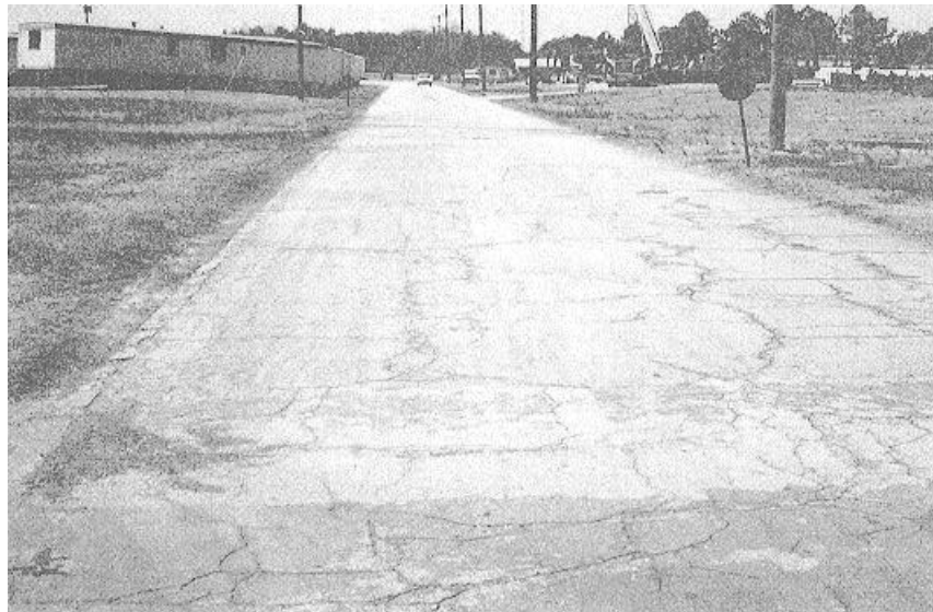
Figure 3-3. Block cracking.
