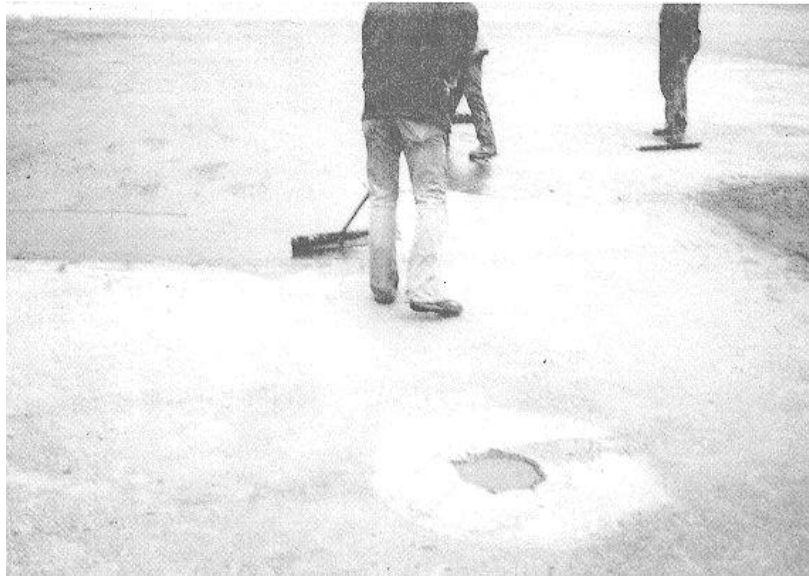
Figure 3-25. Applying a seal coat with squeegees.
