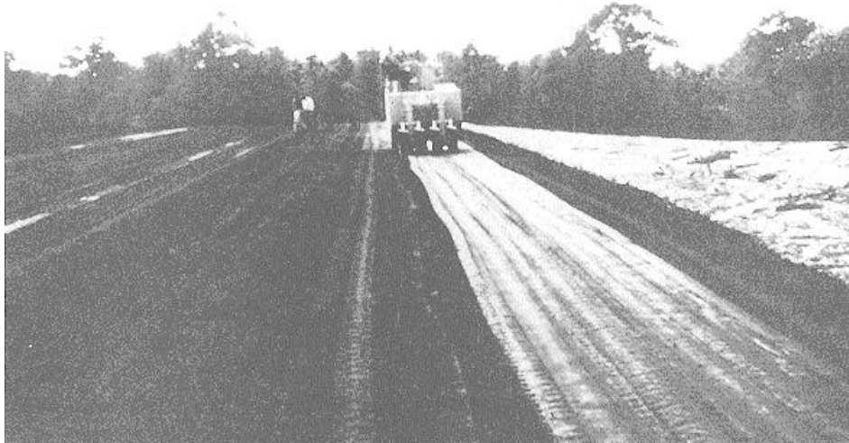
Figure 5-15. Finish rolling with a rubber-tired roller.
