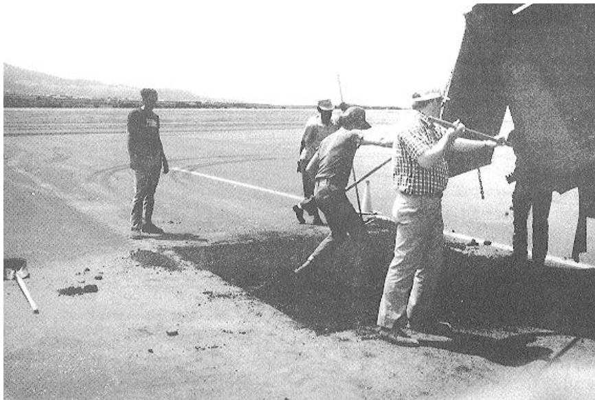
Figure 3-49. Placing asphalt mix in patch.
