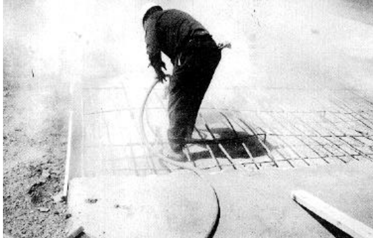
Figure 4-38. Cleaning patch area with compressed air.
