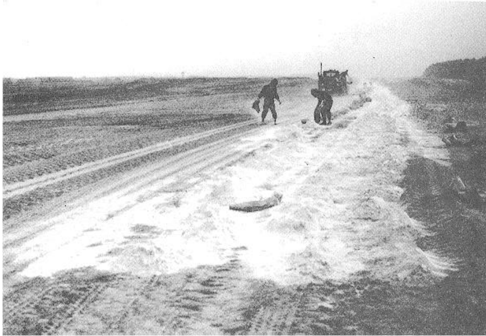
Figure 5-10. Hand spreading bags of cement.
