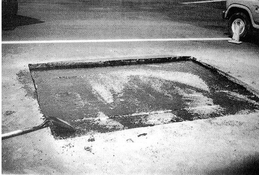
Figure 3-48. Hole to be patched with tack applied
