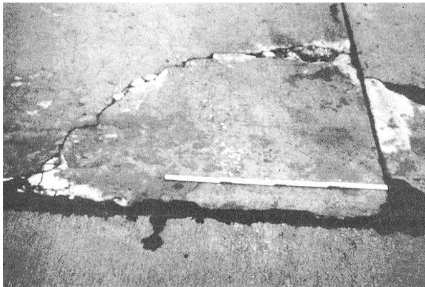
Figure 4-6. Corner break.
