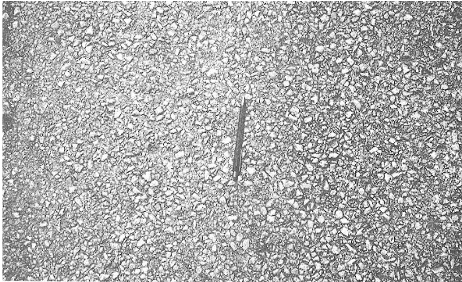
Figure 3-12. Polished aggregate.
