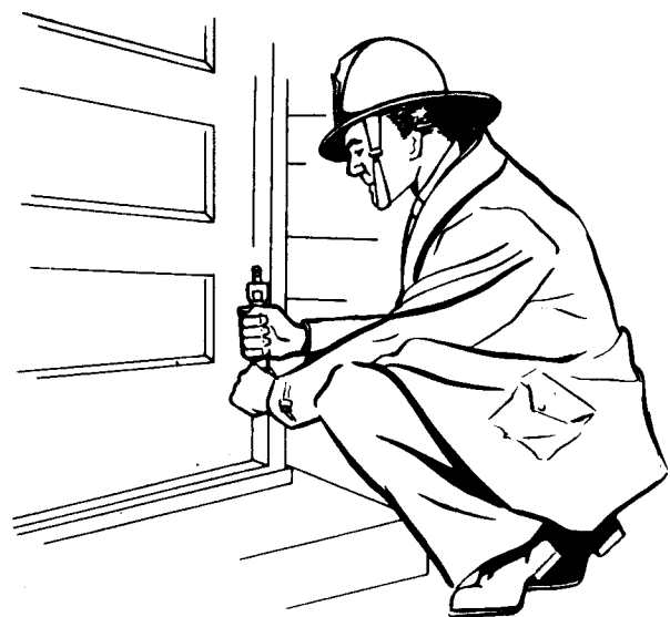
Figure 4-51. Removing the hinge pins.
