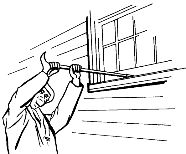
Figure 4-59. Opening check-rail windows.
