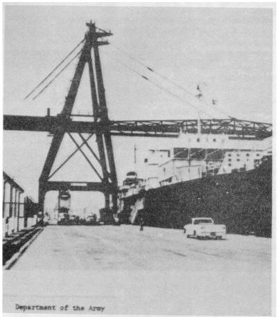
Figure 12-3. Typical rail-mounted gantry crane.
