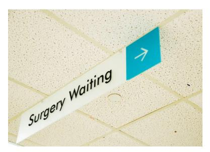
Absorptive ceiling tiles reduce the volume of sounds reflected off their surfaces, the length of time they last, and distance they travel. Photo © iStockphoto.com/sshepard
