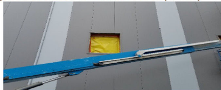
Image 11-4 IMP Louver Termination Sealed
