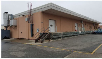
Image 10-2. Building 4 Shop Photo
