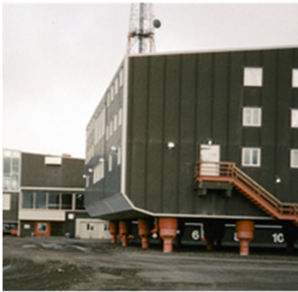
Figure 5-5. Examples of elevated structures on permafrost. Upper photo: An image of downtown Utqiagvik, Alaska where single-story and multi-story buildings, as well as all utilidors, are constructed above ground. Lower left: a large facility at Prudhoe Bay, Alaska. Lower right: a single-story structure at Thule, Greenland. Photos by Kevin Bjella, CRREL.
