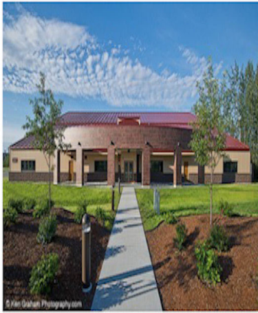
Image 6-1. Building 10 IMP Wall and Roof
