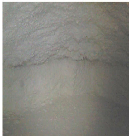
Image 8-4. Building 2 Roof to Wall Joint Dig.
