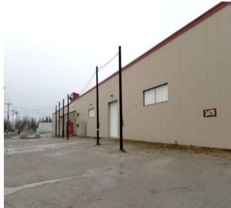
Image 9-2. Building 3 Storage Facility and Shop
