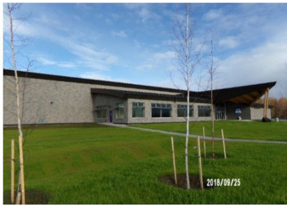
Image 5-1. Bldg. 27 CMU Wall & Metal Roof
