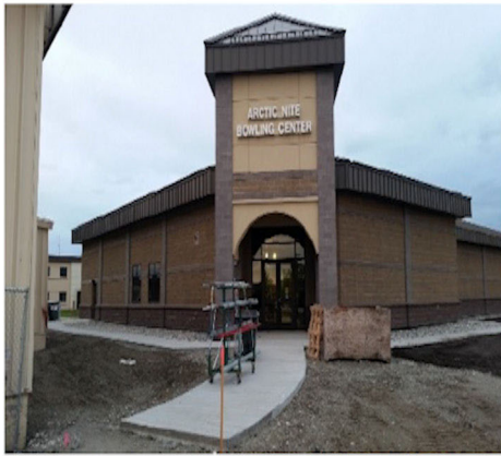
Image 7-1. Building 23 CMU Wall & Attic Ceiling
