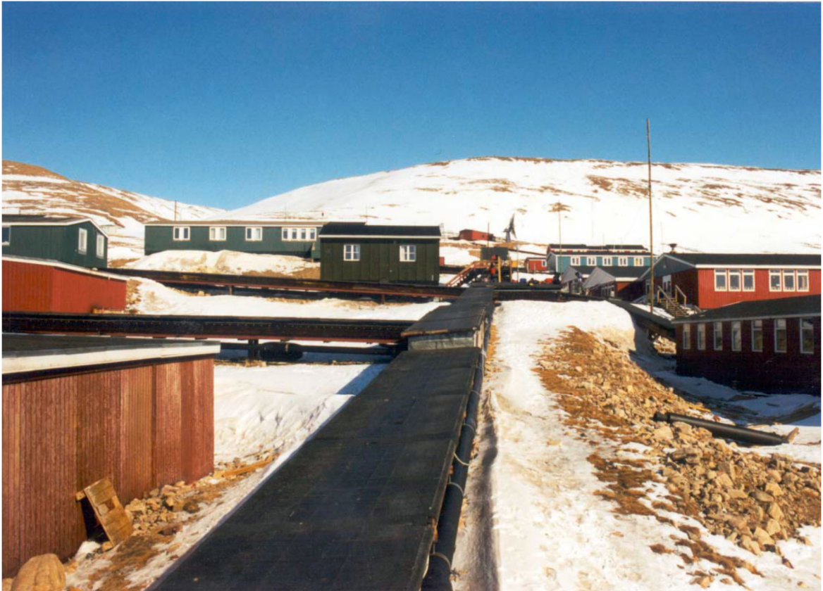
Figure 7-13. Above-ground supply infrastructure. Source: Ramboll A/S.
