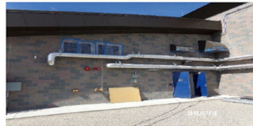
Image 11-5 CMU Louver Wall Termination Sealed
