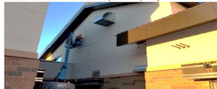
Image 11-3 EIFS Louver Wall Termination Sealed (Winter)
