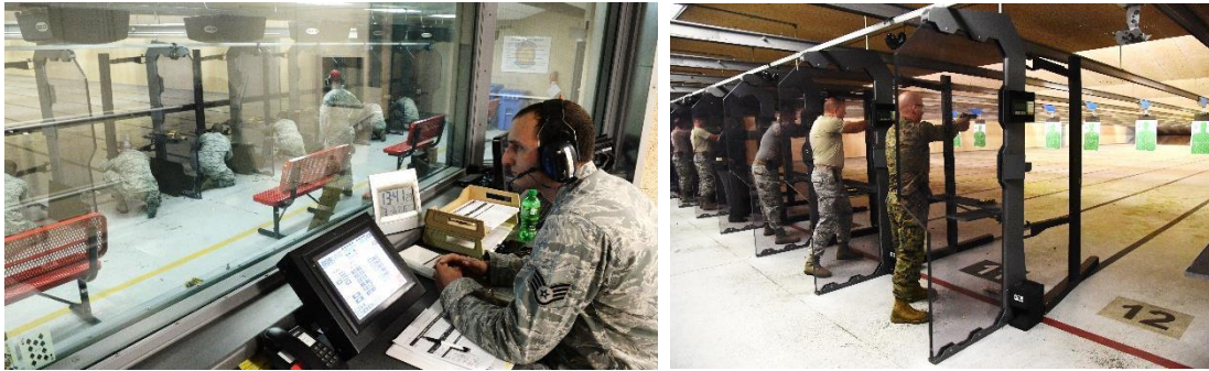
3 Figure 6-4: CATCODE 171-475, Indoor Small Arms Range showing ventilation control 4 panel in control booth 5
