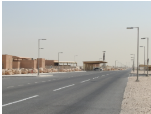
Local Street Lighting
