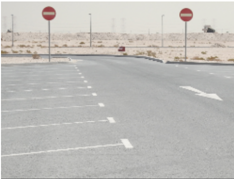
Parking Lot Paving and Striping
