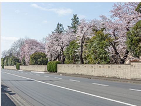
Sound Wall and Landscape Buffer
