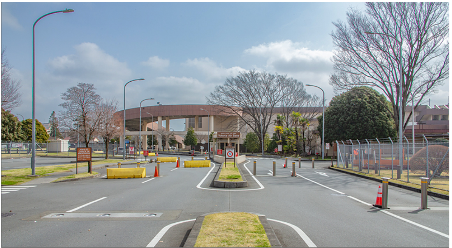
Landscaped Median and Integrated Security Elements
