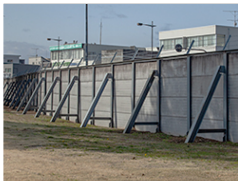
Reinforced Wall at Perimeter
