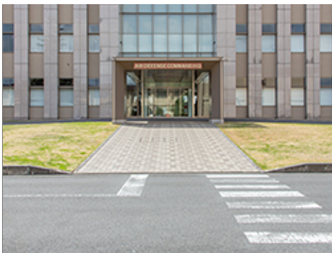
Building Entrance Plaza at Group 1
