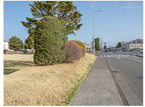
Attached Concrete Sidewalk at Street
