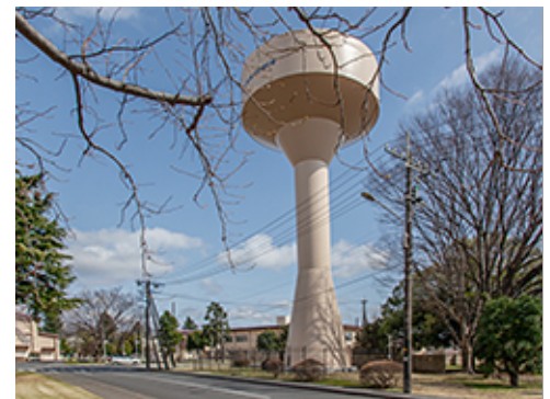
Elevated Water Storage Tank
