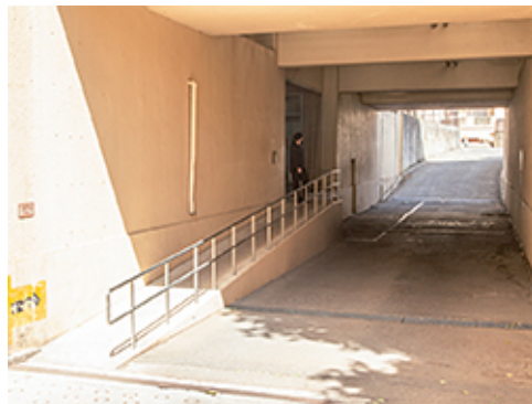
Ramp with Railing
