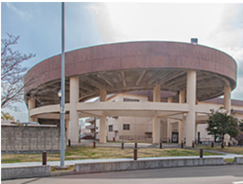
Exterior Ramp at Parking Garage
