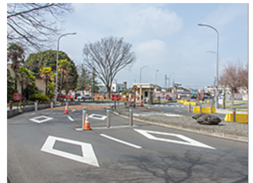
Retractable Bollards at Gate
