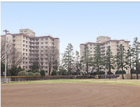
Openings and Balconies Providing Scale
