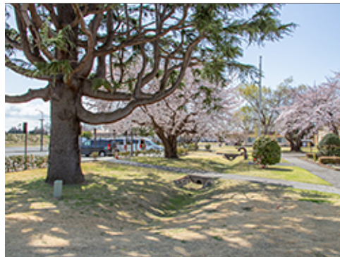
Swale with Drainage Elements
