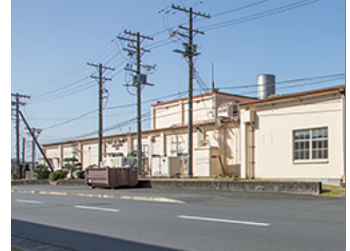
Overhead Utility Lines Adjacent to Group 3
