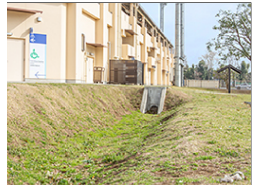
Vegetated Drainage Swale
