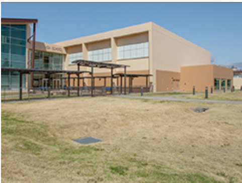
Drainage Basin with Inlets
