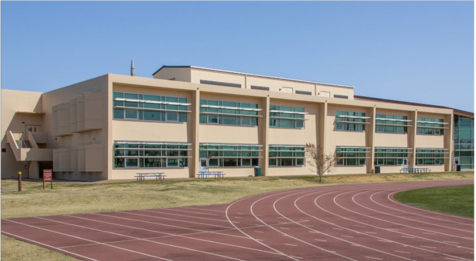
Exterior Materials and Details with Solar Shading Devices on South-Facing Facade
