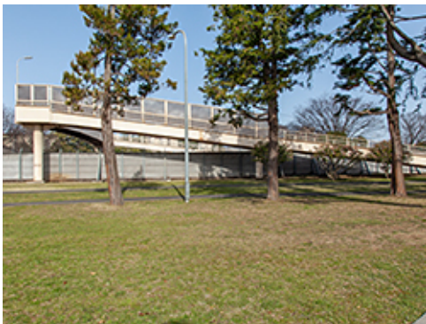
Ramp System over Street
