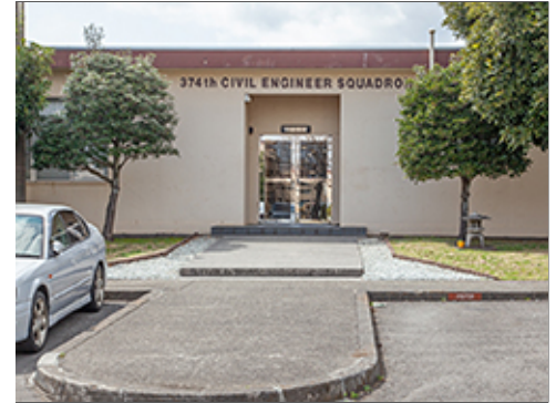
Concrete Paving at Group 2
