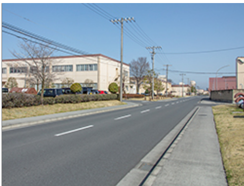
Overhead Utility Service near Group 3
