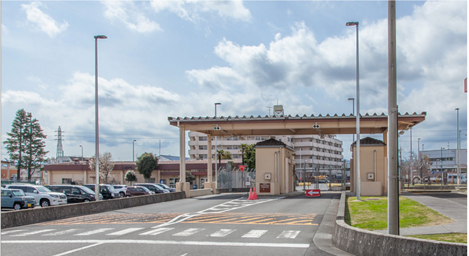
Standard Street Lighting
