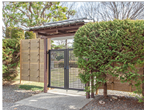
Fencing and Gate
