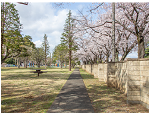
Masonry Wall at Park Boundary
