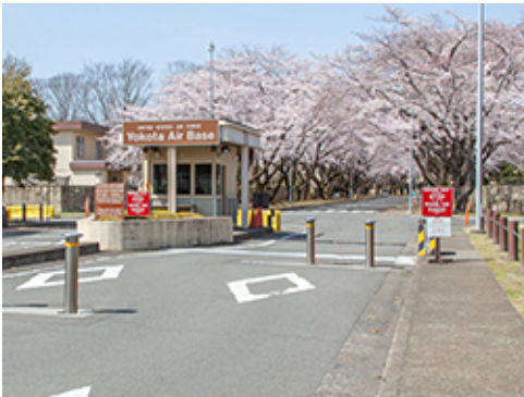
Group 1 Gate at McGuire Avenue
