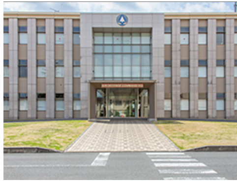
Alignment with Crosswalk
