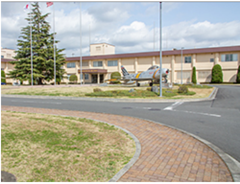
Colored Concrete Paving at Group 1
