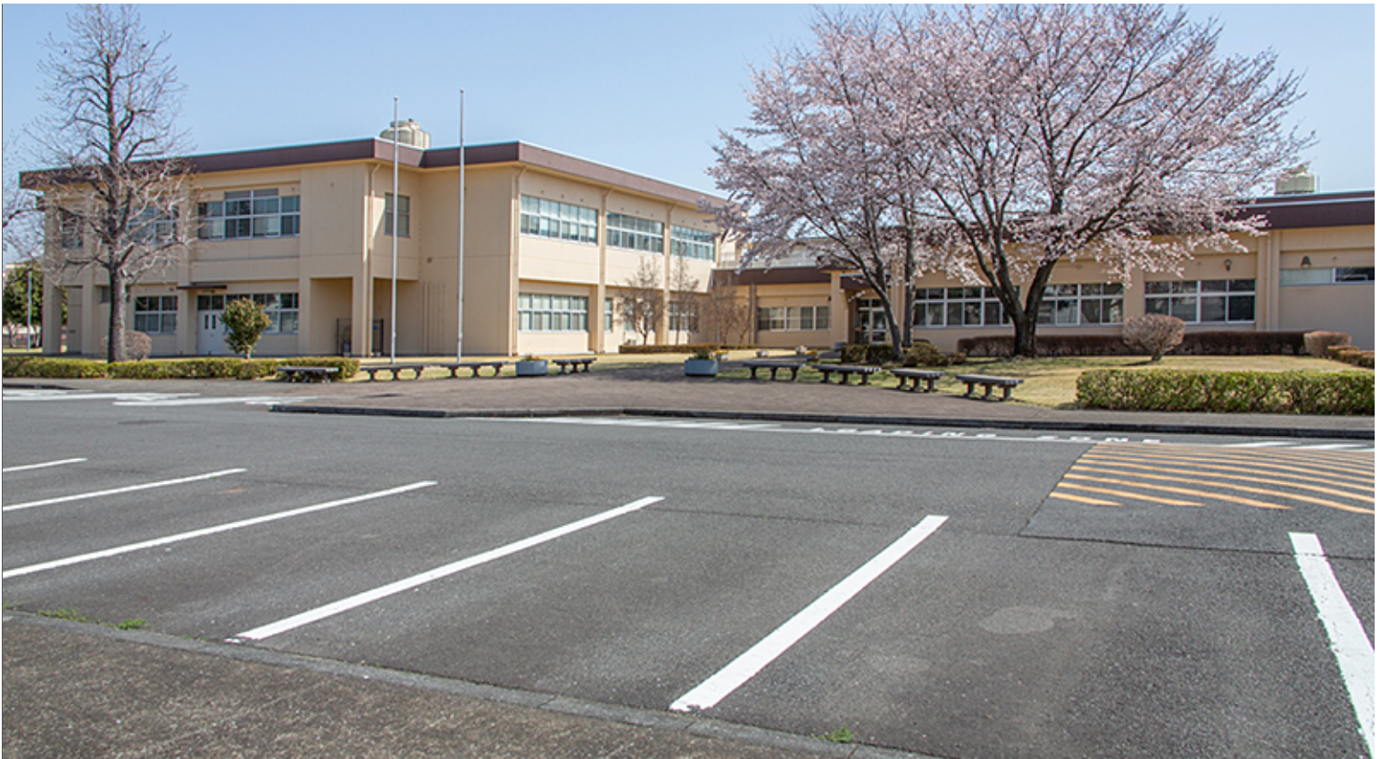
Bituminous Paving and Standard White Striping
