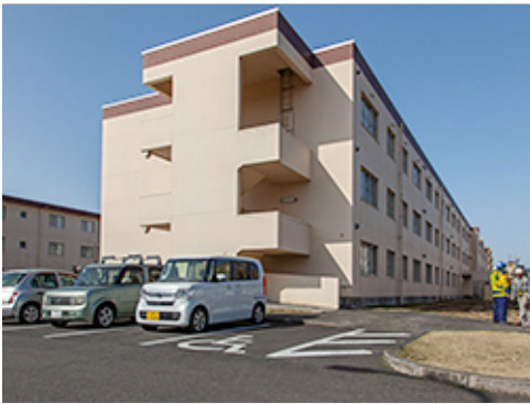
Stairwell Expressed as Element
