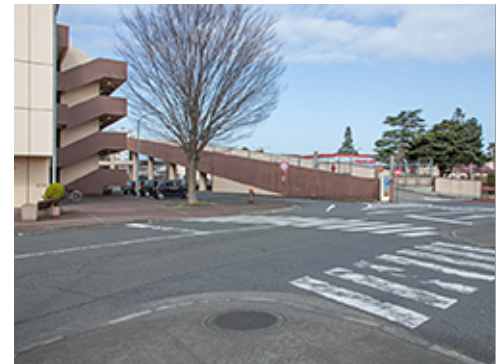
Ramp Access at Street
