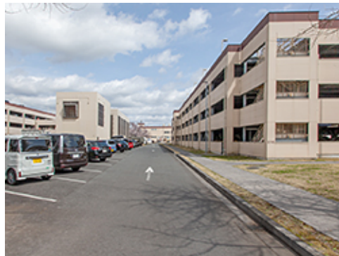
Controlled Access at Garage
