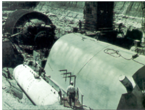
Minuteman-II Launch Control Facility
