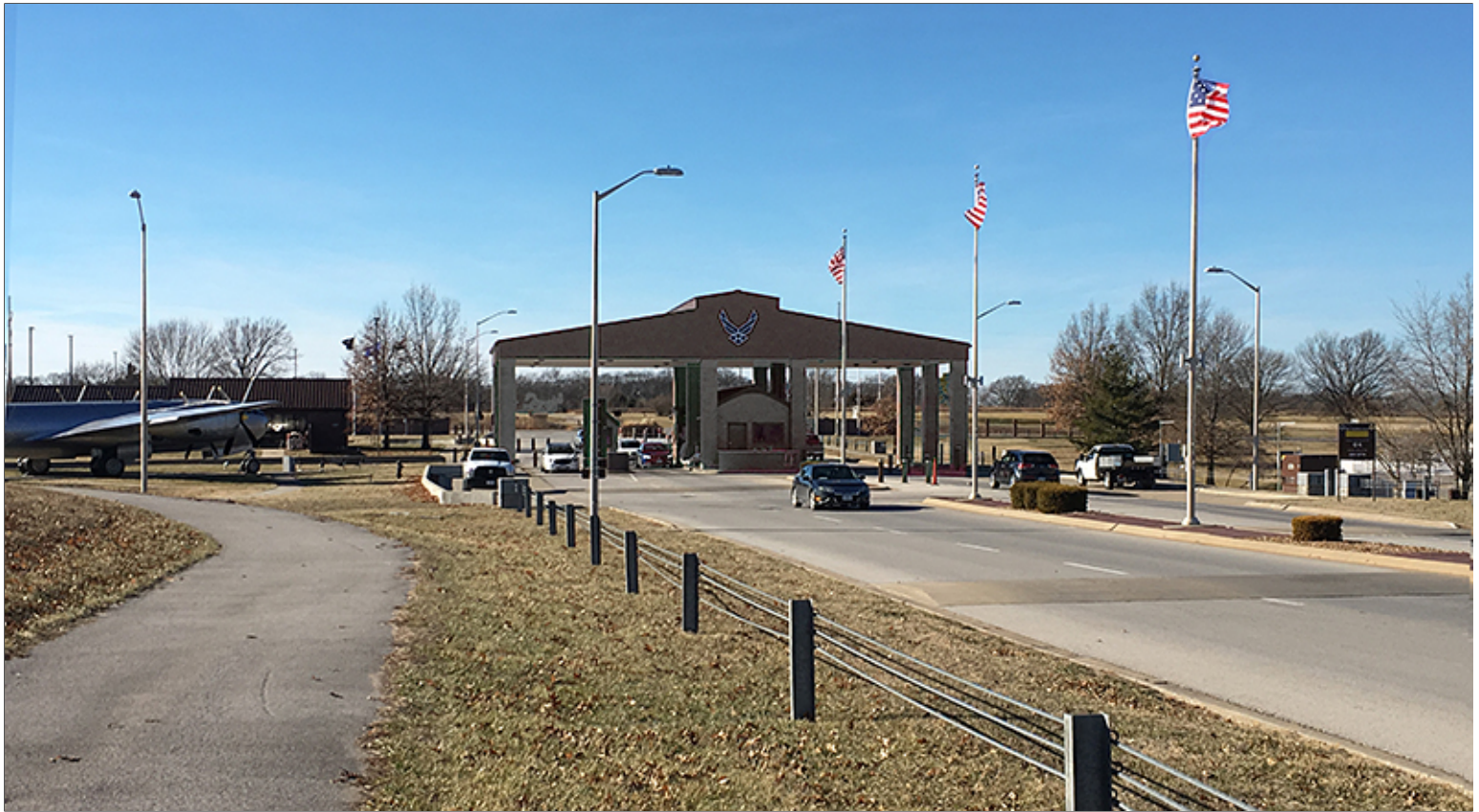
Installation Elements: Streetscape at Main Gate
