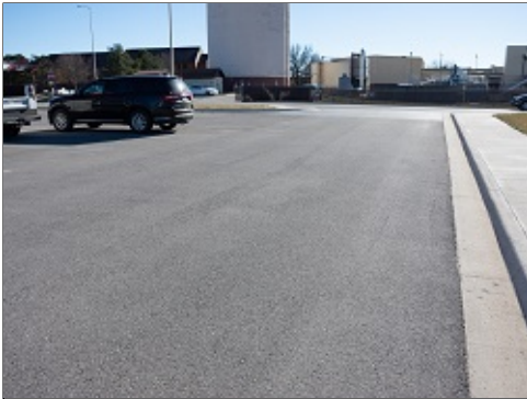
Bituminous Concrete Paving
