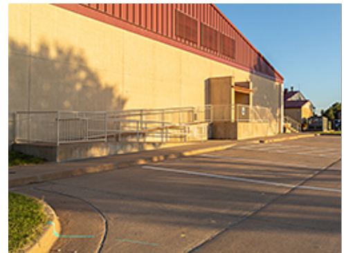
Ramp and Stairs at Group 3
