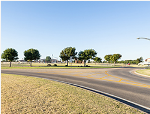
Traffic Circle with Landscaping
