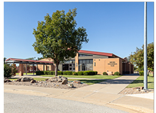
Concrete Paving Adjacent to Group 2
