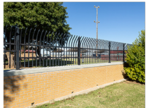
Perimeter Fence near Group 2
