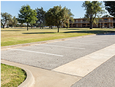
Bituminous Paving and Concrete Pan
