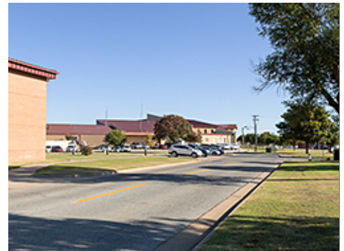
Curb & Gutter with Landscape
