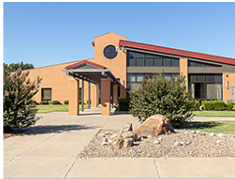
Concrete Entrance Plaza
