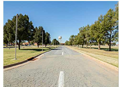
Streetscape at Group 3
