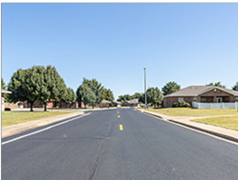
Bituminous Paving with Concrete Sidewalks
