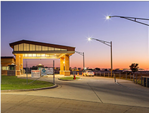
Pole Mounted Fixtures
