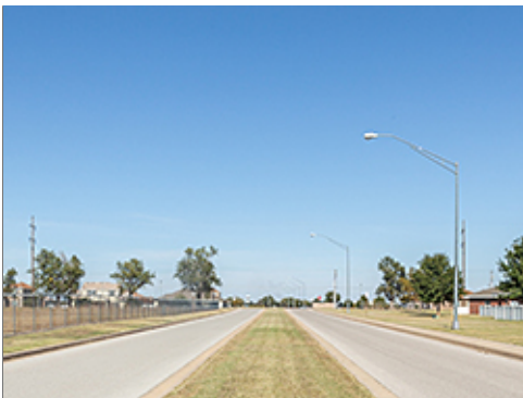
Uniform Street Lighting and Sidewalk Lighting
