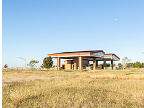
Naturally Forming Grasses near Main Gate
