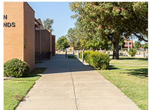
Concrete with Control Joints
