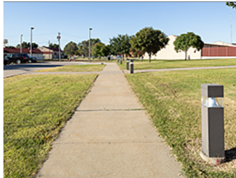
Lighted Bollards Defining Sidewalk
