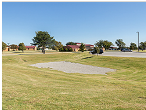
Stormwater Basin with Native Grass Buffer
