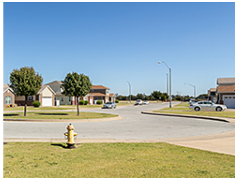
Fire Hydrant and Street Lights in Group 4
