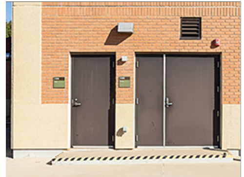
Wall Pack at Service Area
