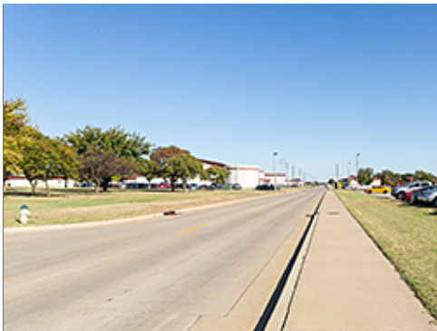
Curb & Gutter with Connected Sidewalk
