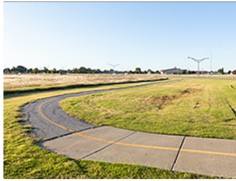
Paving at Trail
