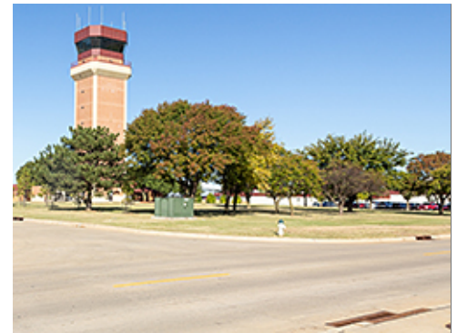
Utility Equipment Adjacent to Group 2
