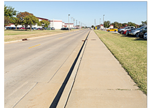
Concrete Barrier Curb and Sidewalk
