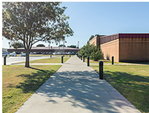
Concrete Sidewalk at Group 2
