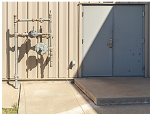
Step / Landing at Group 3 Service Entrance
