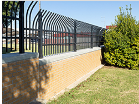
Metal Post and Rail with Masonry
