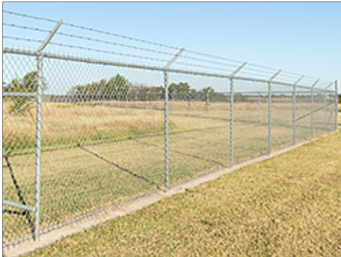
Chain Link Fence near Group 3
