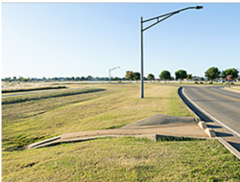
Stormwater Runoff at Street
