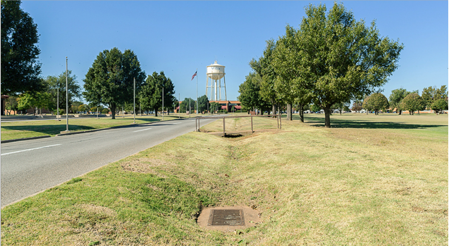
Stormwater Basin with Bridge as Amenity
