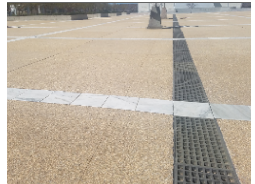
Drain Integrated in Marble Banding
