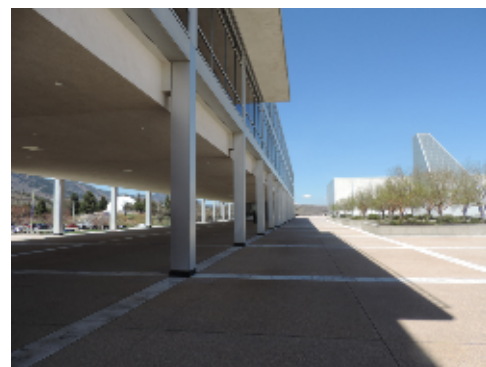
7 Foot Governing Grid in Paving
