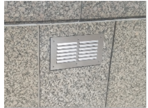
Retaining Wall - Recessed Lighting
