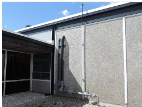
Paint Above Grade Utilities
