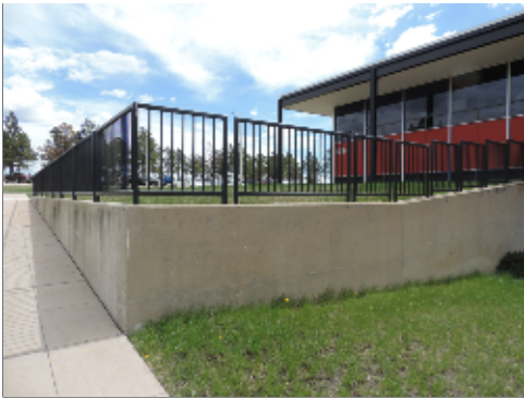
Retaining Wall - Other
