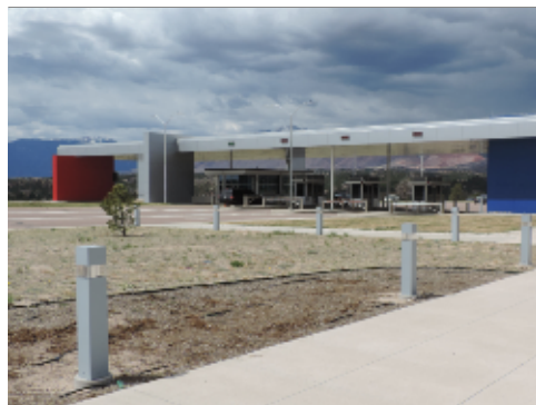
Main Gate - Fencing, Gates
