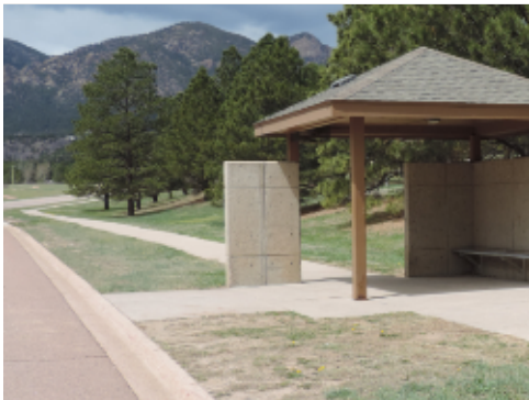
Sidewalk along Roadway
