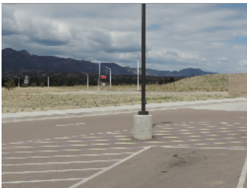
Parking Lot Striping
