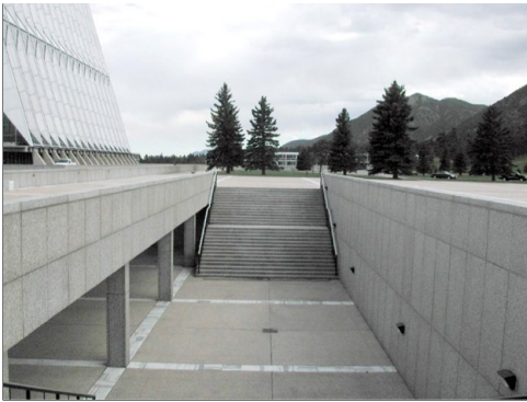
Retaining Wall - Granite
