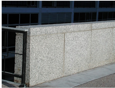
Granite Retaining Wall - Cap and Rail
