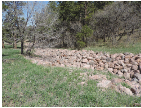
Water Quality Facility
