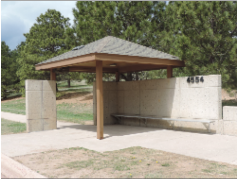
Public Transportation - Shelter
