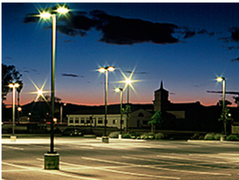
Parking Lot Lighting
