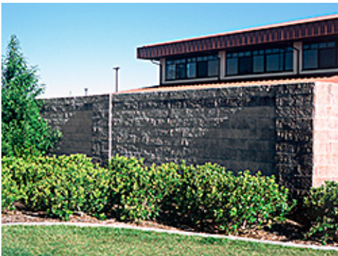
Accent Planting at Masonry Screen Wall
