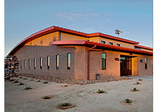
Pervious Paving Used at Fire Station
