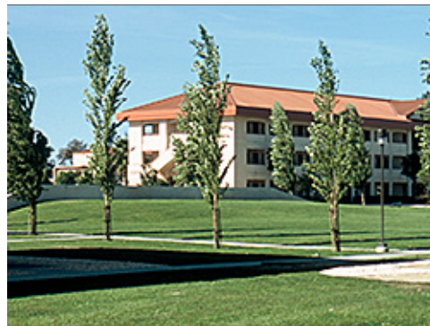
Trees and Integrated Lighting
