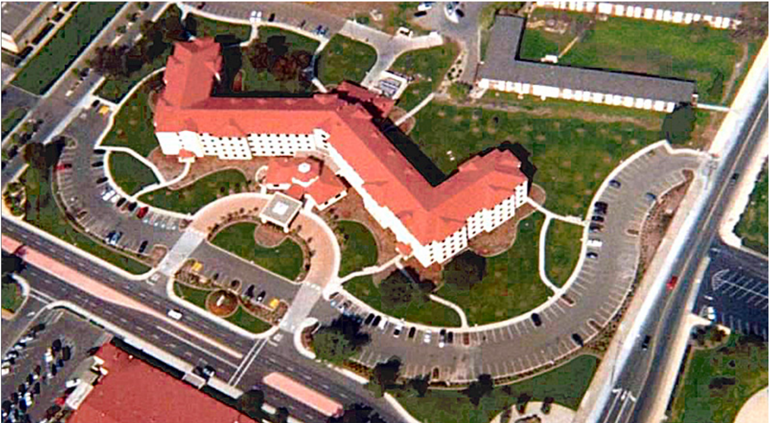
Westwind Inn Base Lodging with Clearly Defined Pedestrian and Vehicular Circulation
