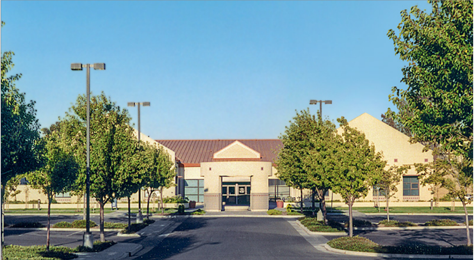
Primary Parking Access Drive Aligning with Building Entrance Feature
