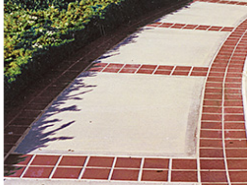
Combination of Concrete and Brick Pavers
