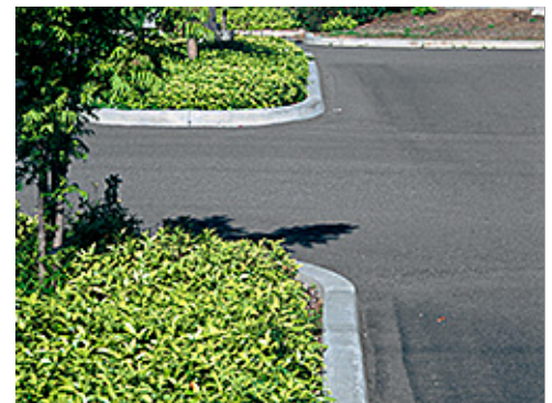
Header Curb at Island
