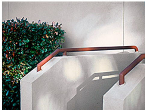
Stair Wall and Railing
