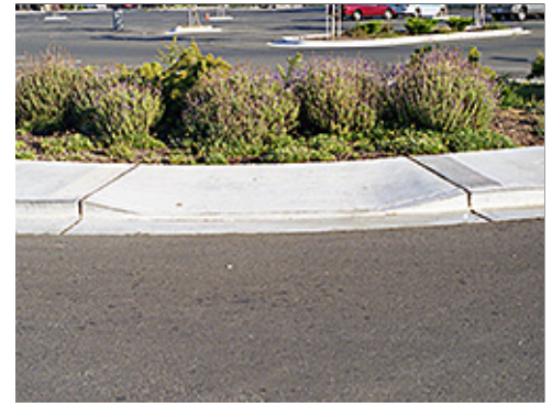
Accent Planting at Curb Cut
