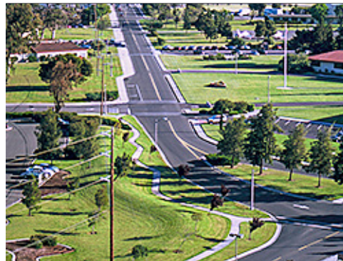
Travis Avenue from Main Gate
