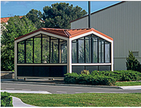
Accent Planting at Bus Shelter
