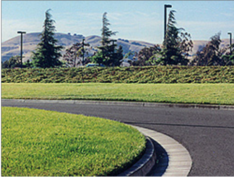
Typical Bituminous Paving with Concrete Curb
