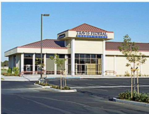
Asphaltic Concrete Paving
